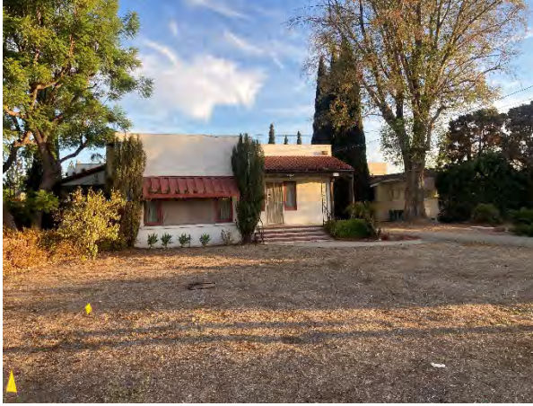
1. View of 2101 E Santa Clara Ave, southwest to north
