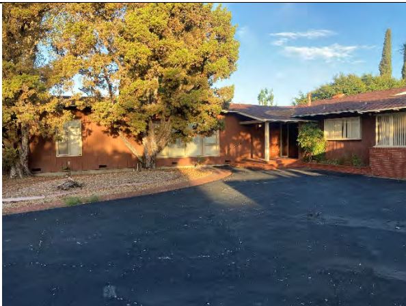
5. View of 2109 E Santa Clara Ave, east to west
