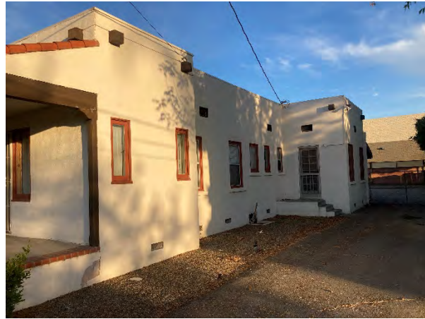
2. View of 2101 E Santa Clara Ave, south to northwest
