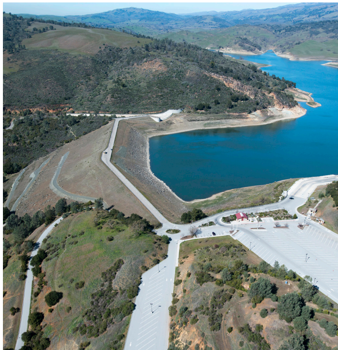
Aerial view of Anderson Dam
