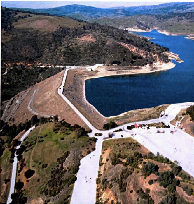
Aerial view of Anderson Dam
