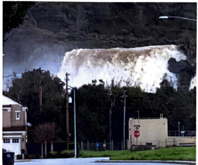
Anderson Dam spillway flow cascades into Coyote Creek behind neighborhood
