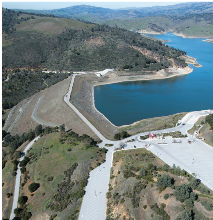
Aerial view of Anderson Dam
