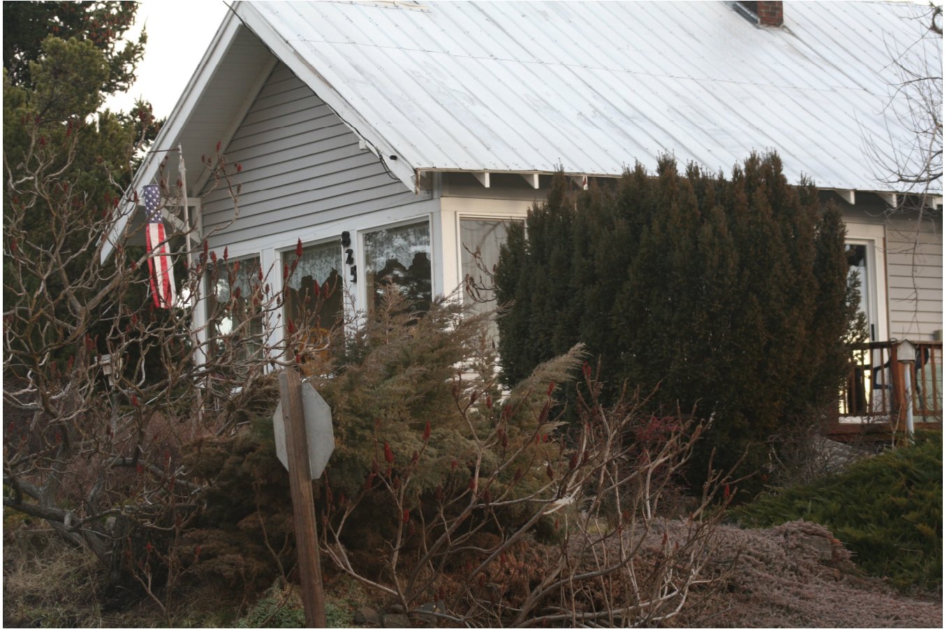
Home with insufficient defensible space
