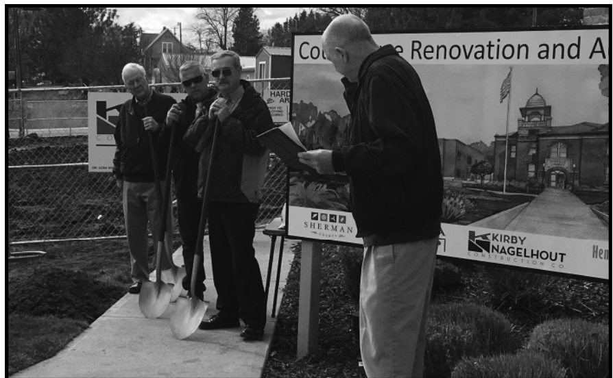
Pictured: Commissioners McCoy and Dabulskis and Judge Thompson prepare to officially break ground after an introduction provided by Justice of the Peace Ron McDermid.
