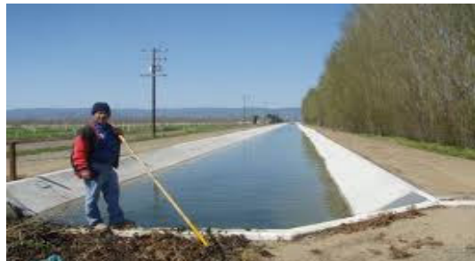
SID Concrete Lined Canal
