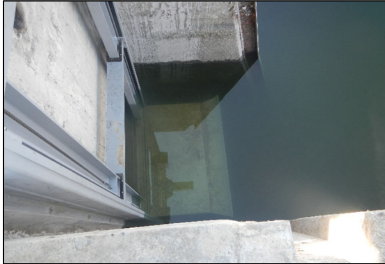
Vaughn Canal Headworks metering
