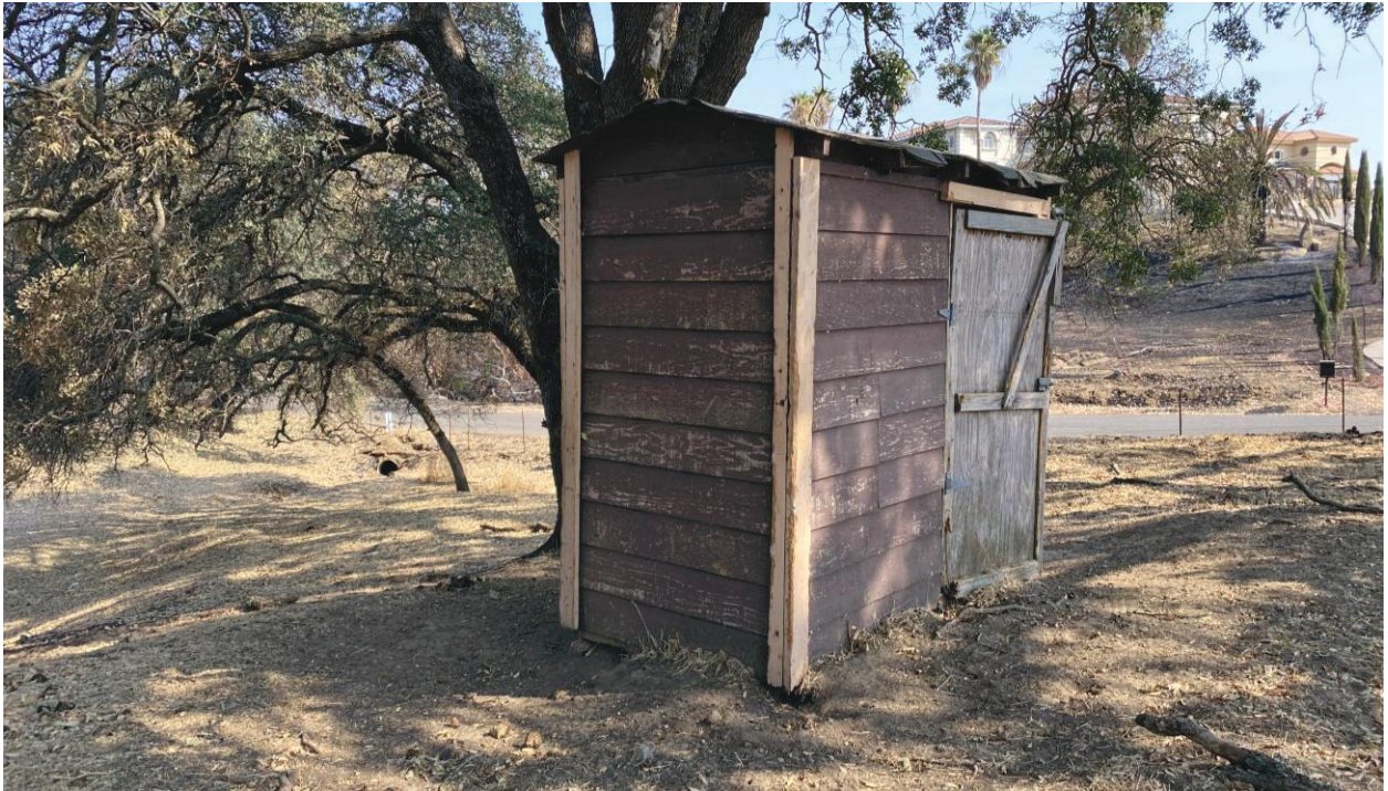
Photo 5. SAS-001 - view to Northeast
