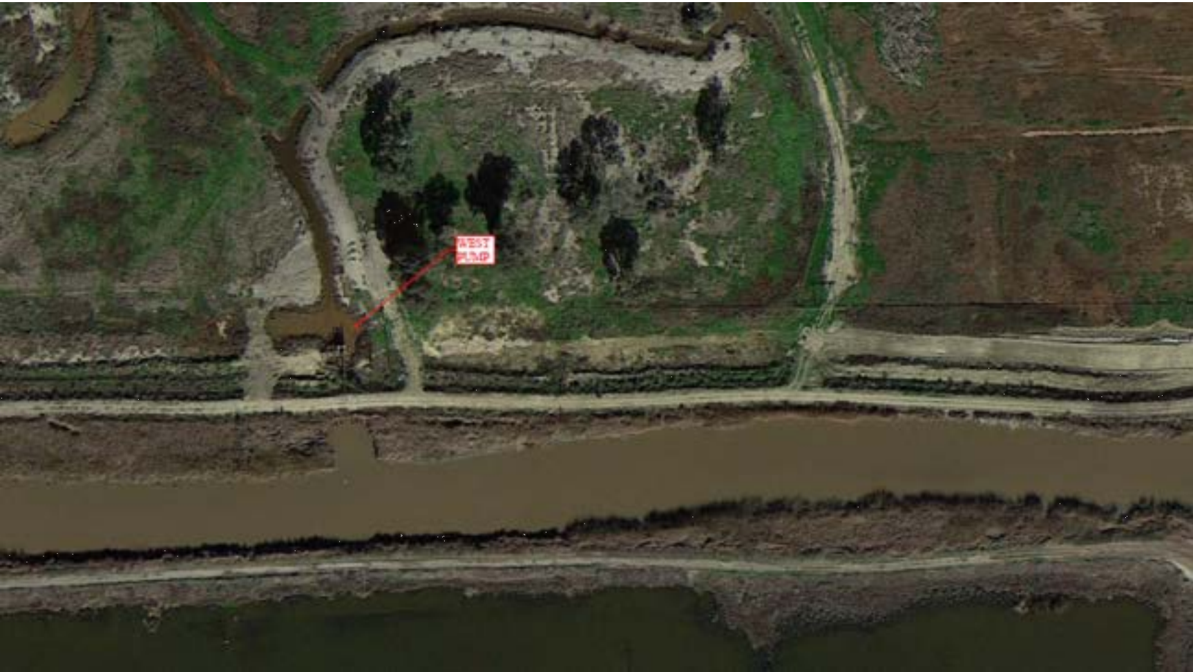
Figure A4: Location of West Pump
