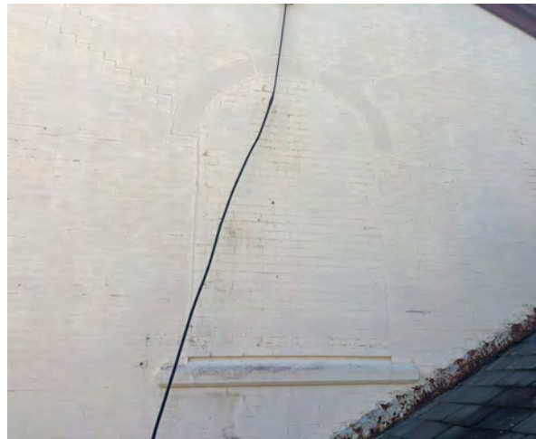
Photo 78: Outline of filled-in arched window above main staircase of Borough Hall.
