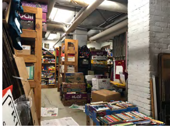
Photo 51: View southeast in Room 013 showing brick columns and exhaust fan on east wall.
