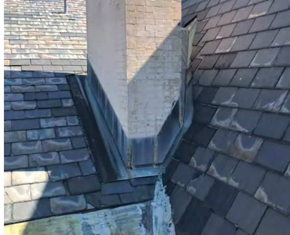
Photo 7: Copper flashing around chimney at south elevation.
