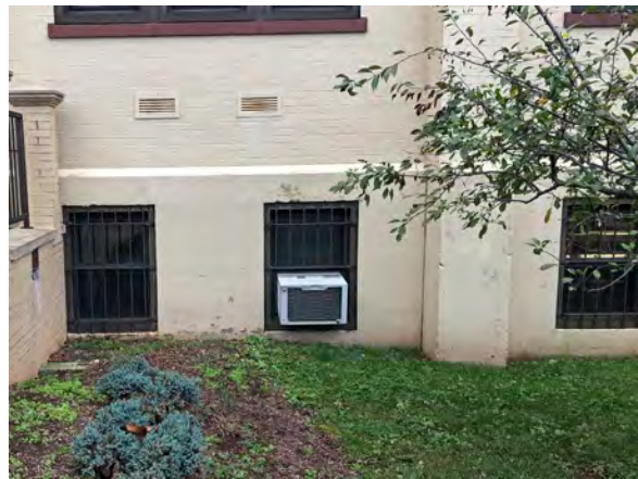
Photo 76: Typical basement windows at north elevation of Library.
