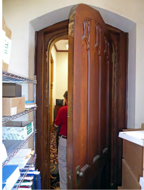
Photo 133: Door connecting to Room 103.
