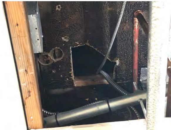
Photo 74: Gypsum wall board chase behind ceiling. Cut to allow conduit installation.
