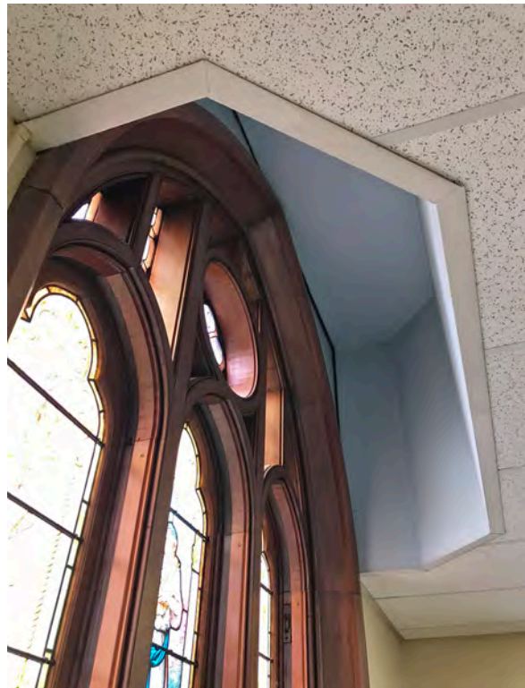
Photo 226: Top of arched window above dropped ceiling.
