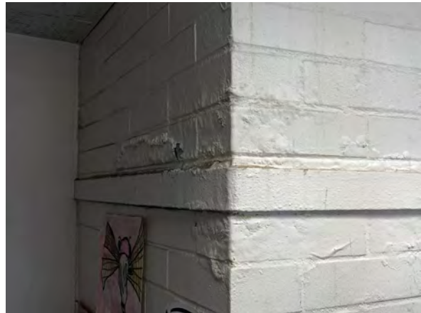
Photo 256: Chimney on east wall in Room 213.
