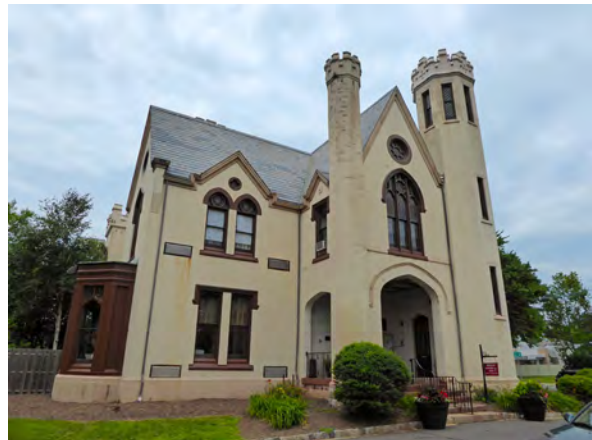
Photo 28: East elevation of Borough Hall, viewed from the south.
