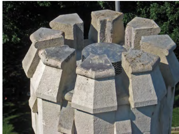
Photo 38: Positive slope and vented cap installed on south tower roof in 2008.
