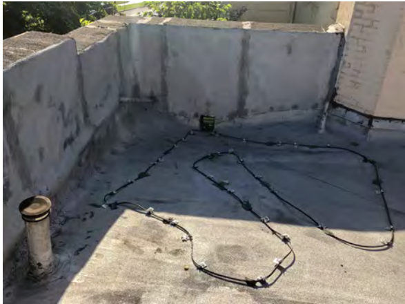
Photo 17: Roof of Library Addition with drain opening in its east parapet.
