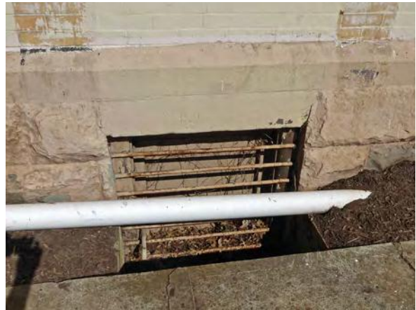
Photo 52: Foundation window (E001) at north side of east elevation.
