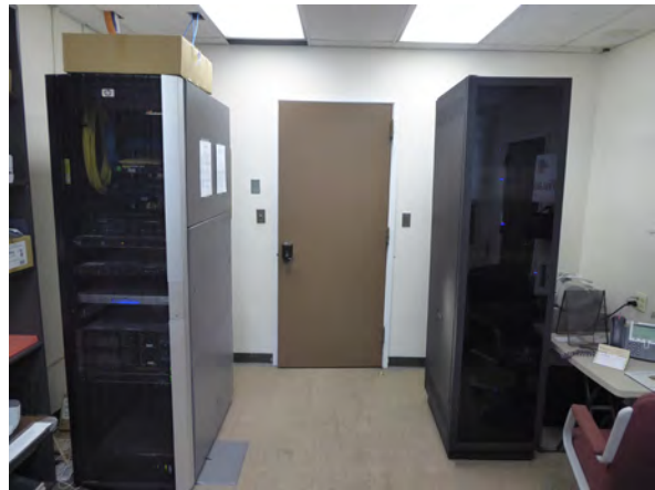
Photo 153: View north in Room 108.
