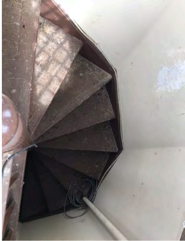
Photo 266: Spiral stair in top room of northeast stair tower.
