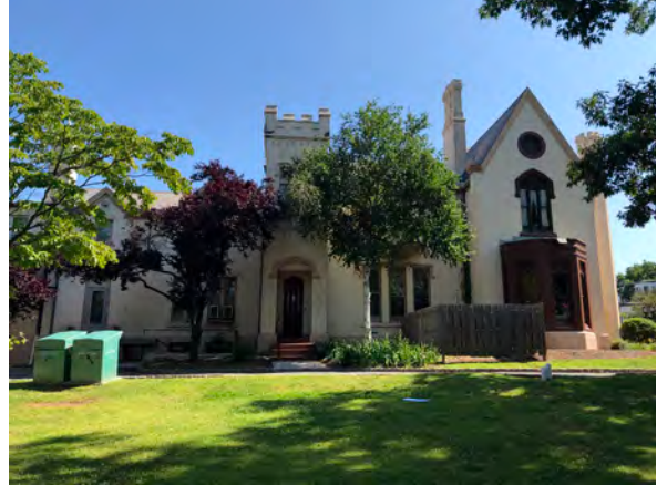
Photo 80: South elevation of Borough Hall.
