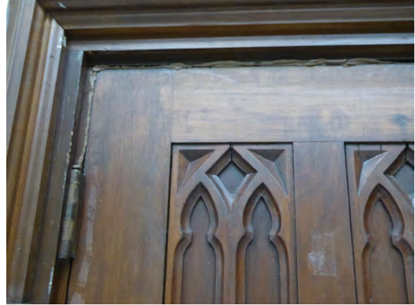
Photo 165: Sealant on top of door connecting to Room 113.
