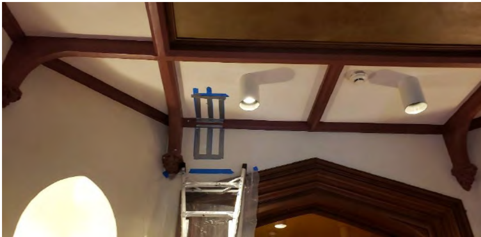
Figure 13. Preparation for exposure windows in Room 100.
