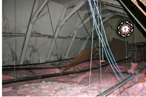
Photo 229: Vaulted ceiling concealed behind dropped ceiling in Room 207.
