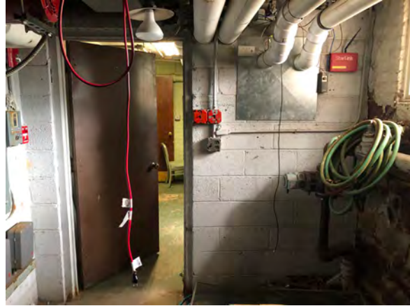
Photo 46: View east in Room 012.
