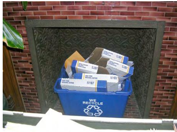
Photo 211: Decorative cast iron firebox insert at fireplace in Room 203.
