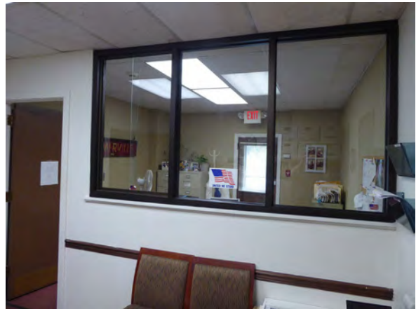
Photo 159: Dividing wall and door between Rooms 109 & 110.
