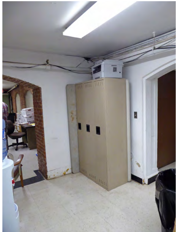
Photo 24: View west in Room 006 showing archway connecting to Room 001.
