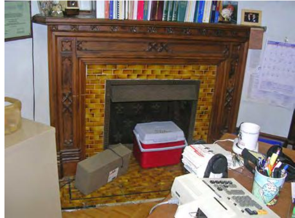
Photo 169: Fireplace in northwest corner of Room 112.
