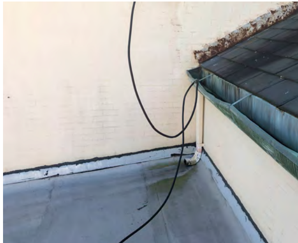
Photo 20: Downspout from Borough Hall roof empties onto Library Addition roof.
