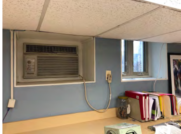
Photo 10: Windows on south wall in Room 002.
