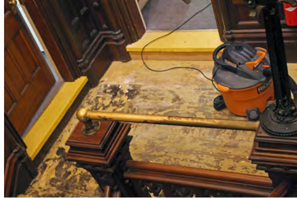
Photo 107: Wood floor of landing exposed during carpet installation in 2014.
