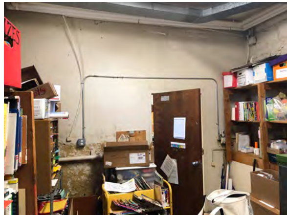
Photo 58: View north in Room 014 showing door to Room 015.
