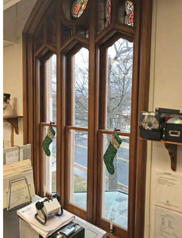
Photo 234: Arched window opening on north wall in Room 207.
