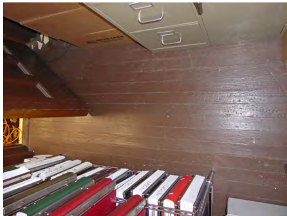
Photo 132: Painted wood floor.
