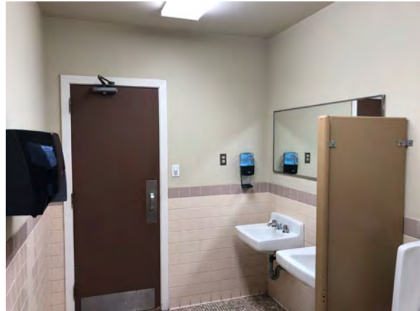
Photo 246: View north in Room 210.
