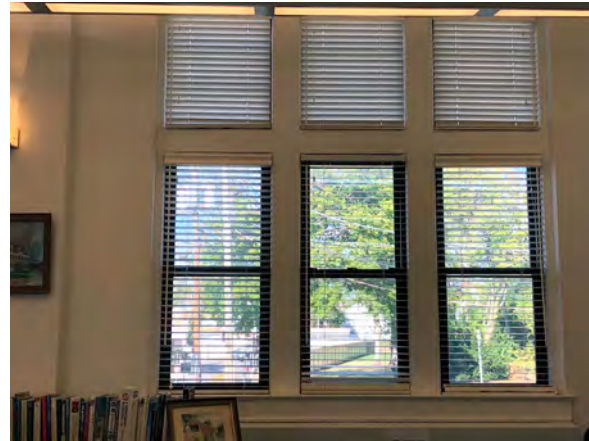
Photo 190: Typical windows in Room 115.
