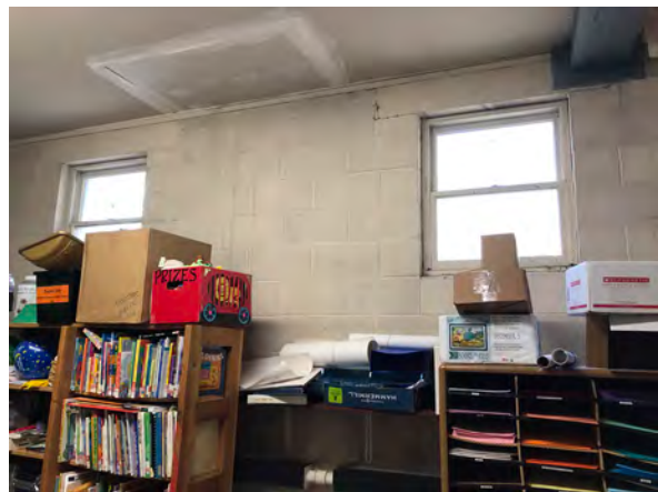
Photo 61: View west in Room 015, showing windows and cut out section of ceiling.
