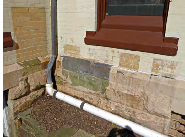
Photo 30: Finish removal tests at north side of east elevation.
