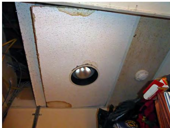
Photo 185: Dropped ceiling in closet of Room 114.
