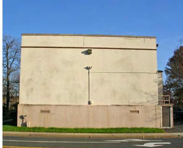
Photo 77: West elevation of Library.
