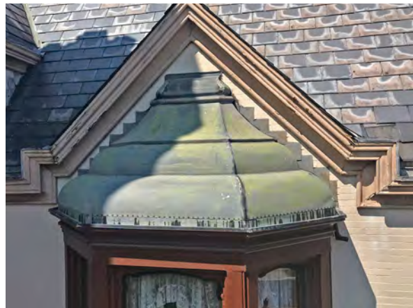
Photo 56: Copper roof on oriel window.
