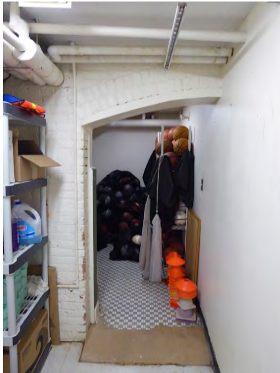
Photo 18: View south in Room 005, showing brick foundation dividing the room.
