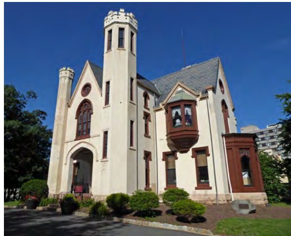
Photo 29: East elevation of Borough Hall, viewed from the north.
