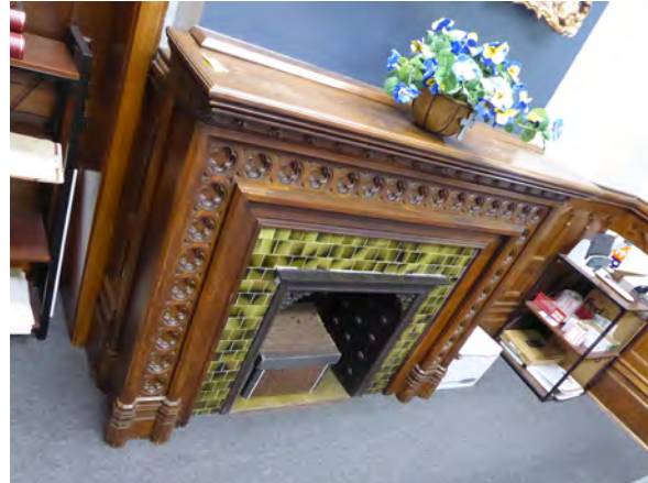
Photo 143: Fireplace on the east wall in Room 104.
