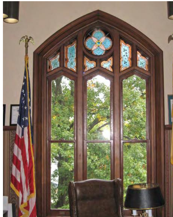
Photo 213: Windows on south wall in Room 204.
