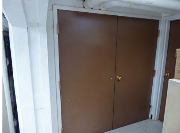
Photo 23: Double doors to closet in Room 006.
