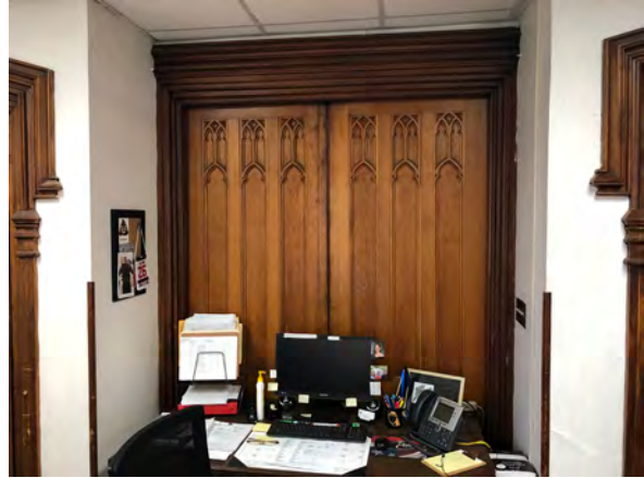
Photo 224: Pocket doors on west wall in Room 205.
