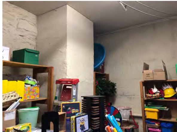
Photo 60: Chimney foundation on east wall in Room 014.
