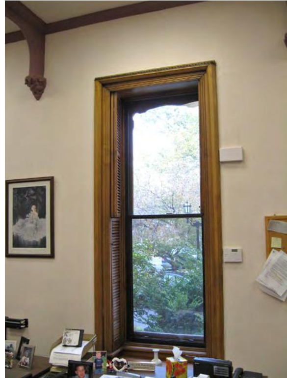
Photo 123: Window and interior shutters on east wall in Room 103.
