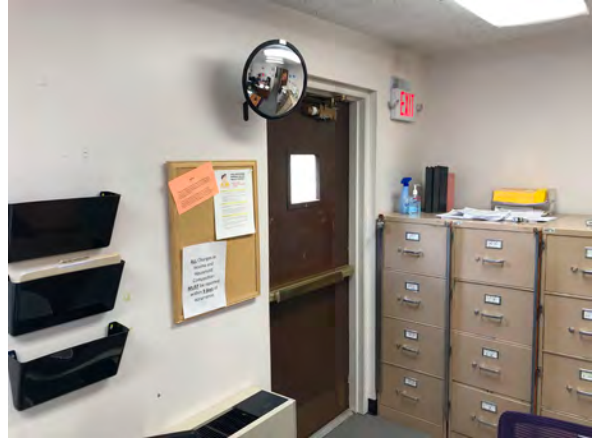
Photo 255: Exit door on west wall in Room 213.
