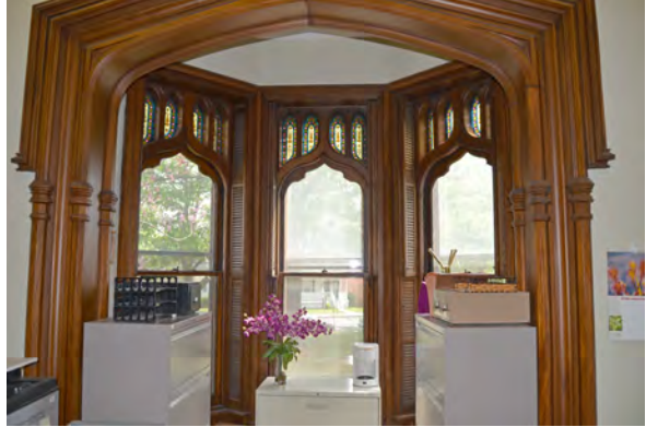
Photo 115: Windows in canted bay on south wall in Room 102.
