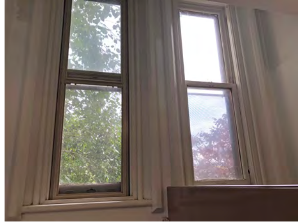
Photo 204: Windows on south wall in Room 202.
