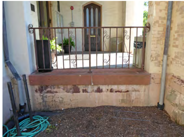
Photo 46: Wrought iron railing on south side of entry porch.
