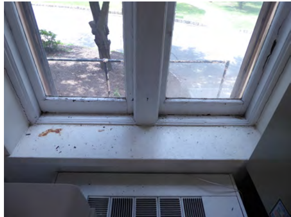
Photo 156: West pair of windows in Room 108.
