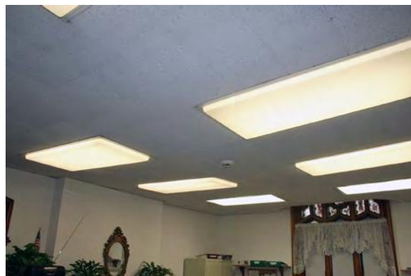
Photo 231: Dropped ceiling in Room 207.
