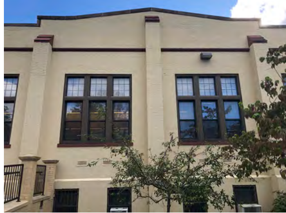
Photo 75: Typical first floor windows at north elevation of Library.
