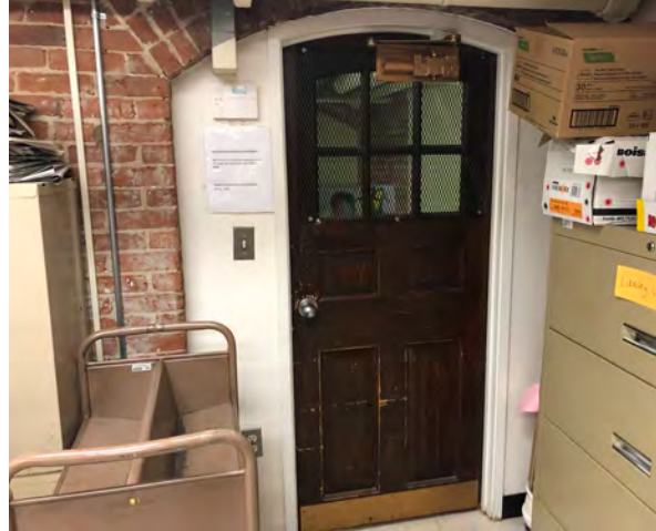
Photo 36: Door on the south wall connecting to Room 001.
