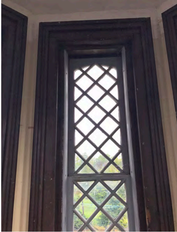
Photo 268: Typical wood window in northeast stair tower.
