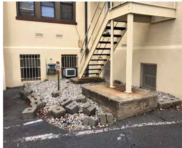
Photo 99: Base of fire escape stairway on rear addition of Borough Hall.
