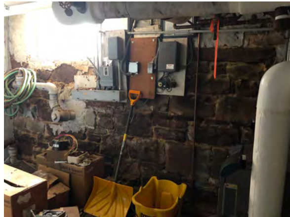
Photo 47: South foundation wall in Room 012.
