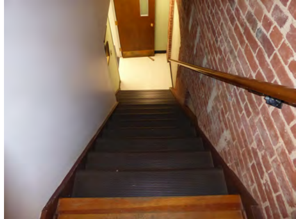
Photo 5: View of basement stairs from top landing.
