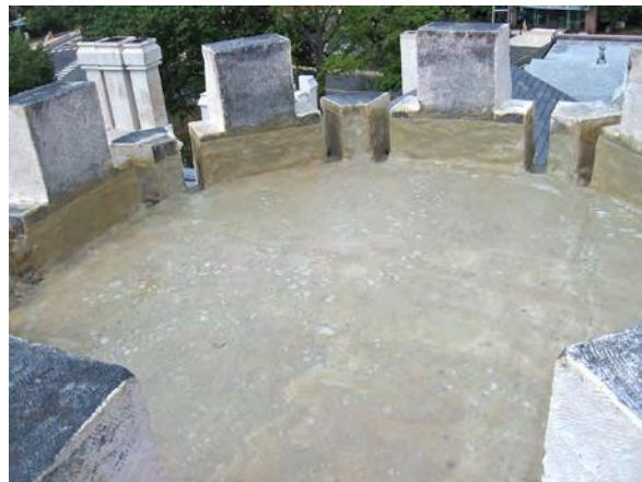
Photo 39: New membrane roof on north tower of east elevation installed in 2010.
