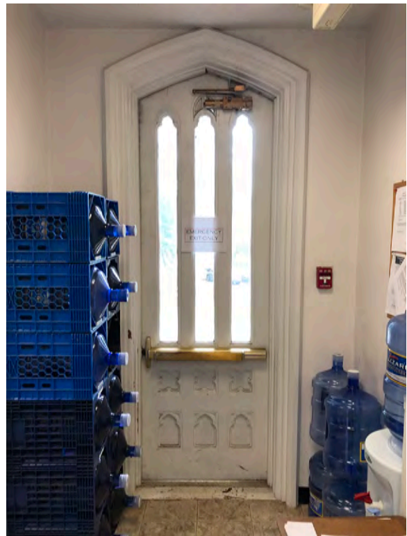
Photo 149: Exterior door on south wall in Room 105.
