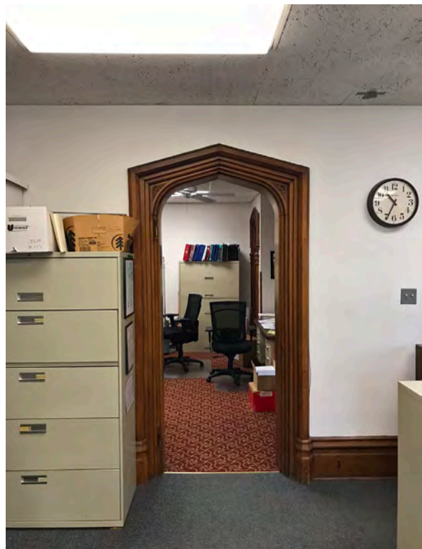
Photo 233: Door into Room 205 on south wall.
