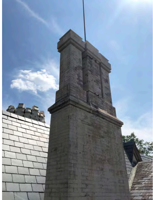
Photo 22: South chimney of Borough Hall.
