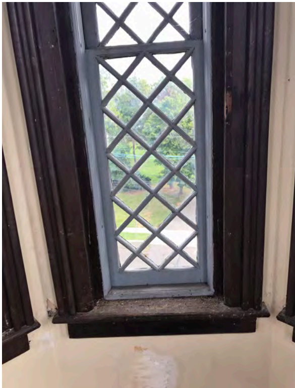
Photo 269: Typical wood window in northeast stair tower.
