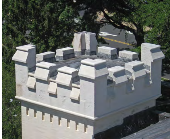
Photo 83: Sloped membrane roof on south tower.
