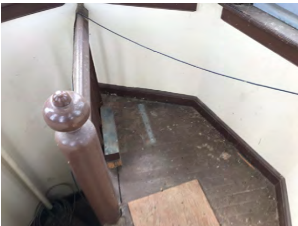
Photo 265: Landing in top room in northeast stair tower.
