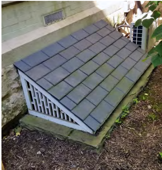
Photo 62: Cover over foundation window on north elevation.
