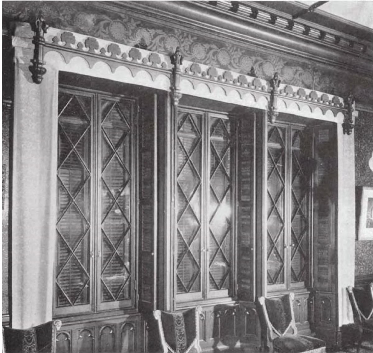
Figure 34: The dining room of the Harral House. While the windows are different, the wainscot appears to be an exact match.
