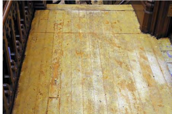
Photo 199: Wood floor exposed during carpet installation in 2014.
