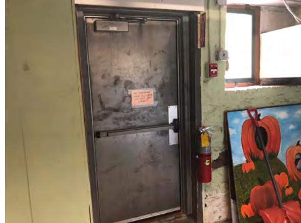
Photo 43: Exterior door on south wall in Room 011.
