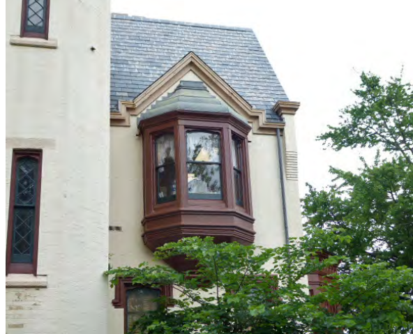
Photo 54: Second-floor oriel window on north side of east elevation.
