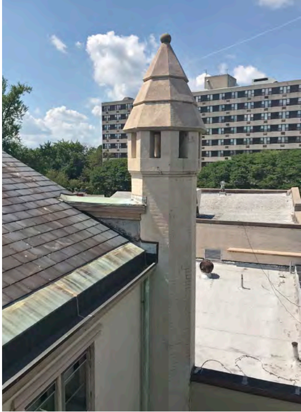
Photo 24: Northwest chimney of Borough Hall.
