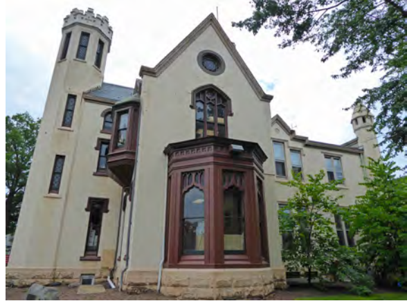
Photo 59: East end of north elevation of Borough Hall.
