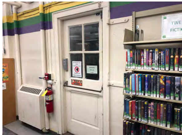
Photo 66: Exterior door on south wall in Room 015.
