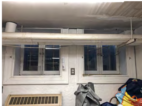
Photo 38: Double casement windows on the north wall.
