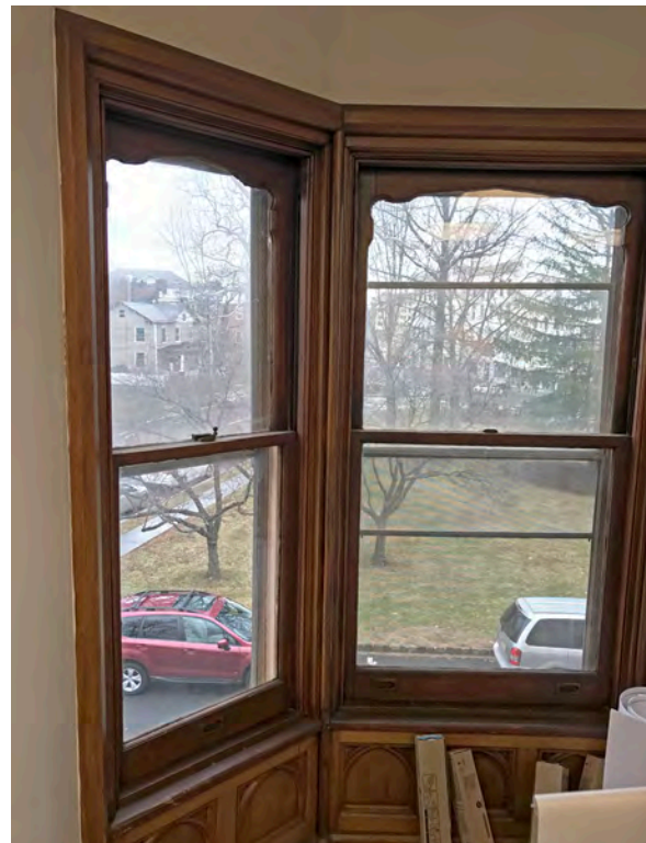
Photo 235: Windows on canted bay area on east wall in Room 207.
