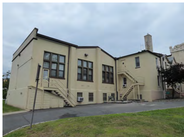
Photo 82: Library and rear addition of Borough Hall. Both fire escape stairways shown in photo.
