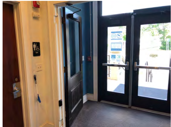
Photo 193: View of entrance vestibule on north side of Room 116.
