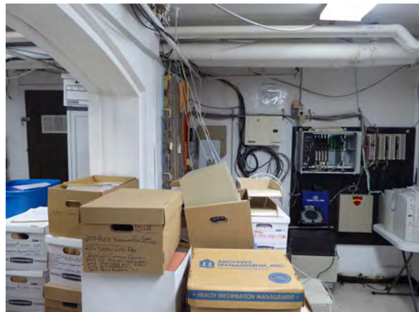
Photo 22: View east in Room 006.
