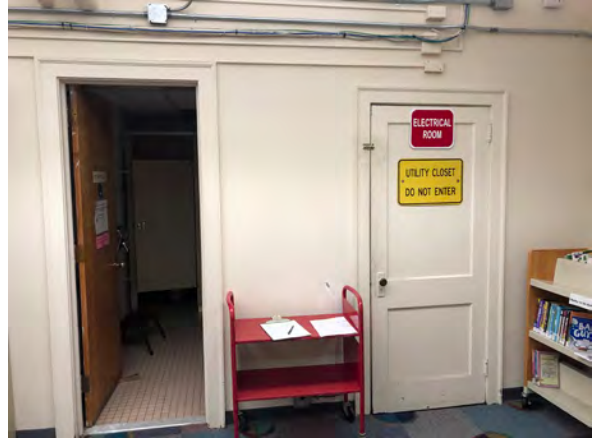
Photo 82: View of doorways into Rooms 019 & 020 from Room 015.
