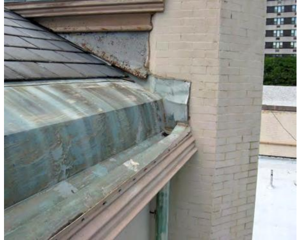
Photo 13: Typical view of built-in gutter at cornices of Borough Hall.
