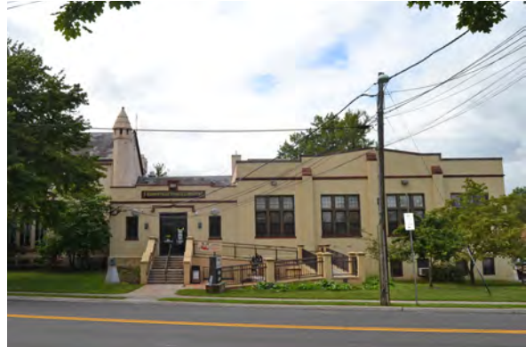
Photo 67: View of Library and entrance stairs and ramp from across street.
