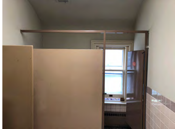
Photo 245: View south in Room 210.
