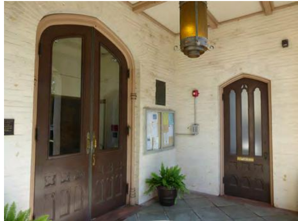
Photo 57: Main entry double doors and side tower door at entry porch.
