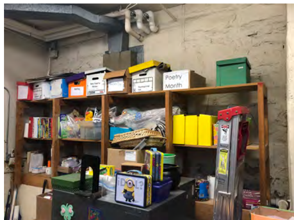
Photo 59: Exposed stone foundation of Borough Hall on east wall of Room 014.
