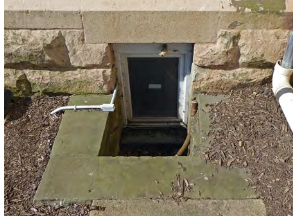
Photo 51: Foundation window (N001) at north wall of north tower.
