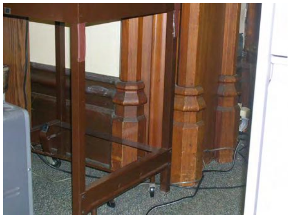
Photo 117: Baseboard and base of trim around south archway in Room 102.
