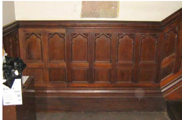
Photo 105: Typical wainscot in Room 101 and along staircase.
