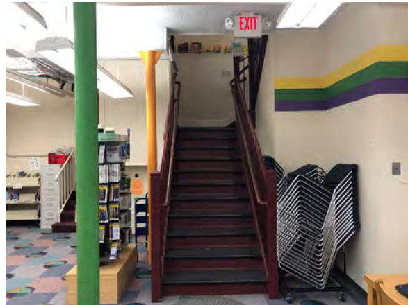
Photo 68: Stair to first floor at east end of Room 015.
