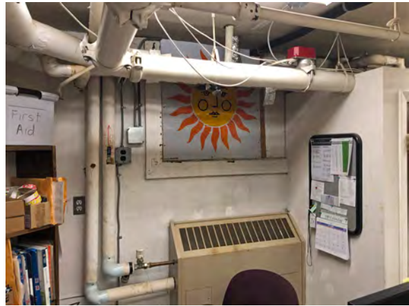
Photo 37: Covered up window opening on the north wall.
