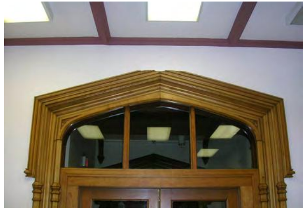
Photo 121: White maple trim around archway on south wall connecting to Room 100.
