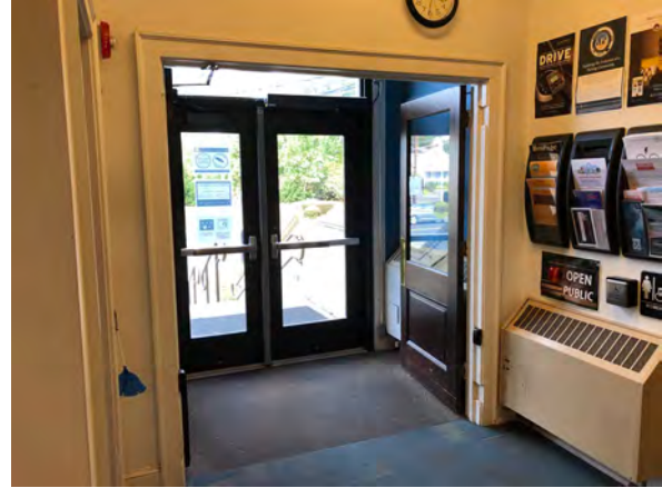
Photo 192: View of entrance vestibule on north side of Room 116.
