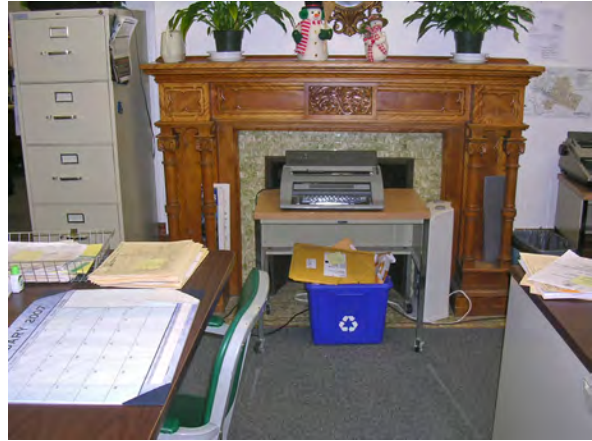
Photo 236: Fireplace on west wall in Room 207.
