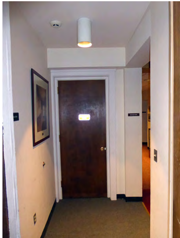
Photo 183: View west in Room 114 showing closet.
