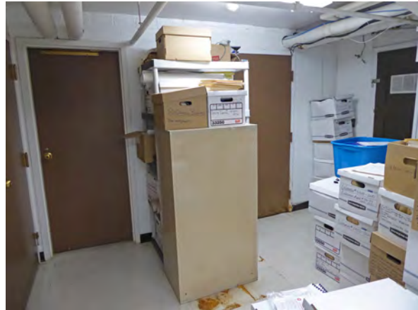
Photo 21: View north in Room 006 showing doors to Rooms 007 & 008 and to tower.
