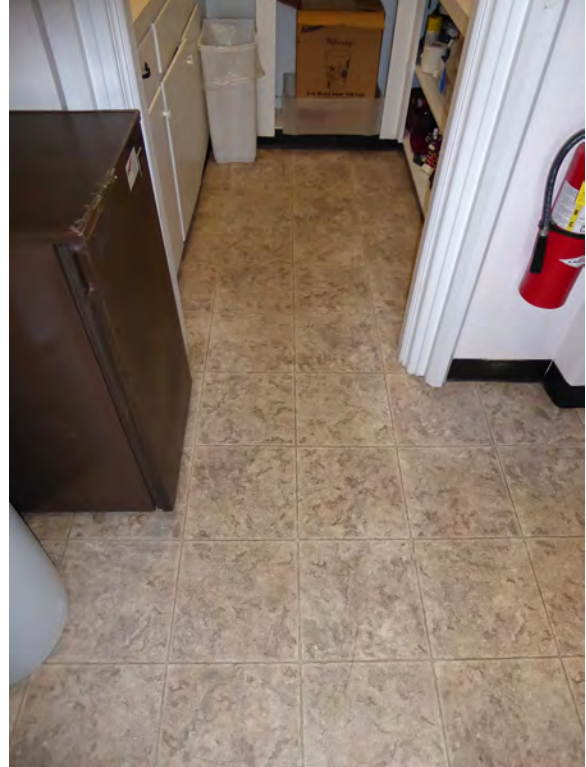
Photo 148: View of floor showing doorway separating Rooms 105 & 106.
