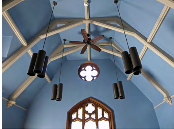
Photo 214: Vaulted ceiling with painted wood framing in Room 204..
