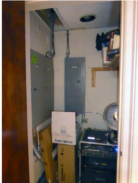
Photo 184: View inside closet of Room 114.
