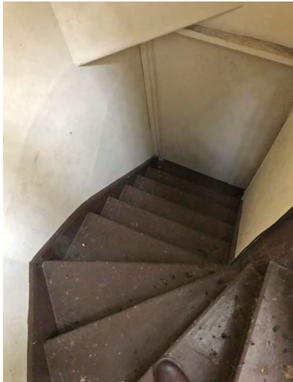
Photo 267: Spiral stair to door in top room of northeast stair tower.
