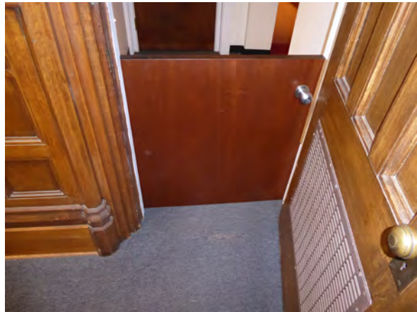
Photo 139: Doorway into Room 115 with half door and showing ventilation panel on historic door.
