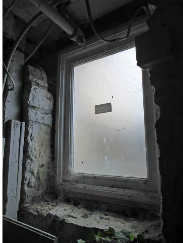
Photo 32: Window on north side of Room OST-2.
