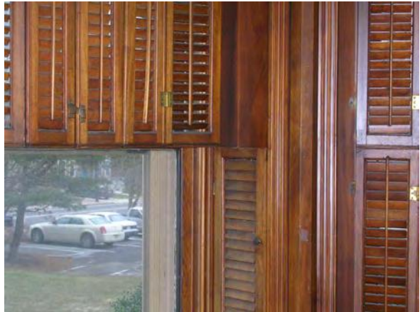
Photo 116: Interior shutters on south windows in Room 102.
