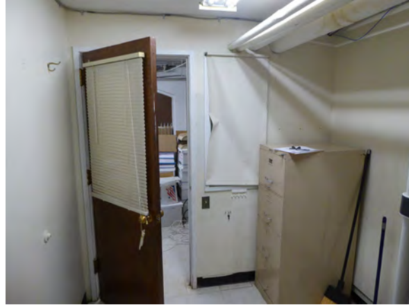
Photo 17: View north in Room 005.
