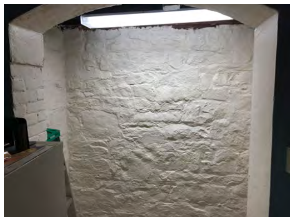
Photo 12: Painted exposed masonry foundation in closet of Room 002.
