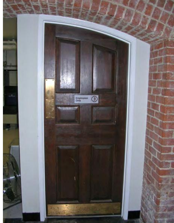
Photo 16: Wood door into Room 004. Photo taken in 2007.
