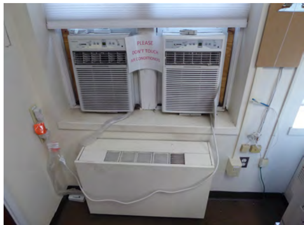
Photo 157: East pair of windows in Room 108 with air conditioning units.
