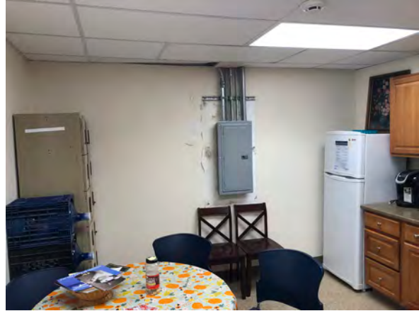
Photo 75: View north in Room 018.
