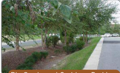
Bio Swale and Curbless Parking
