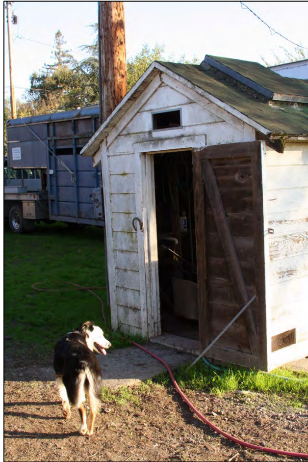
Figure 60: Well house, north elevation
