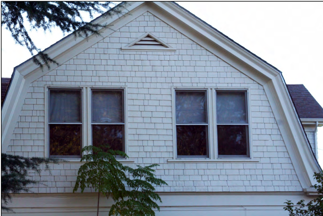
Figure 24: East elevation, second story windows
