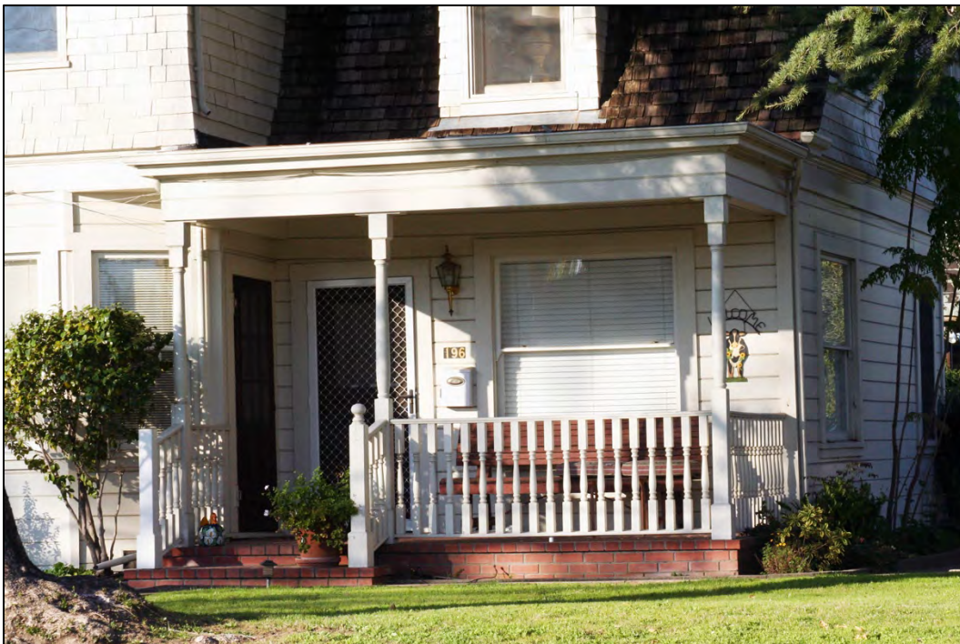
Figure 2: South facade, porch at southeast corner
