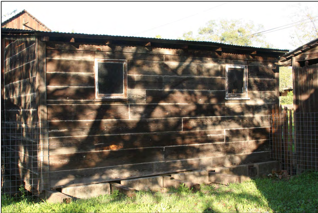
Figure 57: Outbuilding relocated from high school, south elevation
