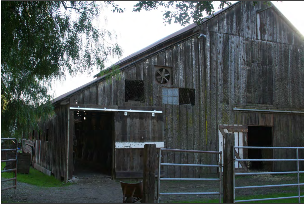
Figure 45: Horse barn, northeast corner
