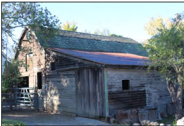
North and east elevations (northeast corner), shed addition on north
