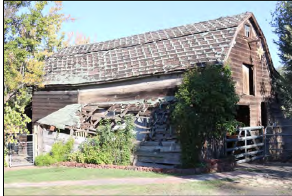
South Elevation (southeast corner)
