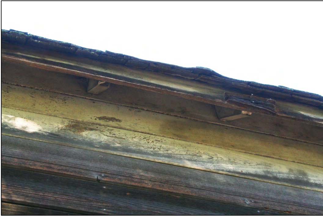
Figure 31: Dairy barn, exposed rafter ends
