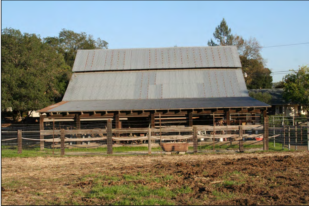
Figure 49: Horse barn, west elevation
