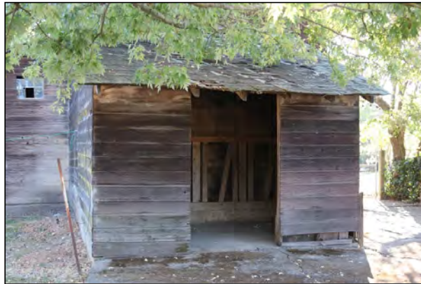
West elevation, shed addition
