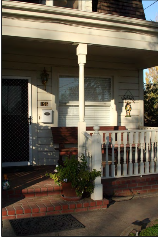
Figure 3: South facade, porch detail
