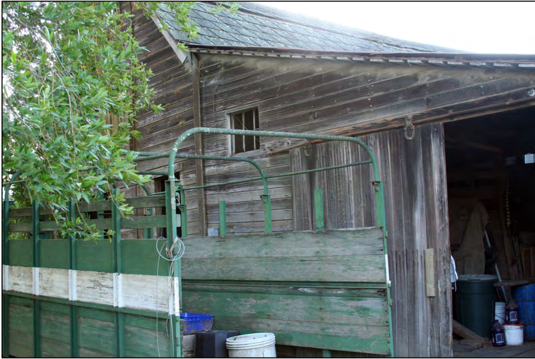
Figure 33: Dairy barn, east elevation of north wing
