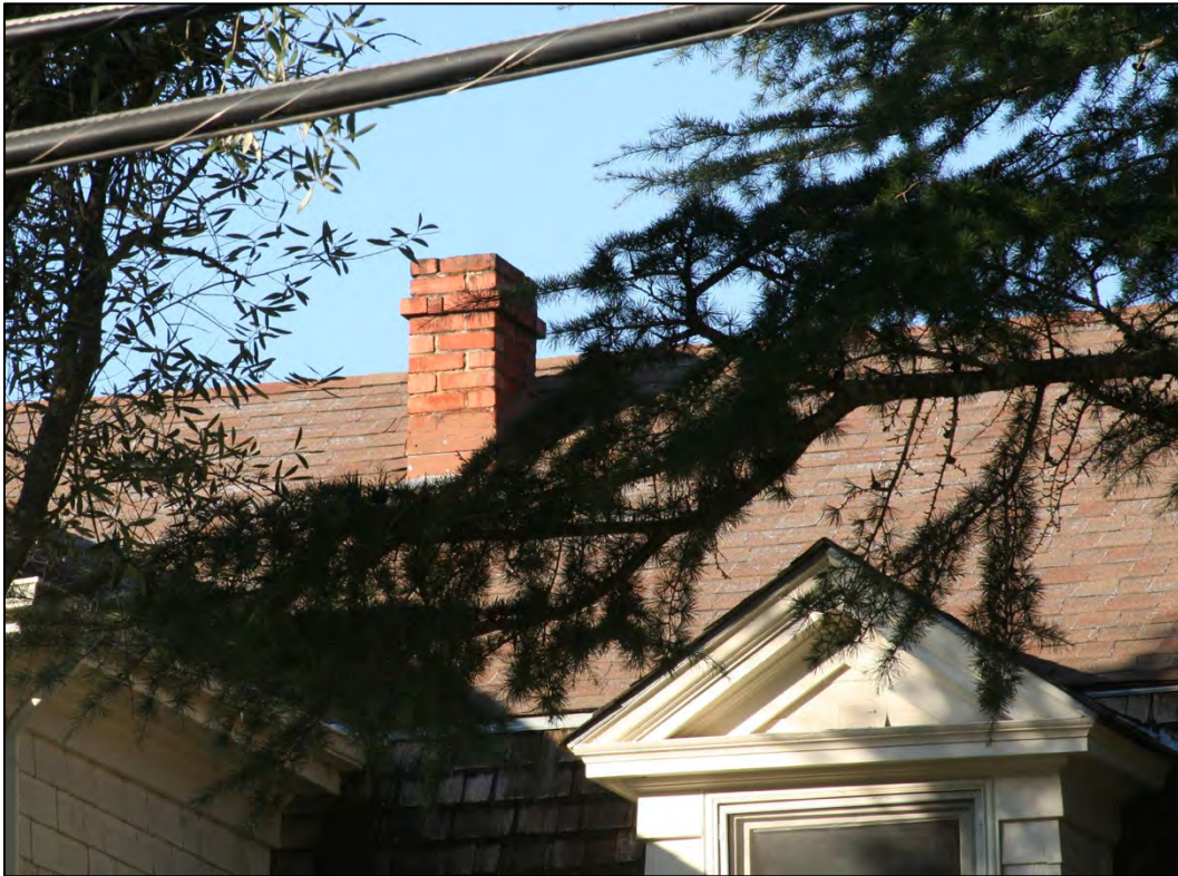
Figure 9: South facade, brick chimney
