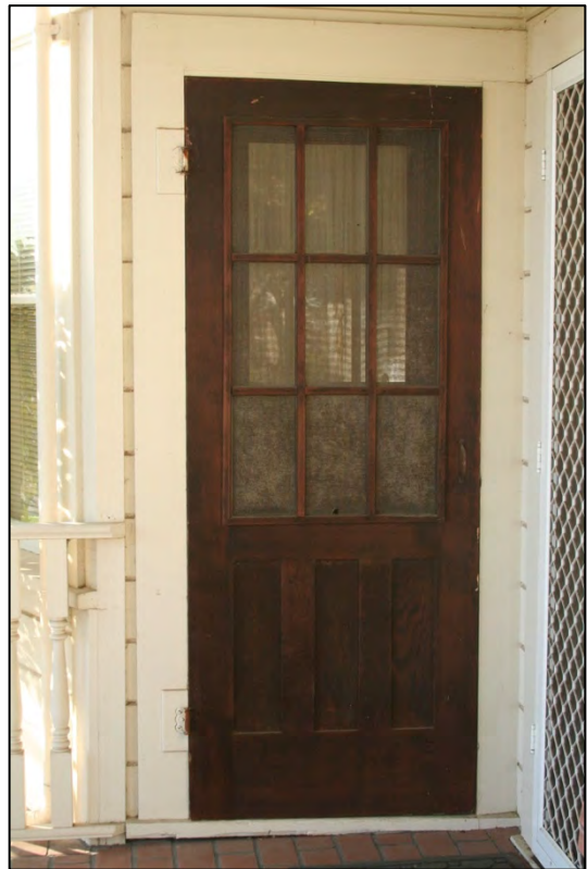
Figure 4: South facade, porch - side door
