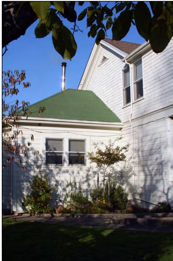
Figure 16: West elevation, junction of west wing
