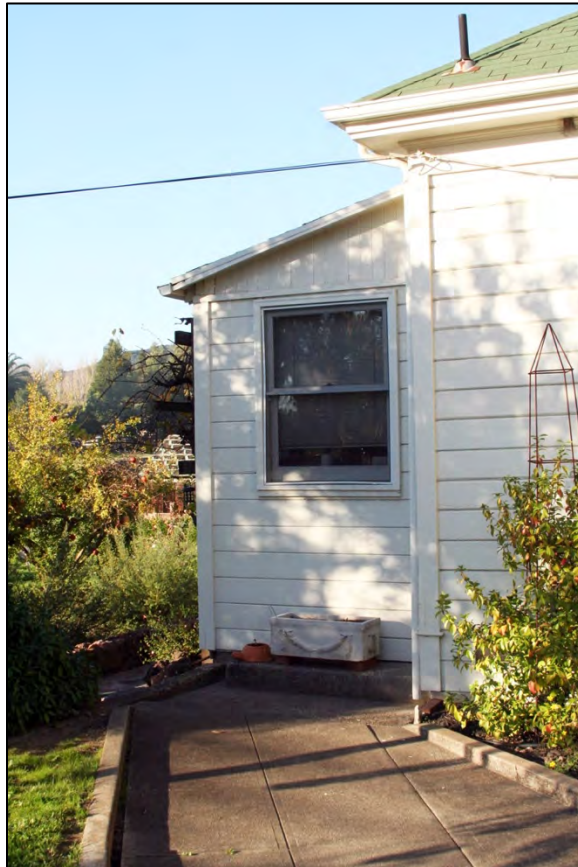
Figure 12: South facade, enclosed porch off of west wing
