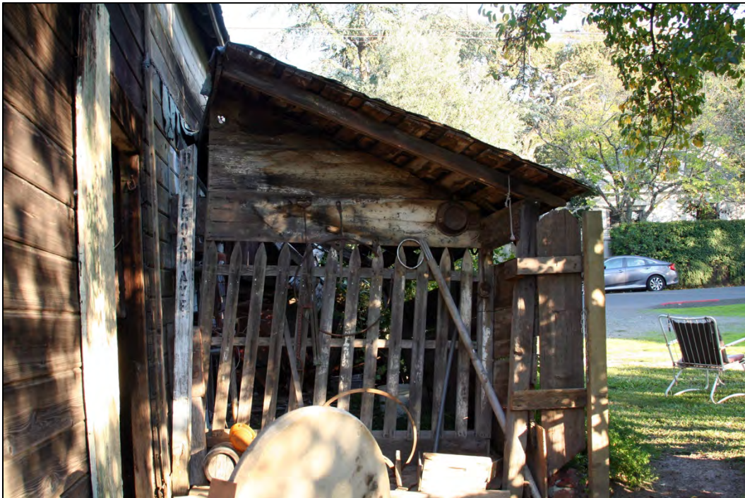
Figure 30: Dairy Barn, south wing looking east
