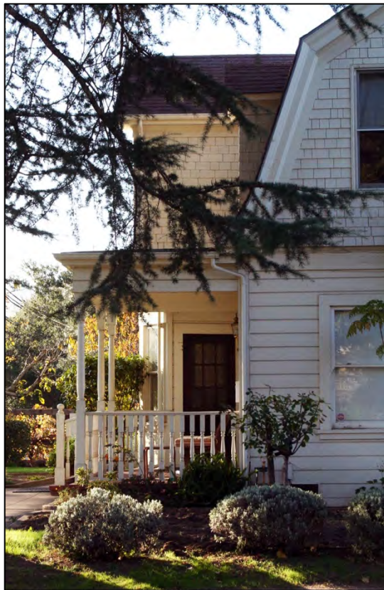
Figure 26: View of front porch from east elevation (2nd St. East)
