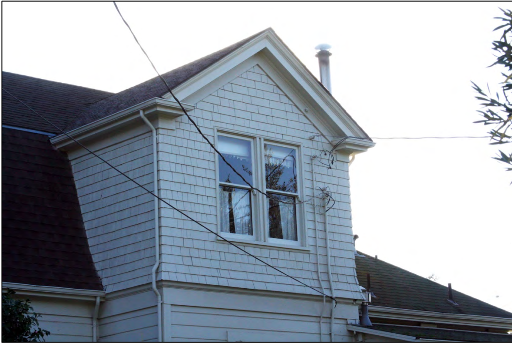
Figure 21: North elevation, pair of windows at second story
