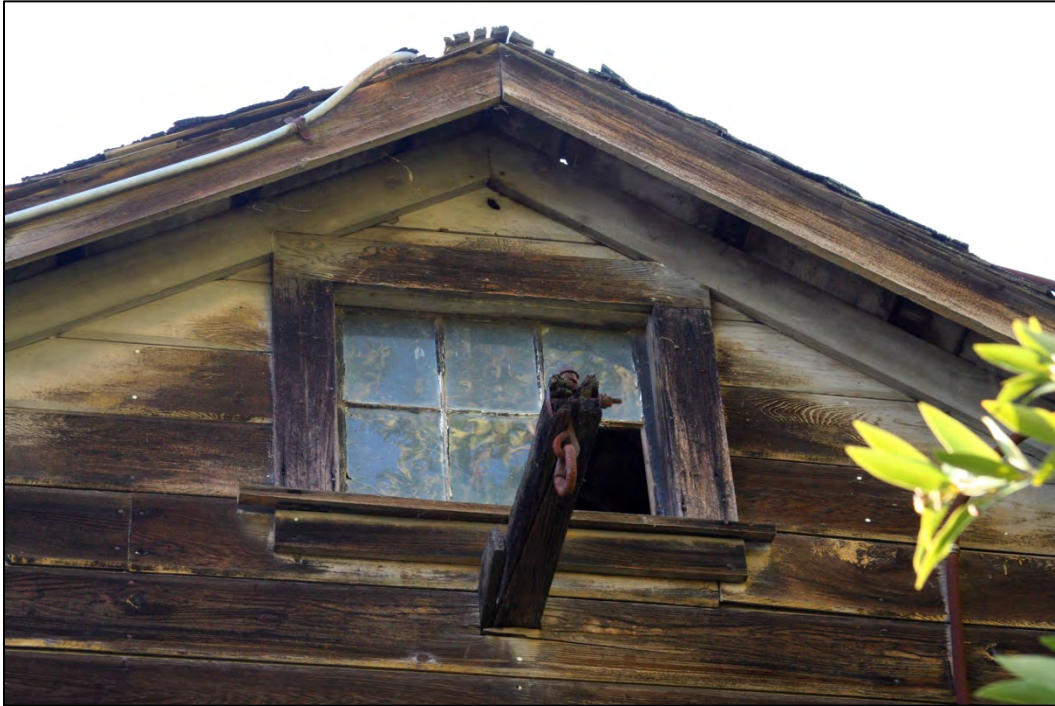
Figure 29: Dairy barn, east elevation gable detail
