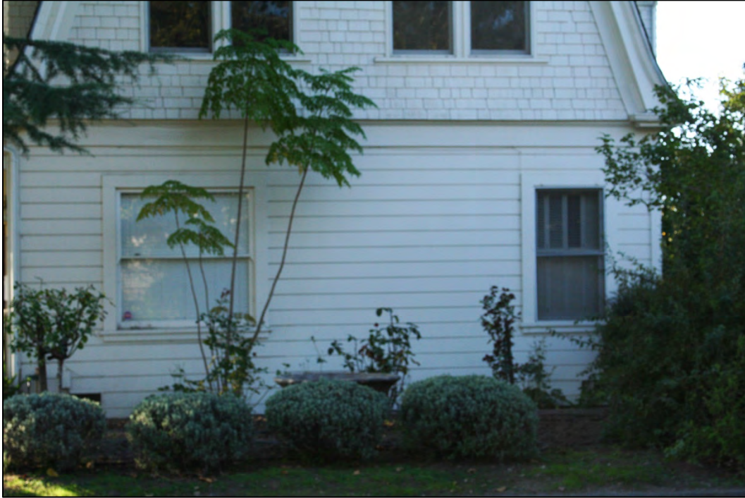
Figure 25: East elevation, first story windows
