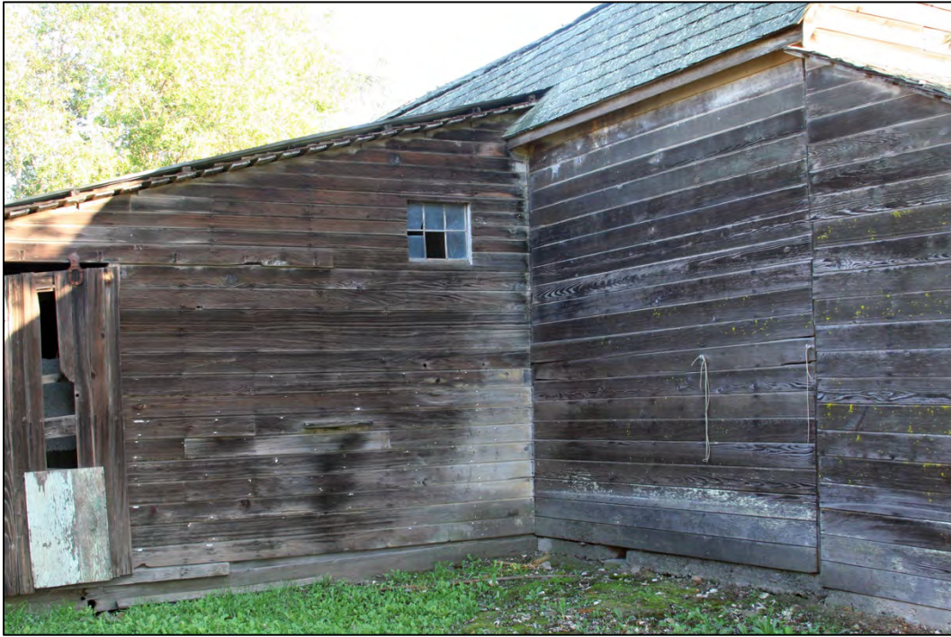
Figure 35: Dairy barn, west elevation of north wing
