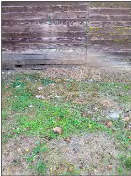
Adobe and earthen alignment, view south. (Photo Acc. No.: ASC-2208-14)
