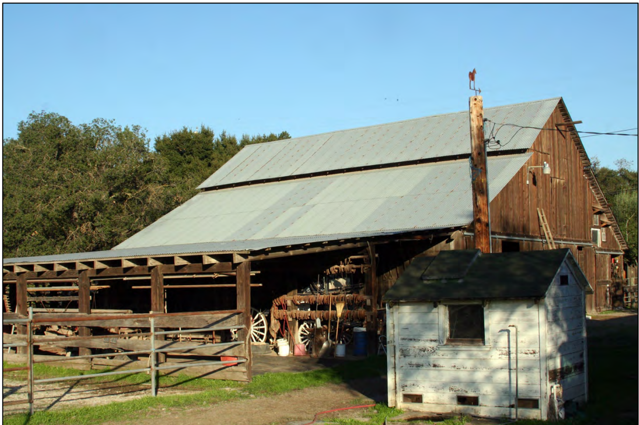
Figure 50: Horse barn, southwest corner (and well house in foreground)
