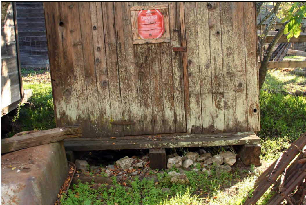
Figure 51: "Dick's Cabin," north elevation
