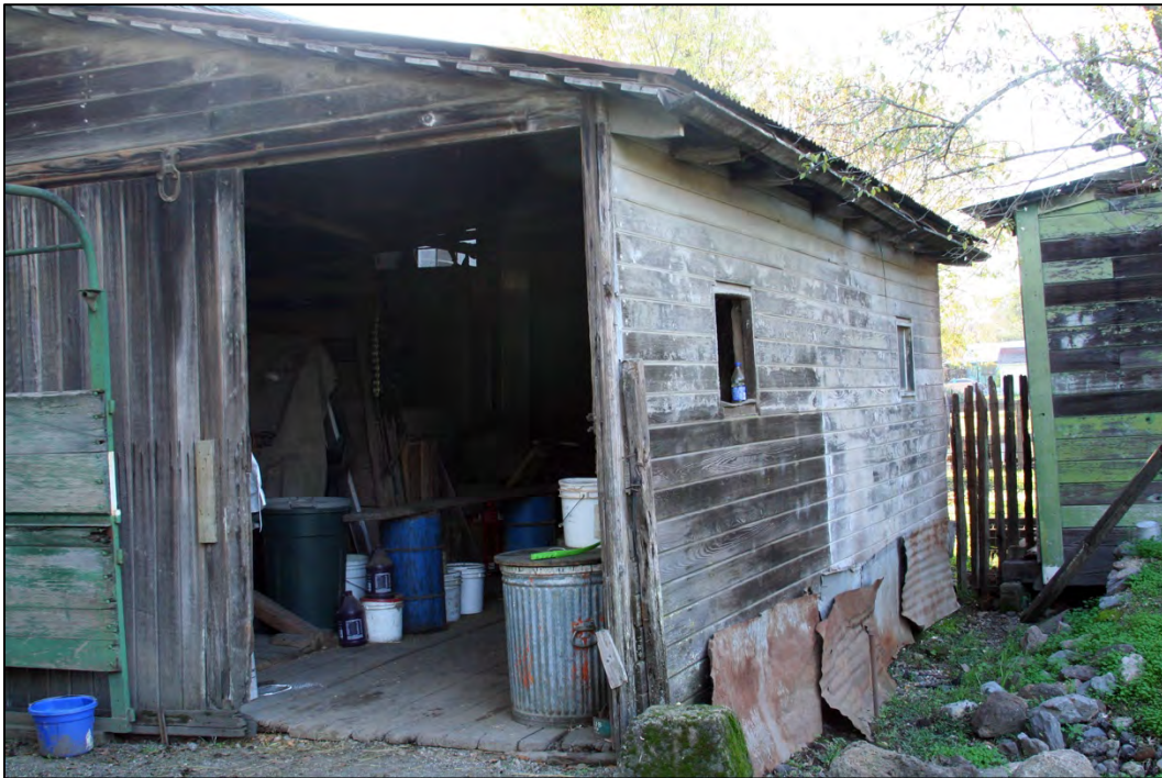
Figure 34: Dairy barn, northeast corner (north wing)
