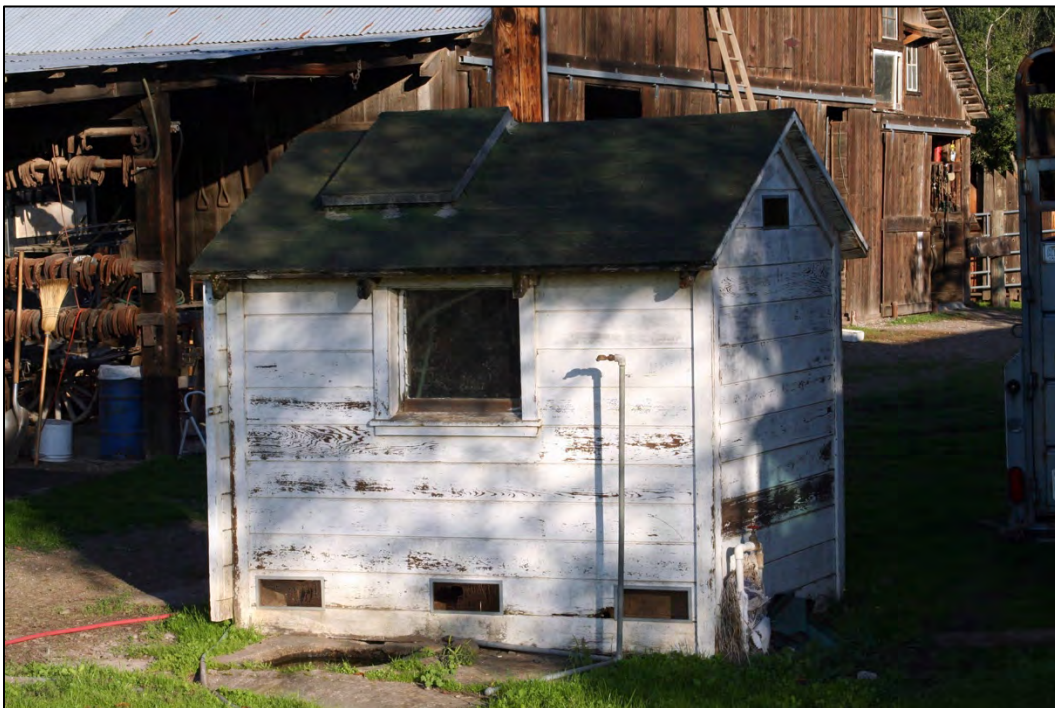
Figure 59: Well house, west elevation
