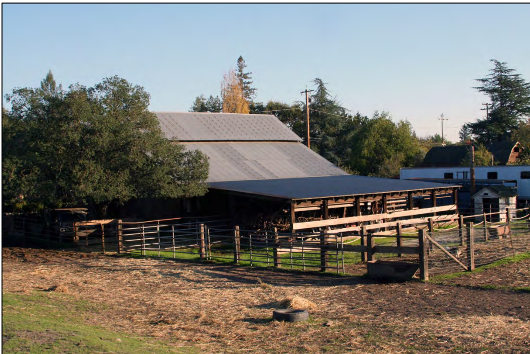
Figure 48: Horse barn, west elevation and wing
