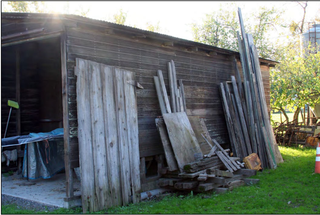
Figure 56: Outbuilding relocated from high school, north elevation
