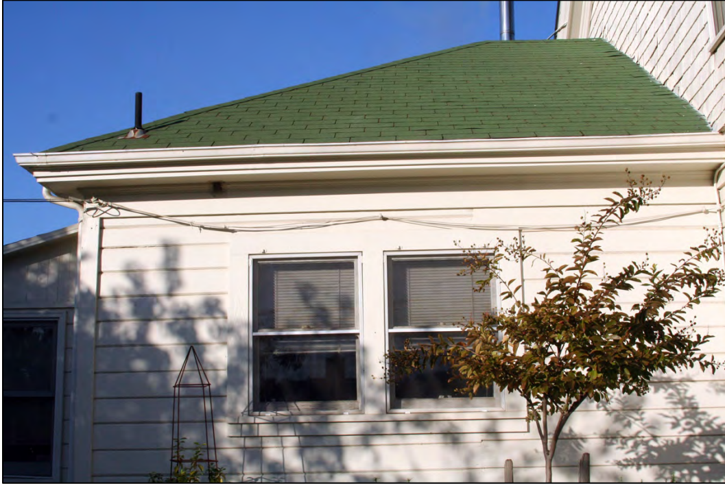
Figure 11: South facade, west wing, pair of windows
