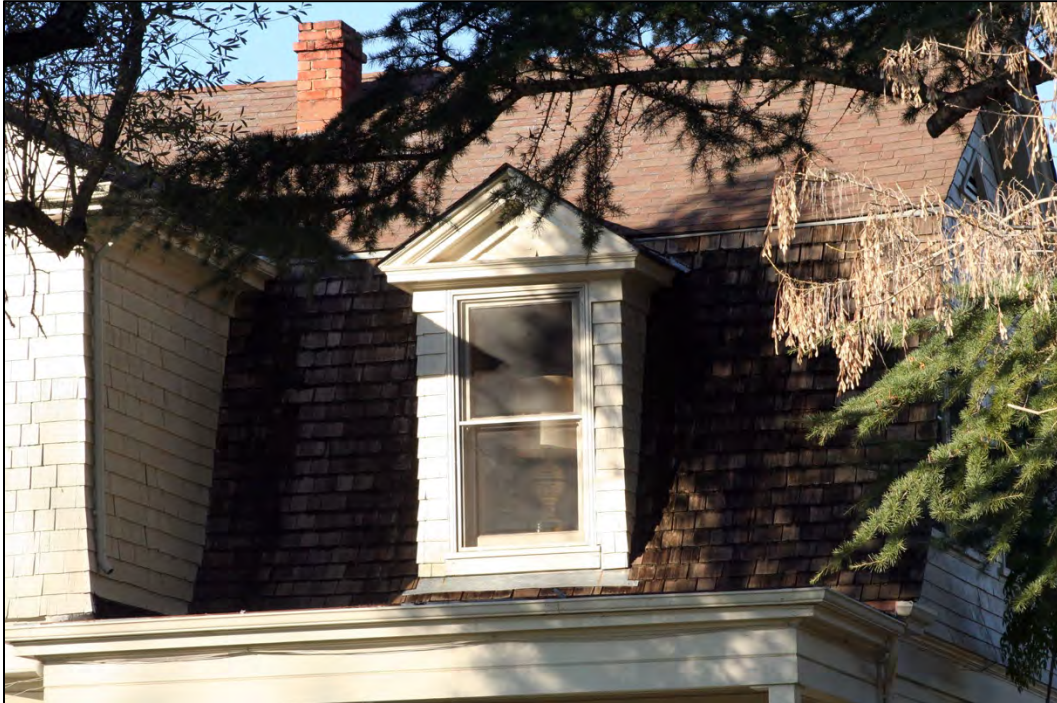
Figure 8: South facade, gabled dormer window
