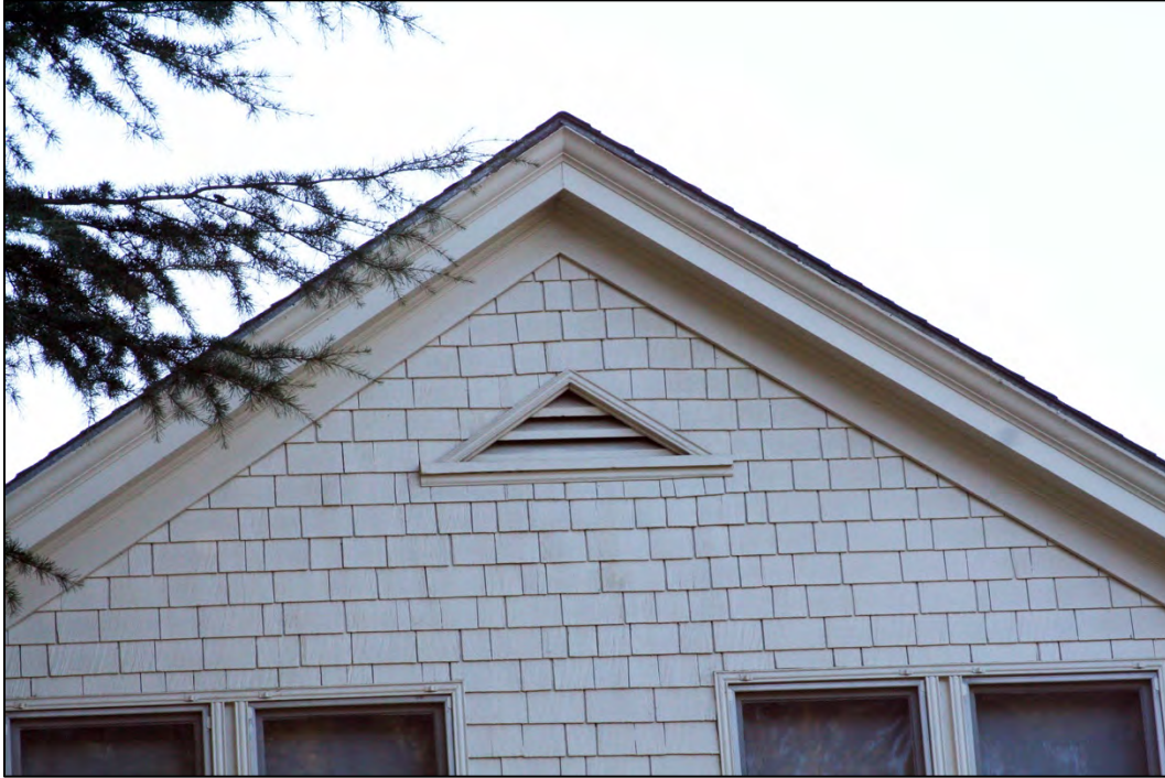
Figure 23: East elevation, triangular gable vent
