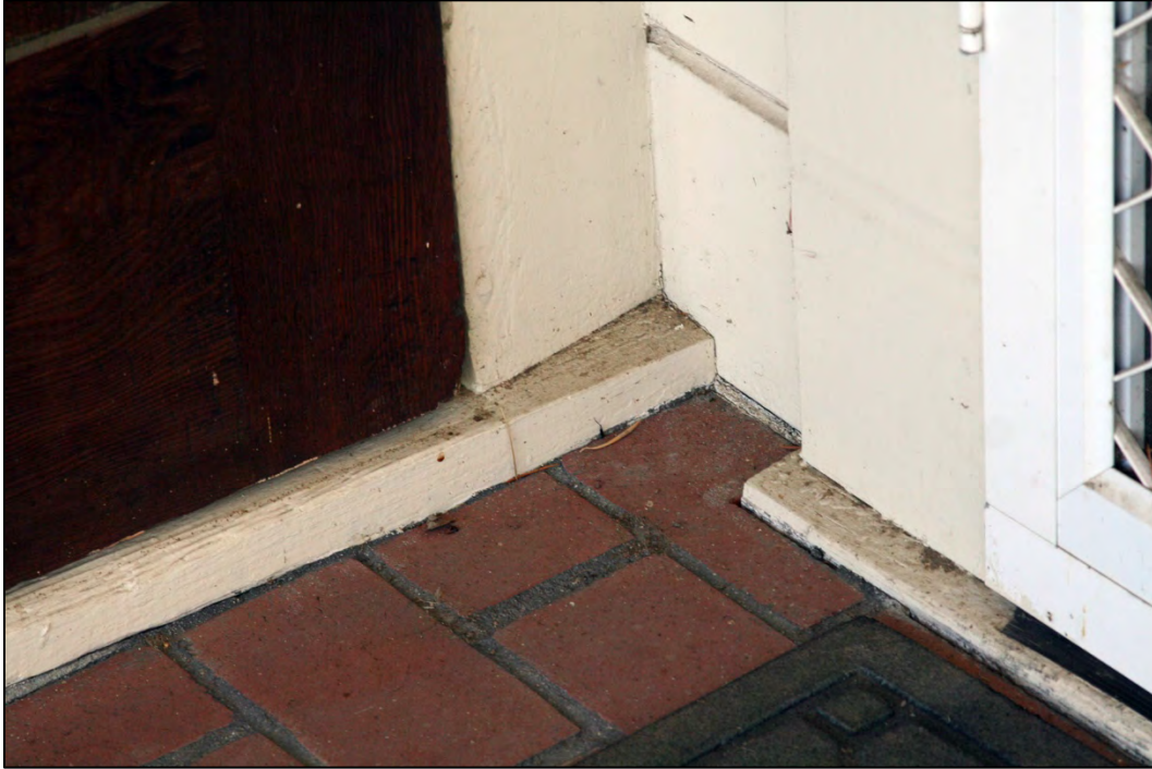
Figure 5: South facade, porch floor
