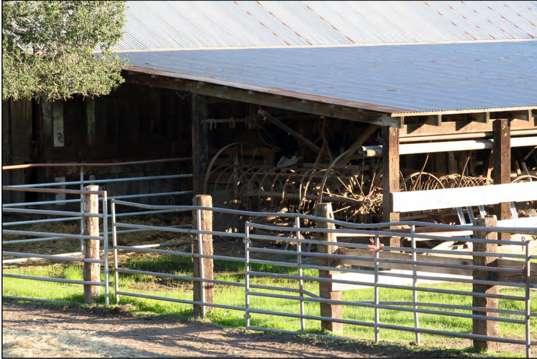
Figure 47: Horse barn, northwest corner
