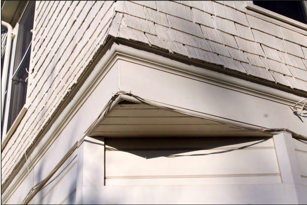
Figure 7: South facade, bay window eave detail
