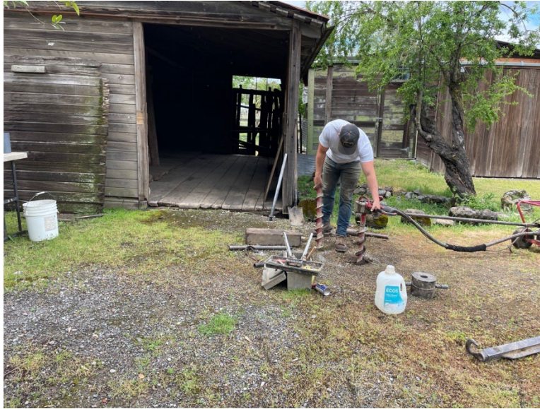
Borehole 5 facing w
