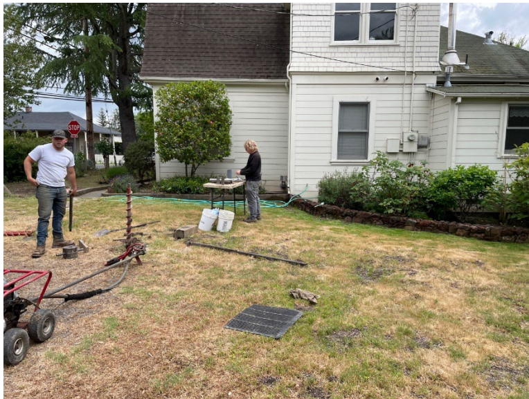
Borehole 6 facing S toward main house.
