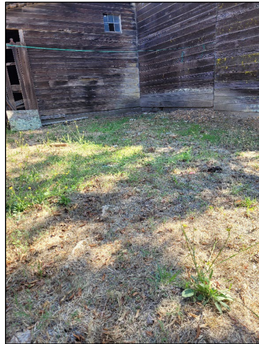
Adobe and earthen alignment, view southeast. (Photo Acc. No.: ASC-2208-13)
