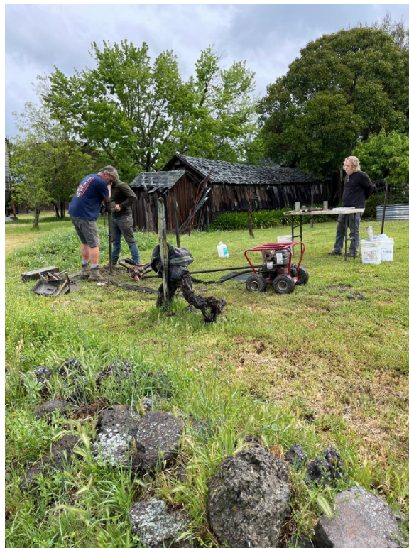
Borehole 2 in progress, facing NNE (shed of horse barn in background)
