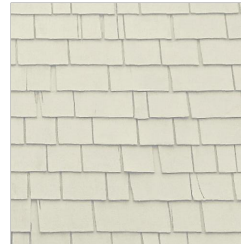
PAINTED HORIZONTAL WOOD SIDING AND WOOD SHINGLES AT EXISTING MAIN HOUSE TO REMAIN
