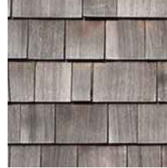
CEDAR SHINGLE ROOFING, TYPICAL
