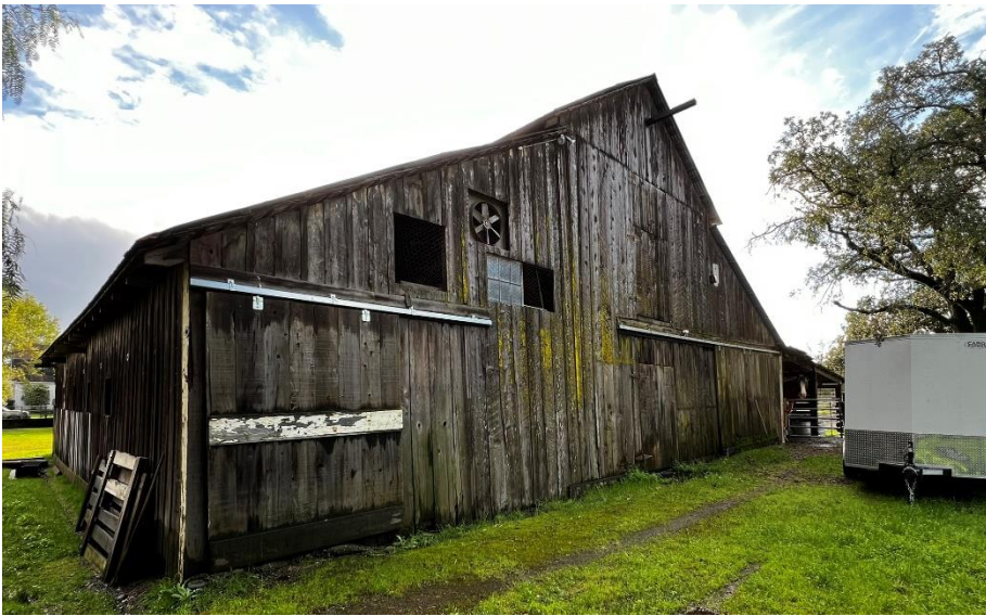
Horse Barn (BLDG. 9) (to remain)
