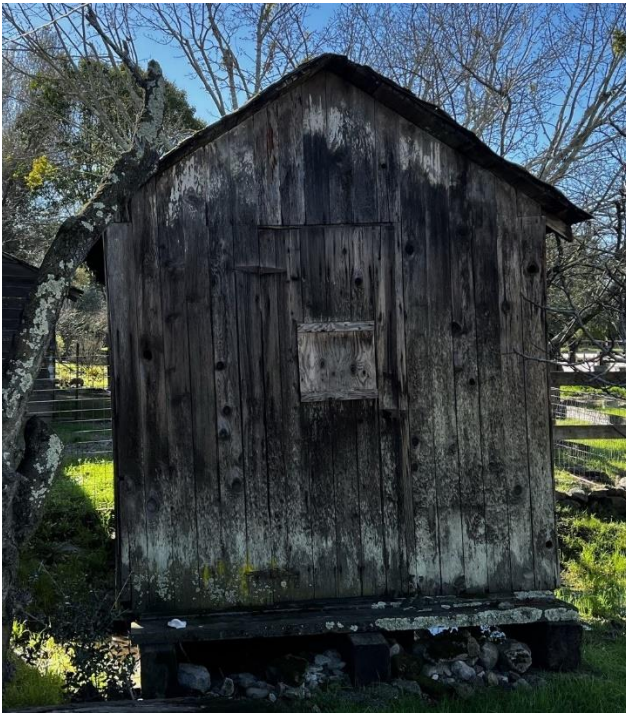
Shed (BLDG. 5) (to remain)
