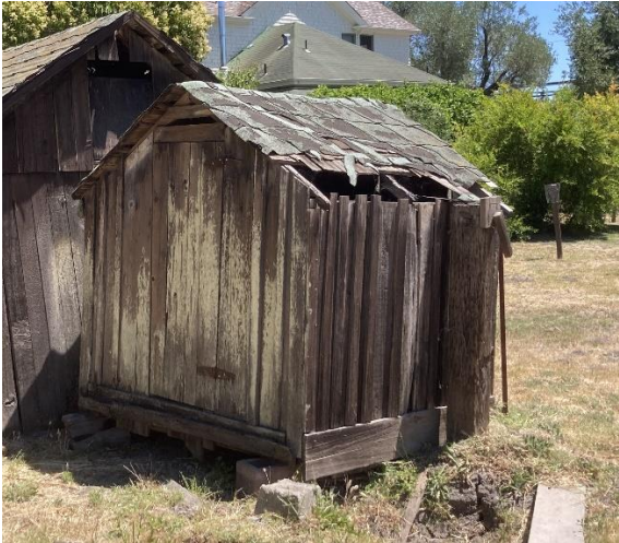
Storage shed (BLDG. 2) (to be relocated on site and rebuilt/repaired)
