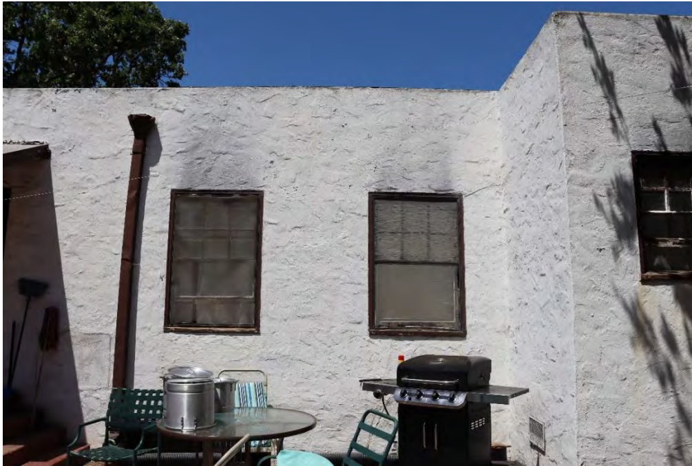
Figure 10. East elevation, facing north.
