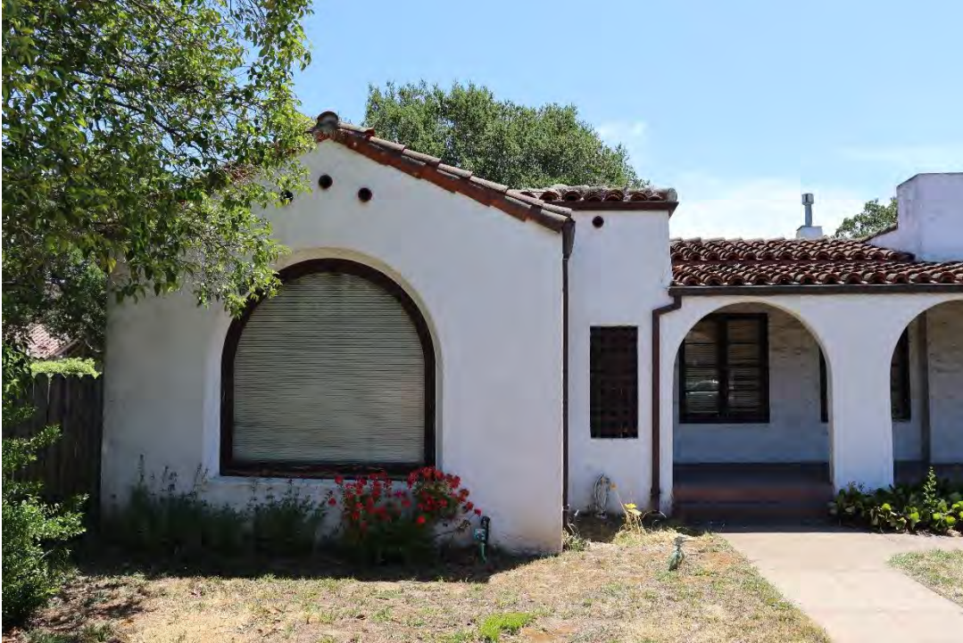
Figure 24. Photo showing the west elevation with fixed arched picture window along the projecting gable wing, facing east.
