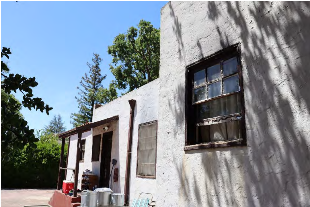
Figure 31. East elevation, facing south.
