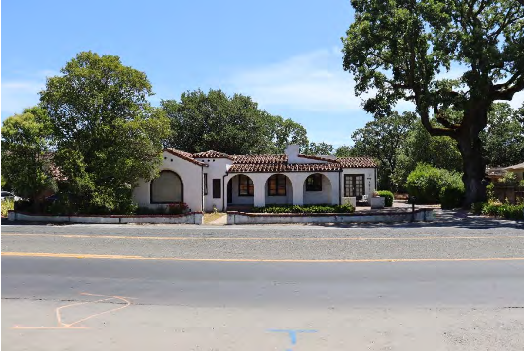
Figure 20. West elevation, facing east.
