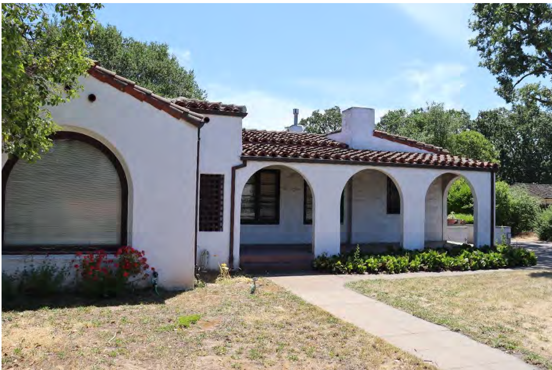
Figure 21. West elevation, facing east.
