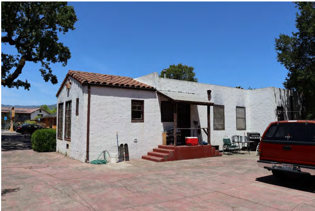
Figure 9. East elevation, facing north.
