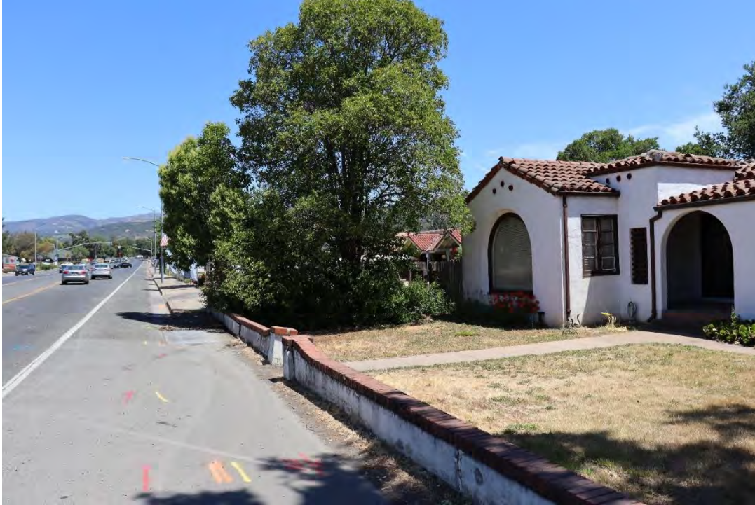
Figure 33. Photo showing the low garden wall along the western boundary of the Property, facing north.
