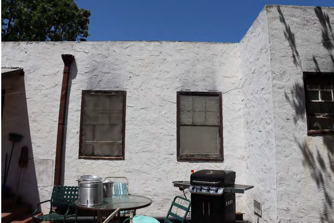
Figure 30. East elevation, facing north.
