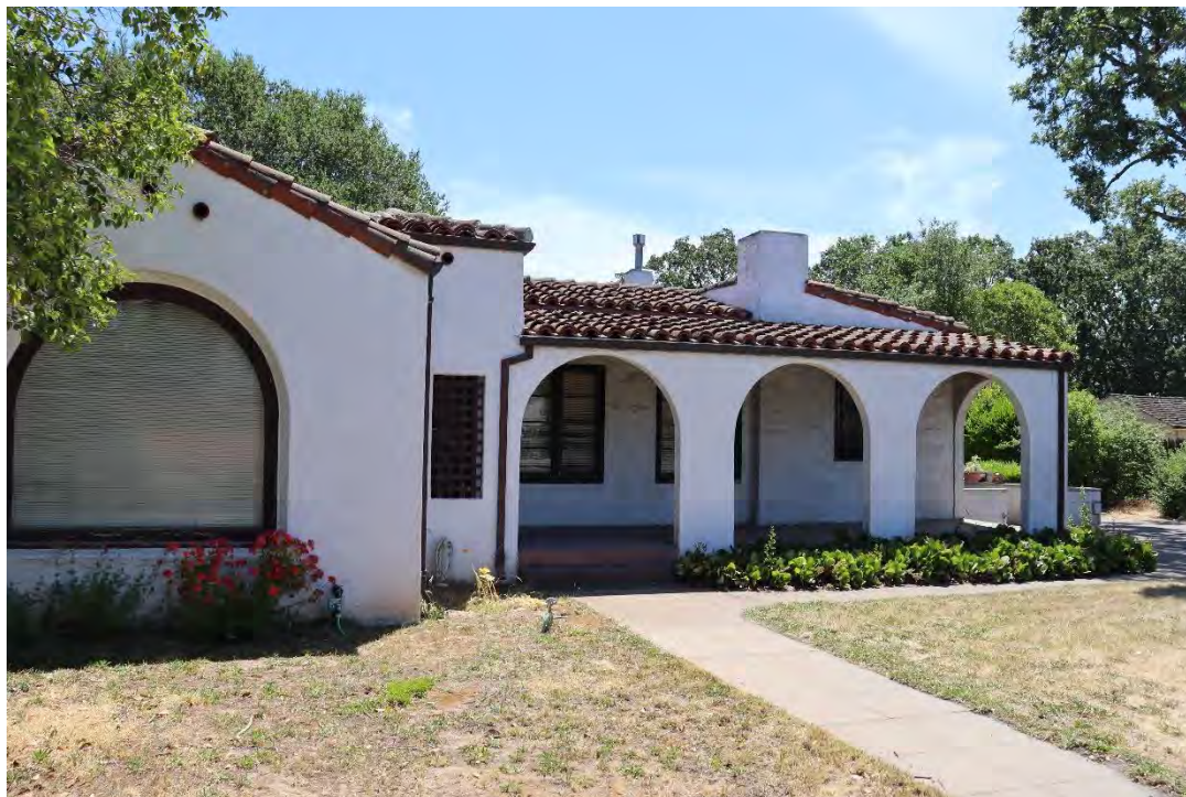
Figure 1. West elevation, facing east.
