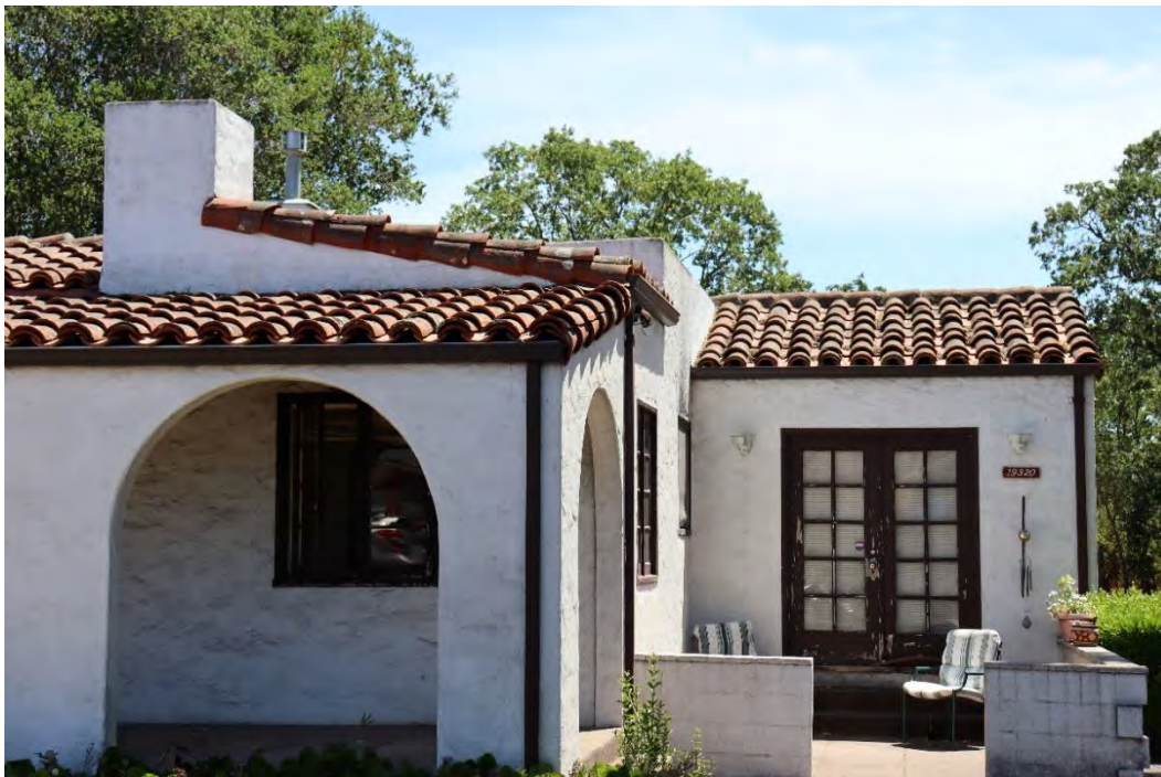
Figure 5. Photo showing the open courtyard along the primary façade.
