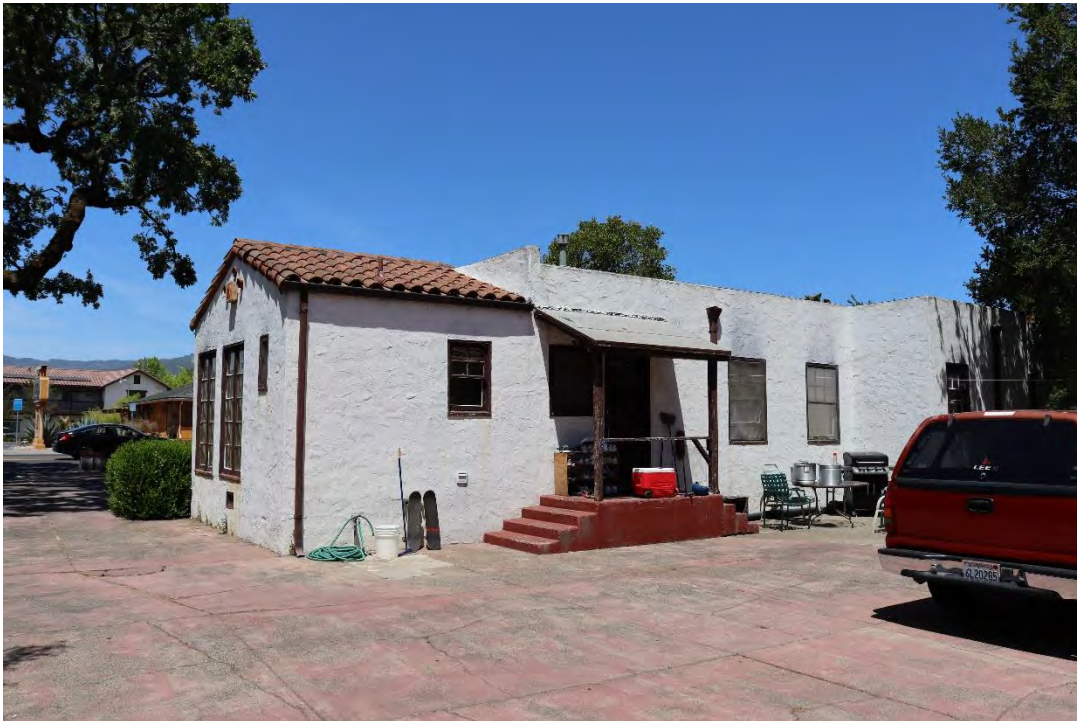
Figure 29. East elevation, facing north.
