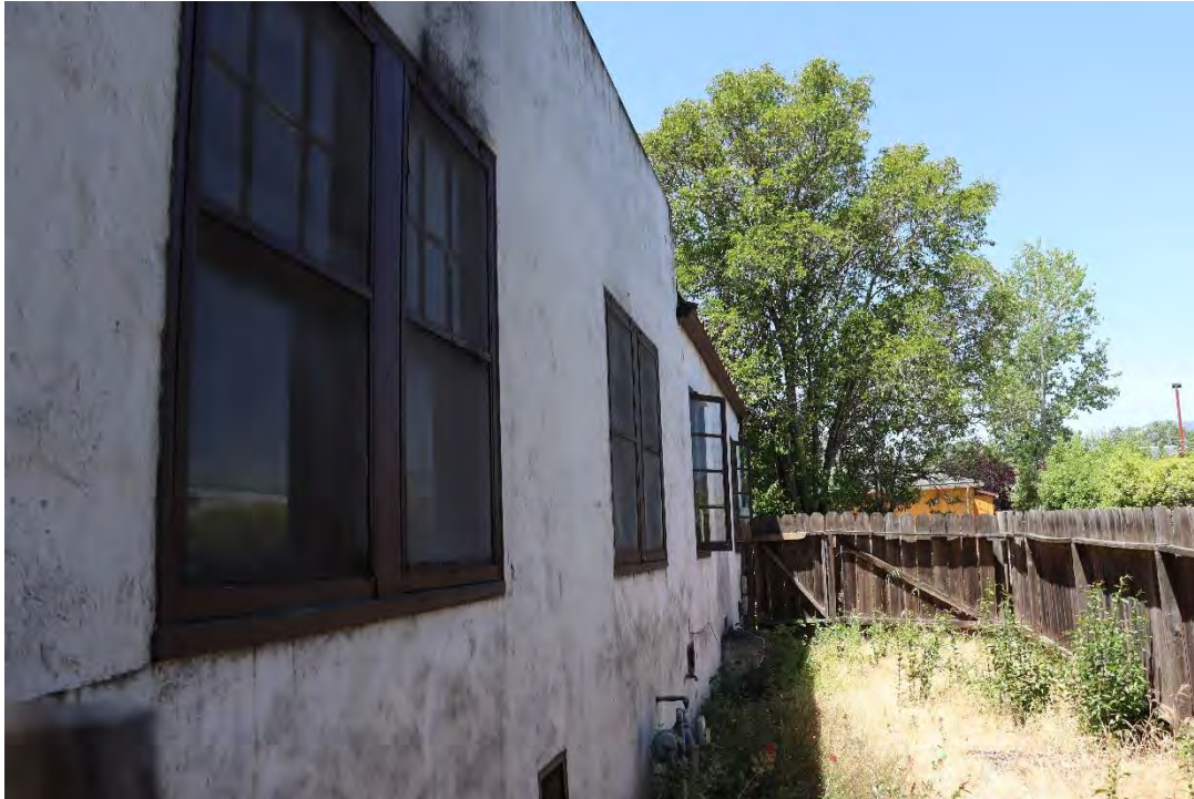
Figure 12. North elevation, facing west.
