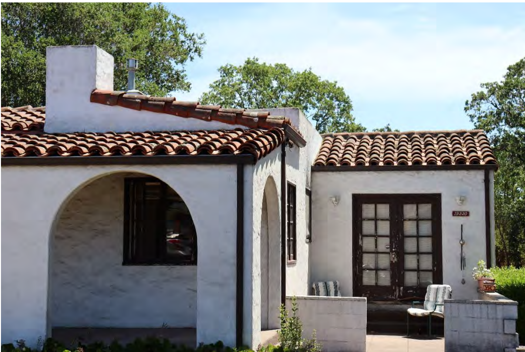
Figure 25. Photo showing the west elevation with an open courtyard, facing east.
