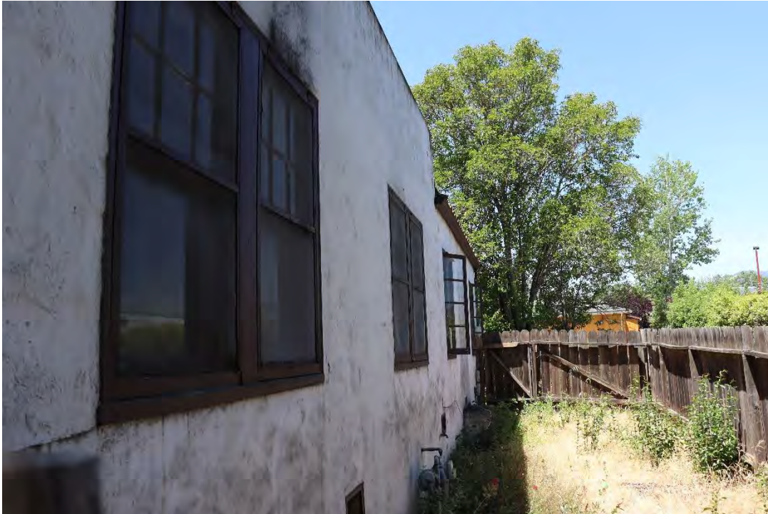
Figure 32. North elevation, facing west.
