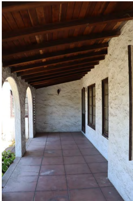
Figure 23. Photo showing the wooden beams and wood ceiling.
