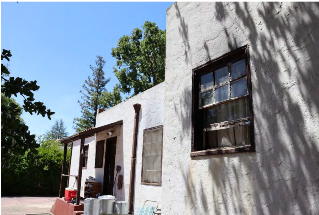
Figure 11. East elevation, facing south.
