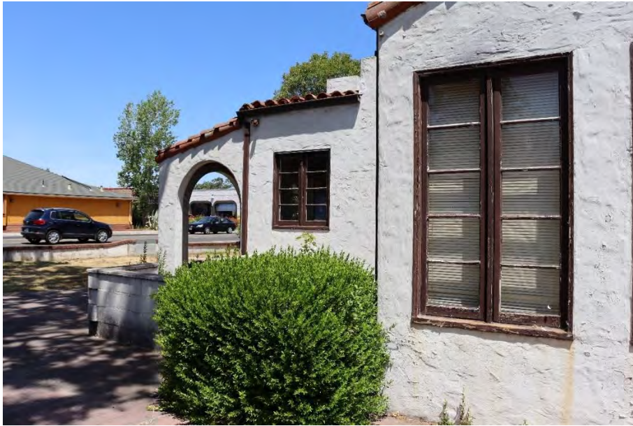
Figure 7. South elevation, facing northwest.
