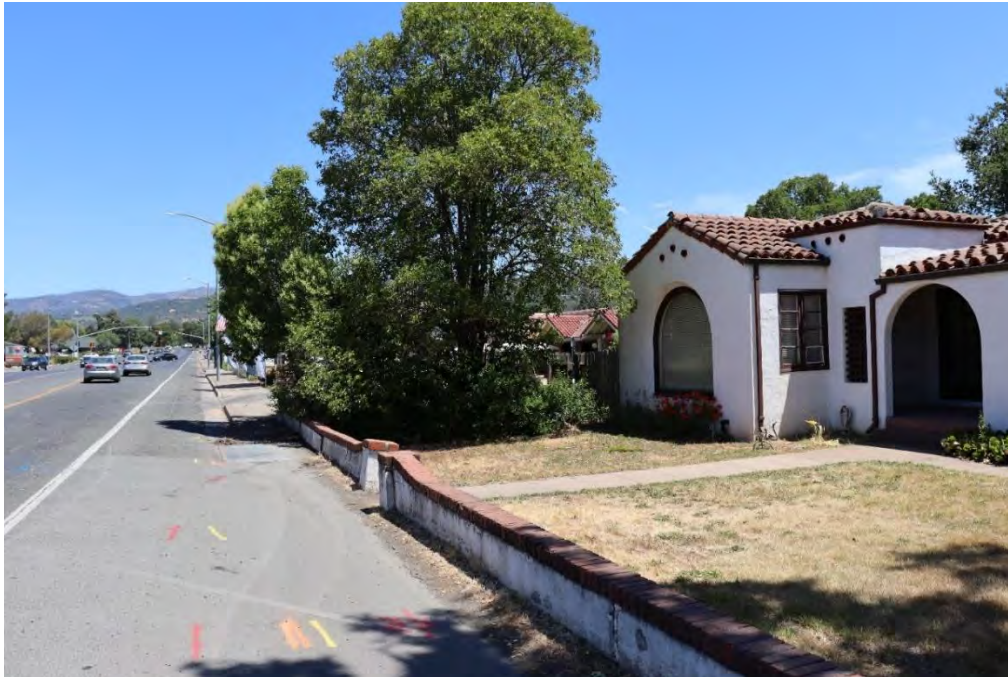
Figure 13. Photo showing the low garden wall along the western boundary of the property, facing north.
