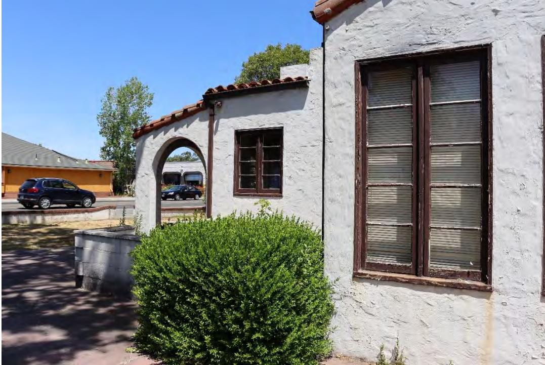
Figure 27. South elevation, facing northwest.
