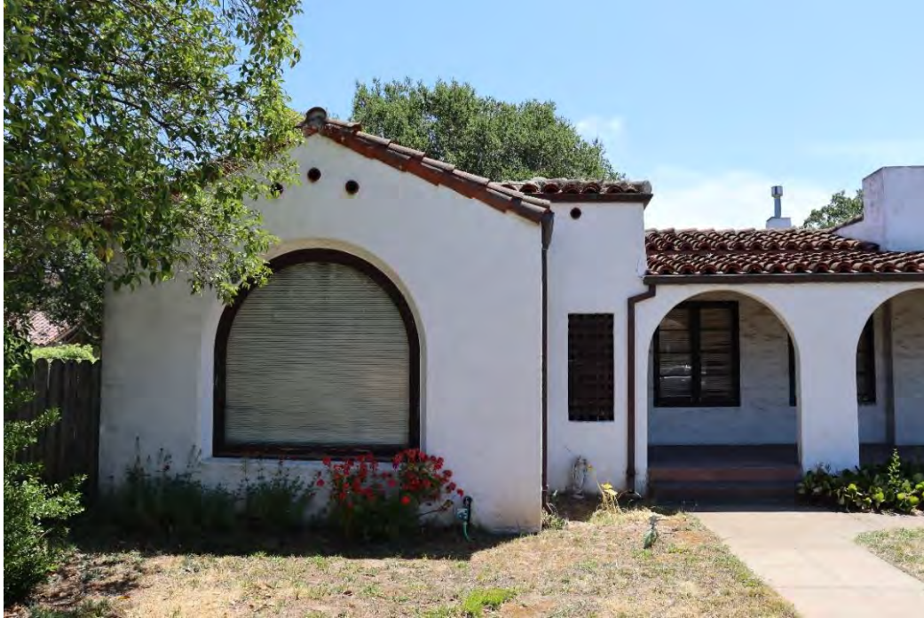
Figure 4. Photo showing the fixed arched picture window along the projecting gable wing, facing east.
