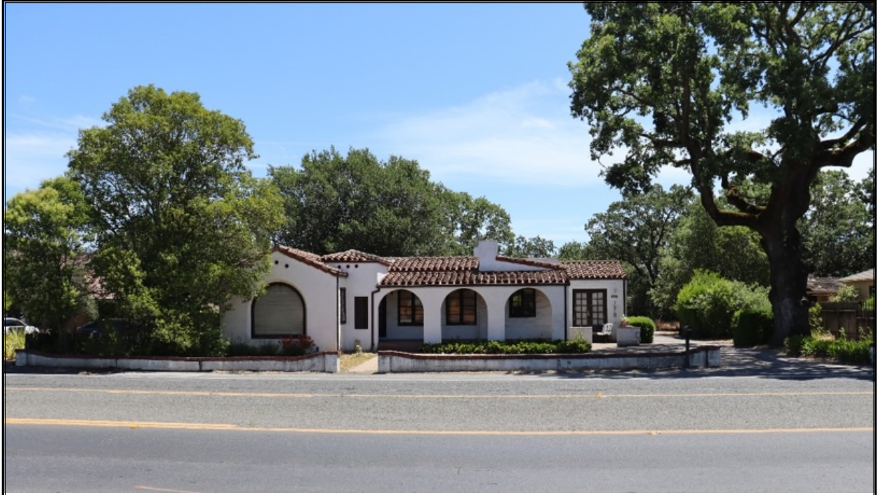
View looking east at the single-family home from Highway 12
