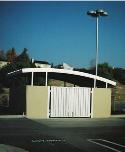
Figure 3.1. Roofed and bermed refuse area.
