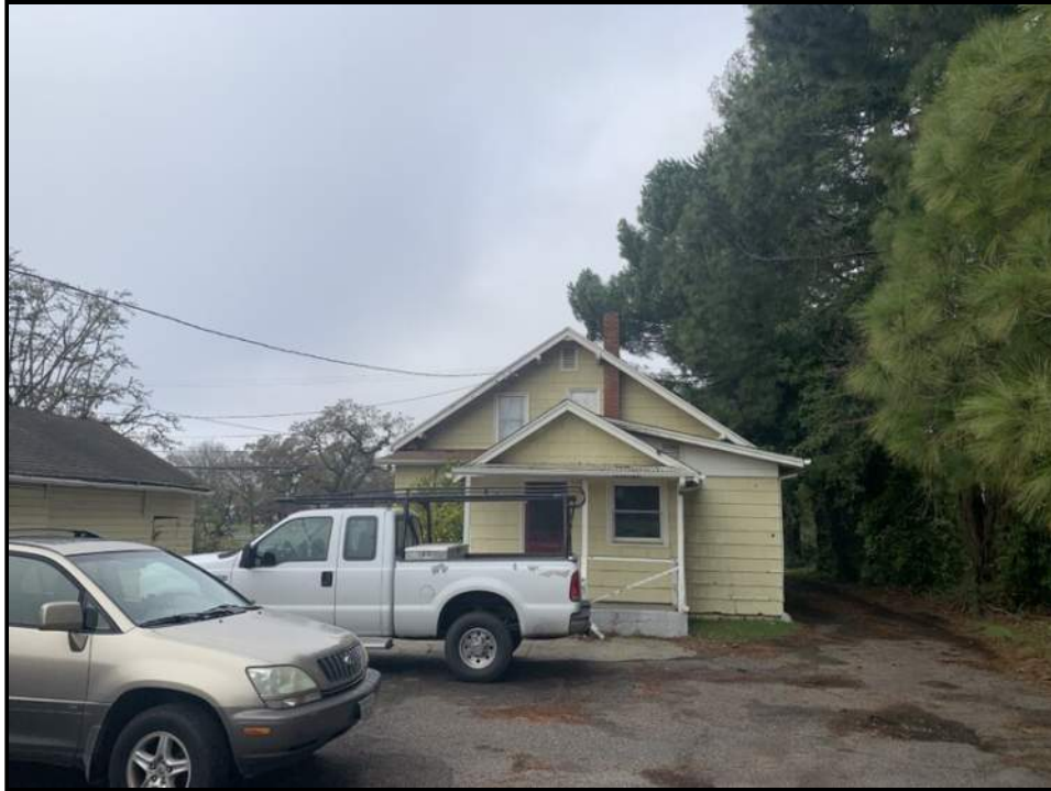
Photo 4: View of the northwest residential structure looking to the west.
