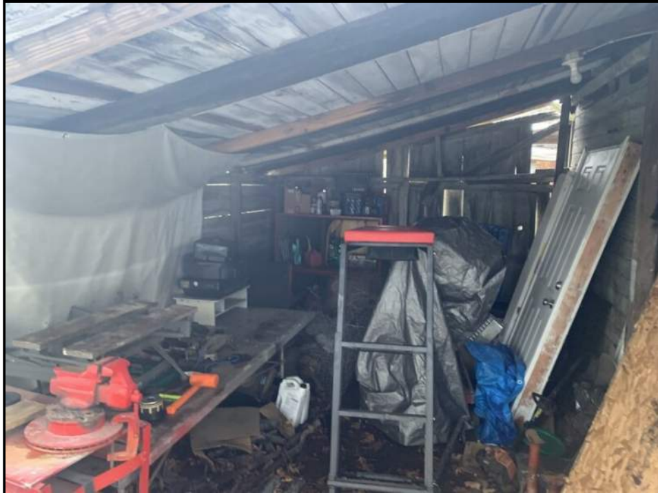
Photo 14: View of interior area of a barn.
