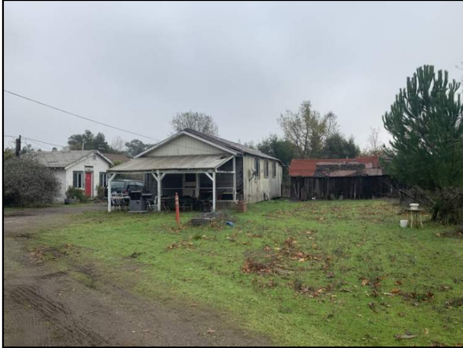
Photo 5: View of a storage structure in the center, a residential structure on the left and a barn on the right.
