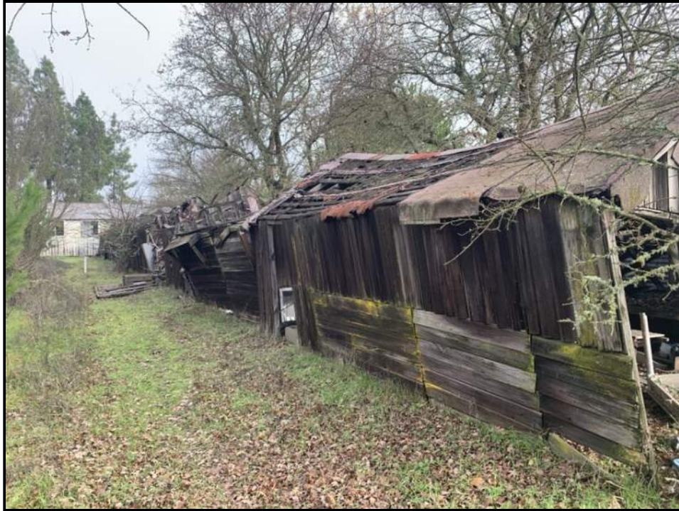
Photo 18: View of barn falling apart on the central portion of the Subject Property.
