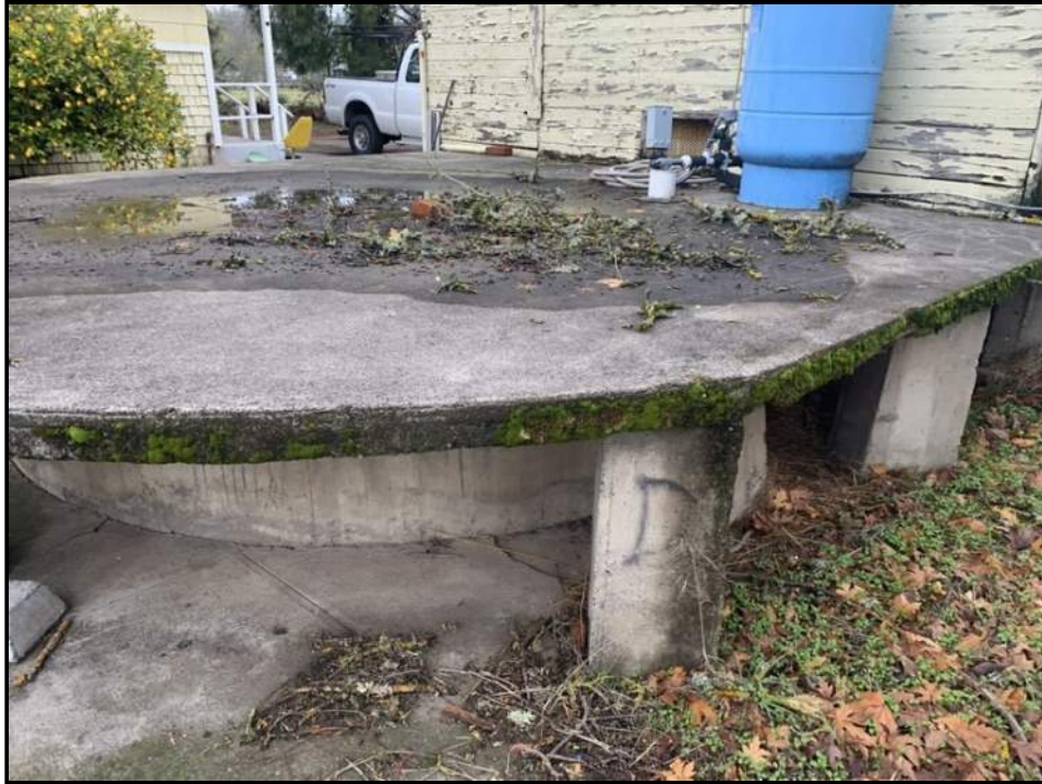
Photo 12: View of base of water well.
