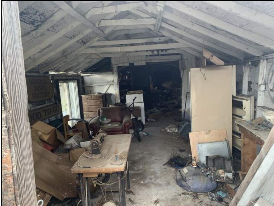
Photo 16: View of interior of barn structure.
