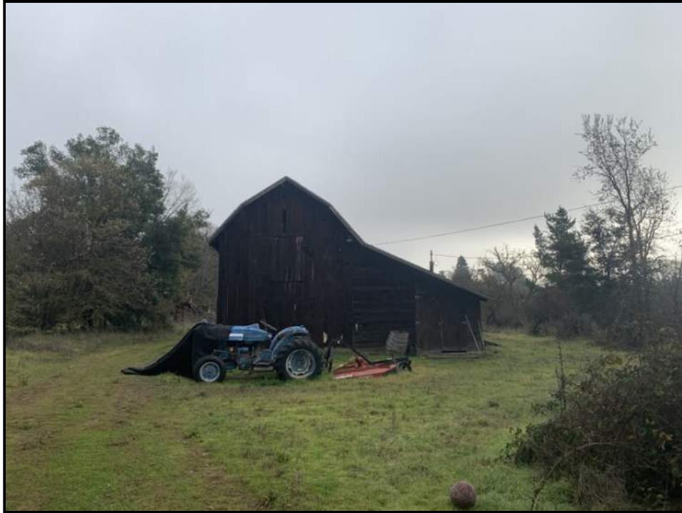
Photo 15: View of barn structure.
