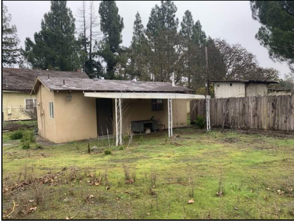
Photo 9: View of storage structure.
