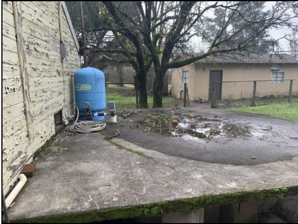
Photo 10: View of water well.
