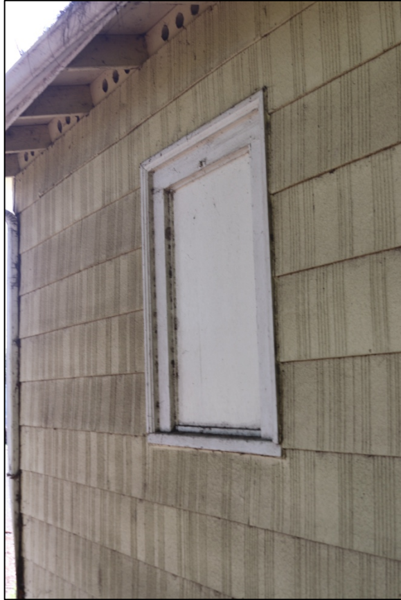
Figure 29: North elevation, infilled window
