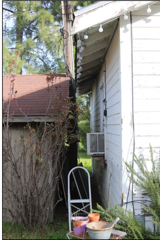
Figure 31: Two sections do not abut
