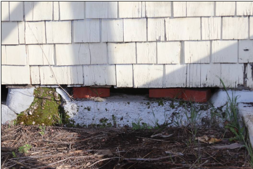
Figure 16: South elevation, foundation detail, random bricks
