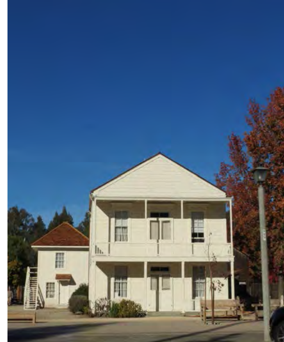
Toscano Hotel Annex and Tank House, contributors to both the Sonoma Plaza National Historic Landmark and the Sonoma Plaza National Register Historic District.
