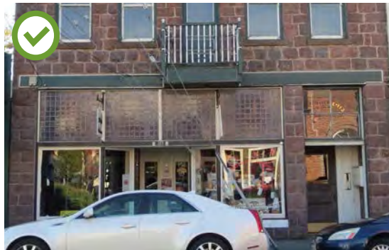
Original transom windows contribute to the historic character of the commercial building and should be retained.
