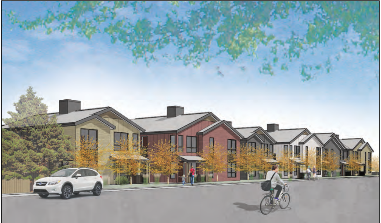
Clay Street frontage, looking east.
