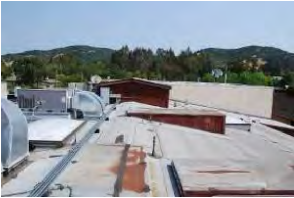
Figure 26: Roof, facing north.
