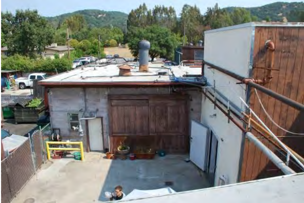
Figure 25: West facade, rear (north) portion, taken from the roof, facing north.
