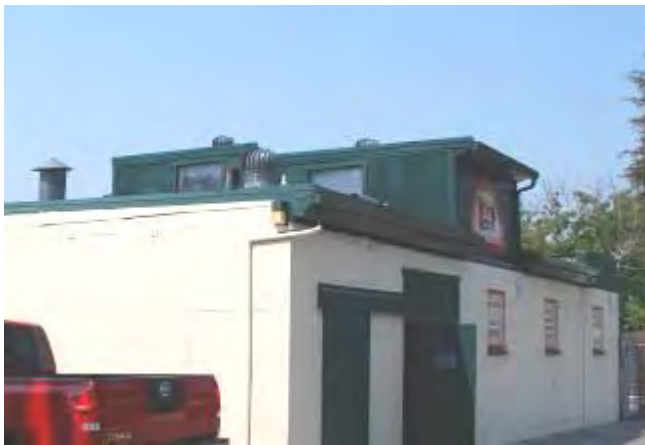
Figure 18: Rear (north) facade, mezzanine mass, facing southwest.
