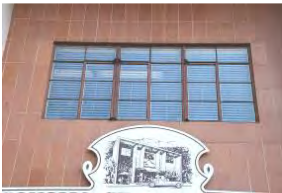
Figure 7: Primary facade, second story center window group, facing north.
