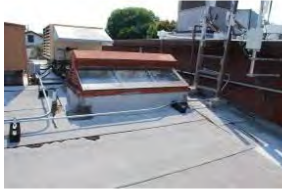
Figure 27: Roof, including monitor skylight, facing west.
