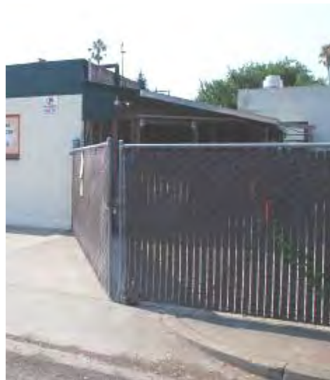
Figure 19: Rear (north) facade, fenced utility yard and open porch at right (west), facing south.
