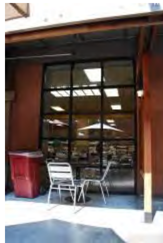
Figure 13: East facade, center portion, right multi-lite window, facing west.
