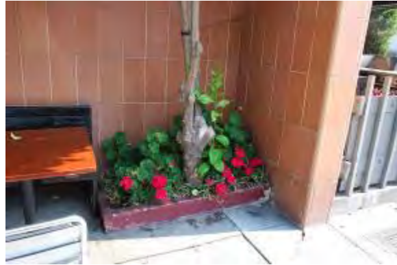
Figure 6: Primary facade, planter at right, facing northeast.
