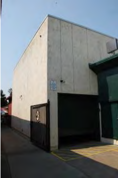
Figure 15: East facade, rear portion, two-story mass, facing southwest.
