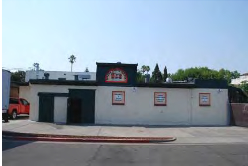
Figure 17: Rear (north) facade, facing south.
