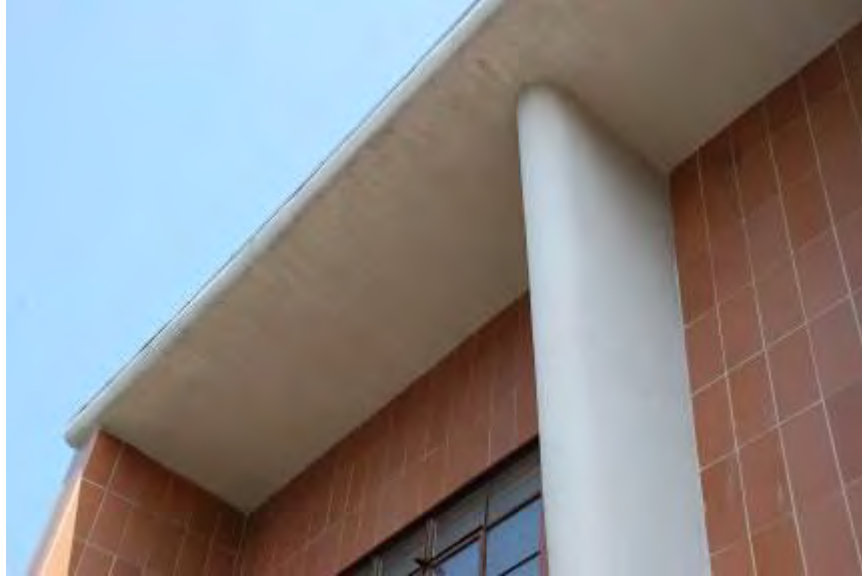
Figure 9: Primary facade, roofline, facing northwest.
