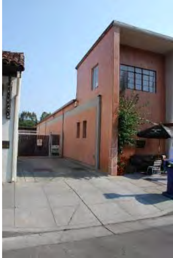
Figure 22: West facade, facing northeast.
