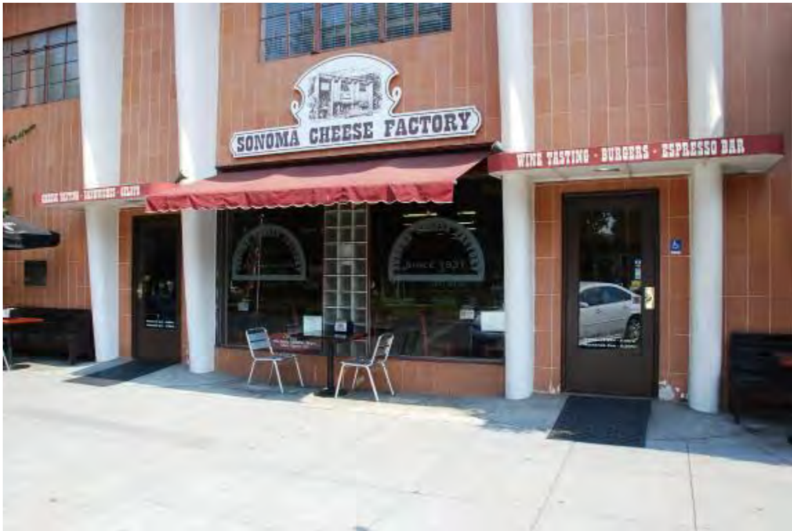
Figure 4: Primary facade, primary entrances, facing northwest.
