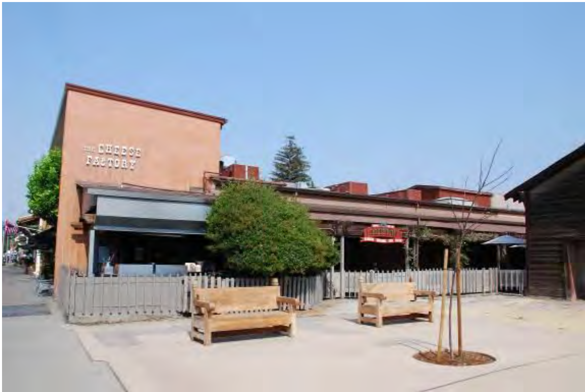
Figure 10: East facade, front and center portions of the building, facing west.
