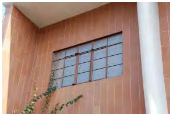
Figure 8: Primary facade, second story left window group, facing northwest.
