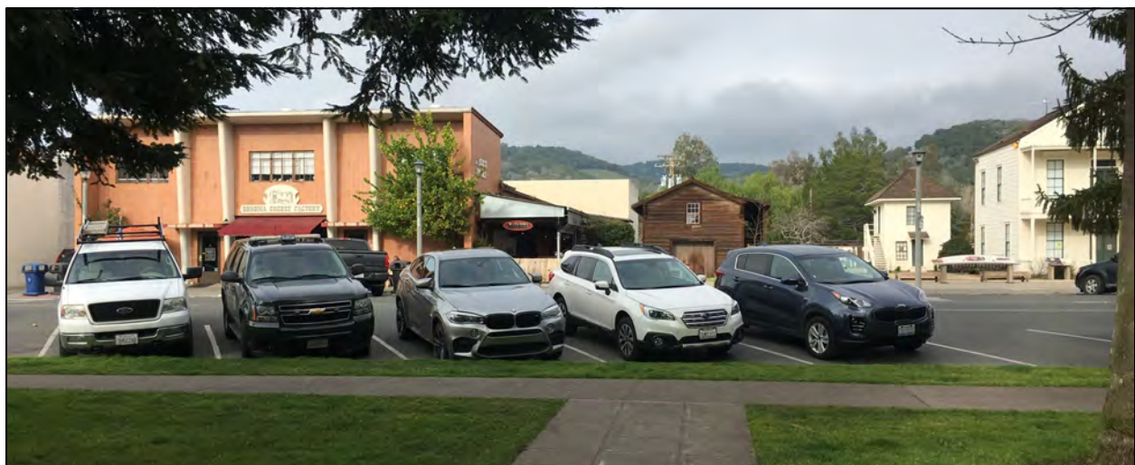
Sonoma Cheese Factory, Existing View from South.
