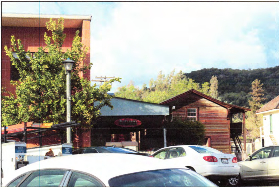
Figure 2: South facade (West Spain Street), covered dining and path
