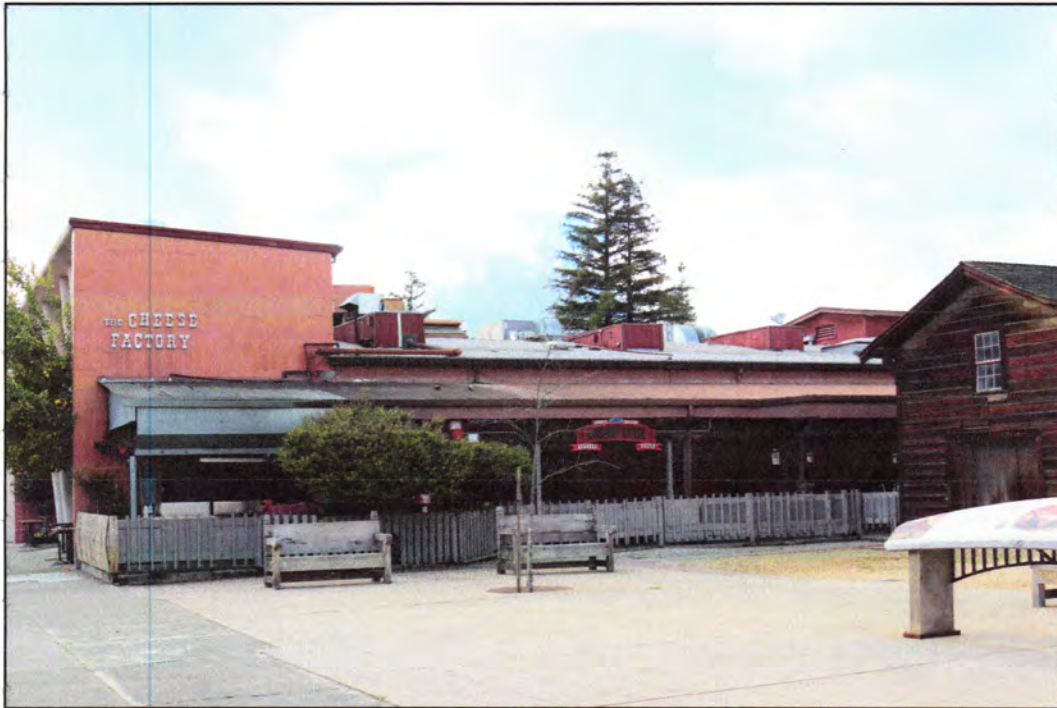
Figure 1: East Facade, one-story character defining block (massing)
