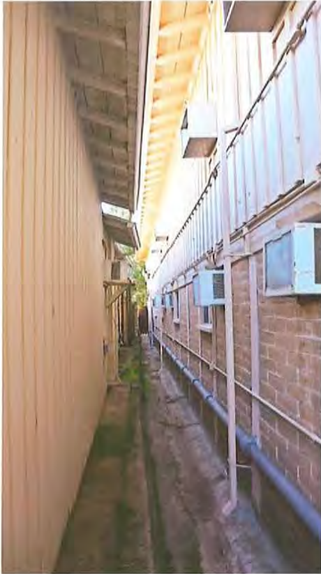
Secondary Dwelling, south elevation (left), facing east.
