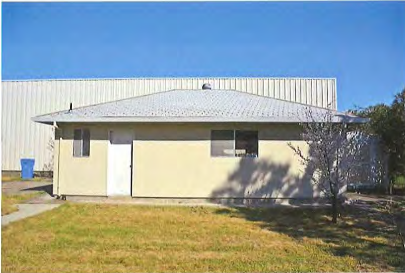
Garage, south elevation, facing north.
