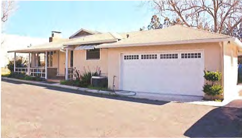
Main House, west and partial south elevations, facing northeast.
