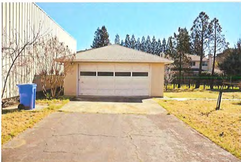
Garage, west elevation, facing east.
