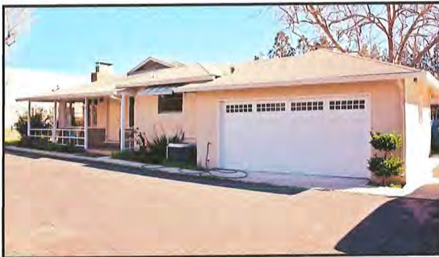
Figure 3: Main House, west elevation, facing northeast.
