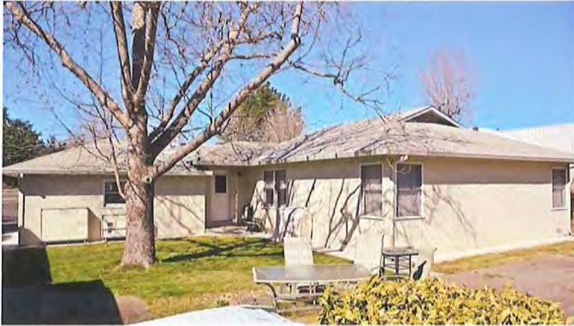
Main House, east elevation, facing west.
