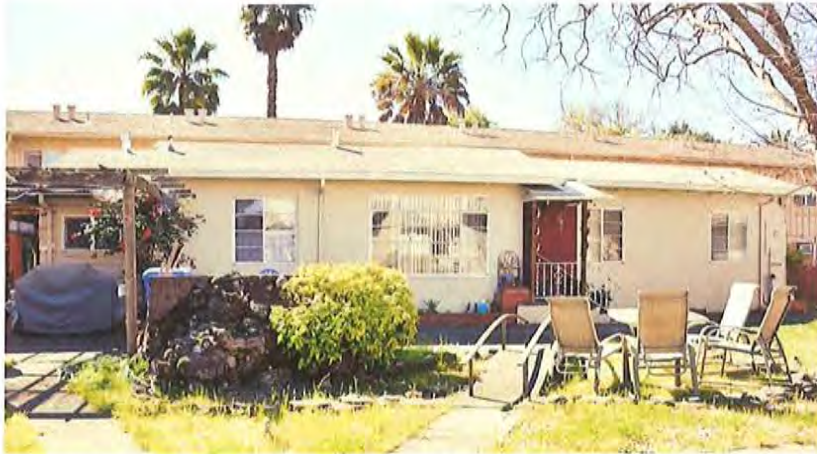
Secondary Dwelling, north elevation, facing southwest.
