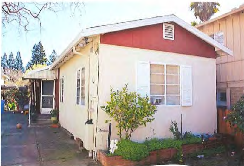
Secondary Dwelling, partial north and west elevations, facing southeast.
