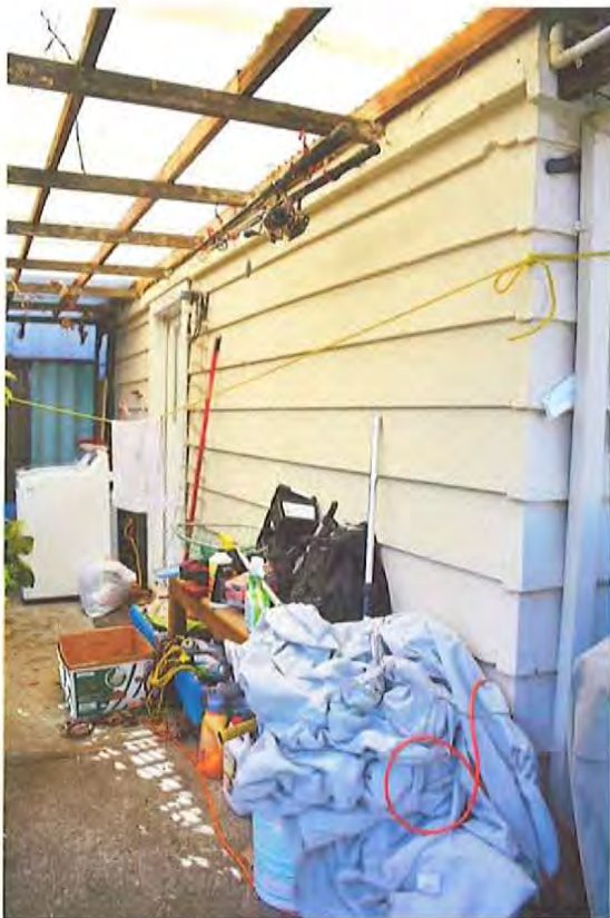
Secondary Dwelling, east elevation, facing southwest.
