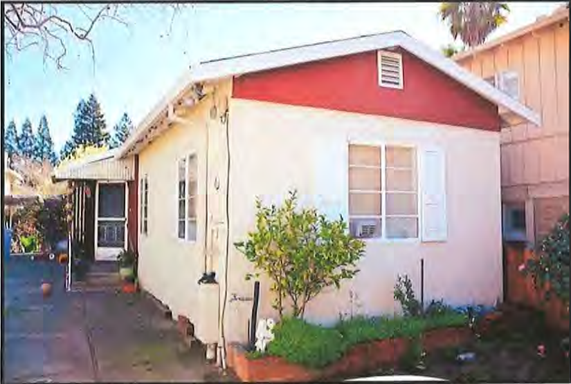
Figure 4: Secondary Dwelling, partial north and east elevations, facing southeast.
