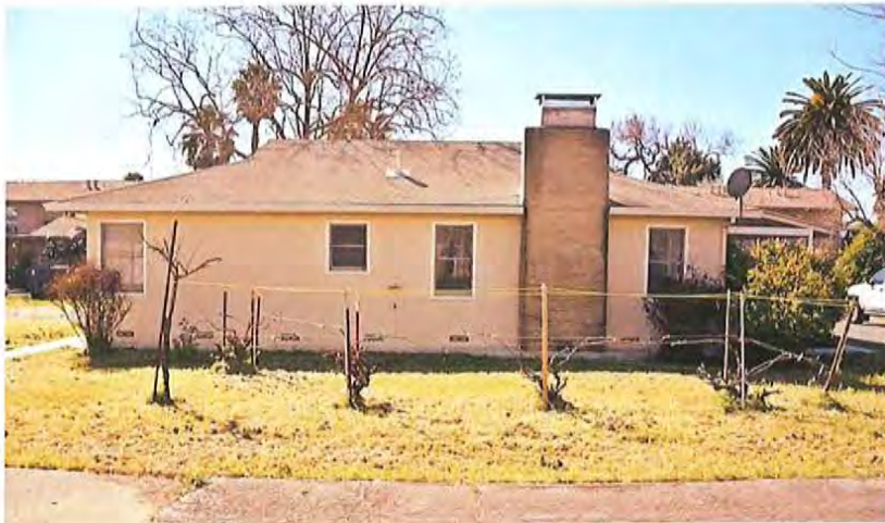
Main House, north elevation, facing south.
