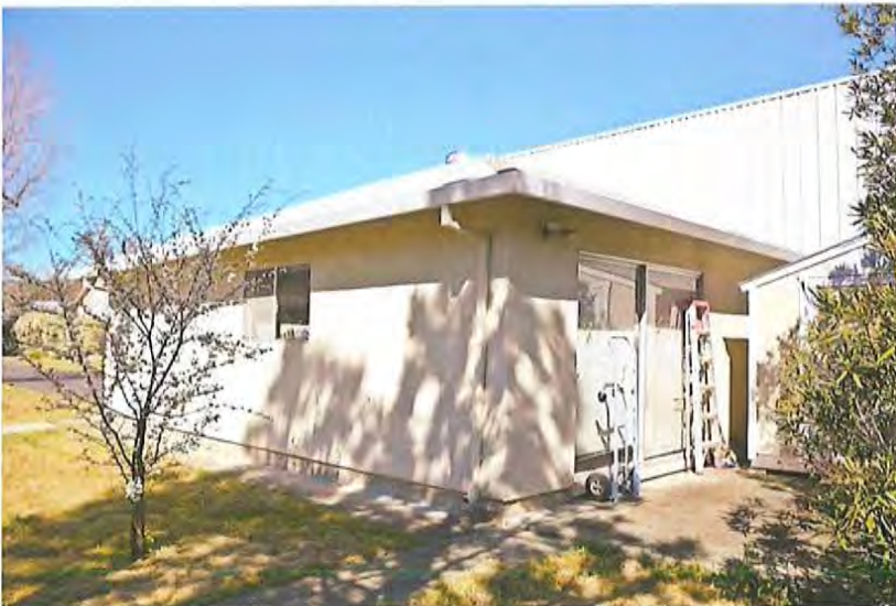
Garage, south and east elevations, facing northwest.
