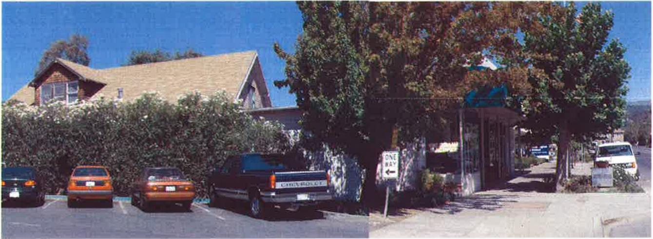
View of building looking north/ northwest. Photo shows original single family residence in rear with commercial storefront addition facing Broadway Street. Entrance to the residence in rear is through the row of Oleander bushes. The commercial storefront extends underneath the second floor of the ca. 1900 house.
