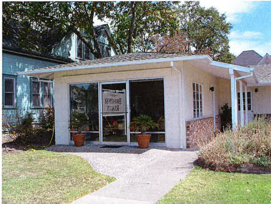
View of garage alteration. Garage door has been filled in with large plate-glass picture windows and a glazed door.
