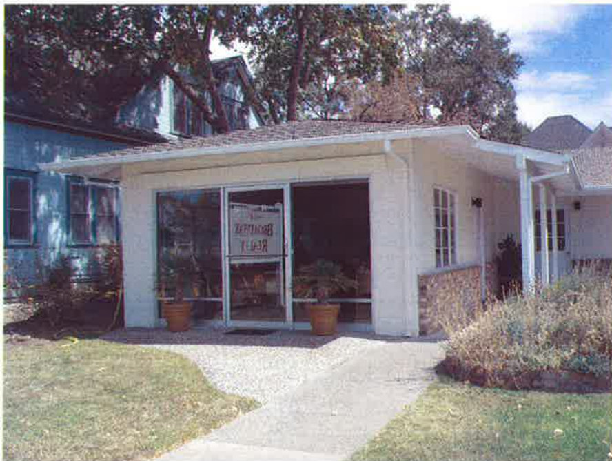
View of garage alteration. Garage door has been filled in with large plate-glass picture windows and a glazed door.
