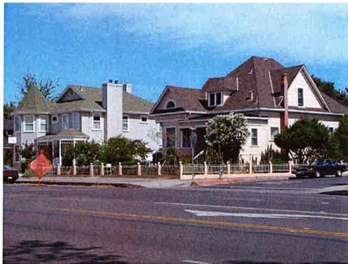
Photo showing historically compatible new construction (left) next to District Contributor built in 1904 (right). View taken looking northeast at the intersection of Broadway and France Streets.
