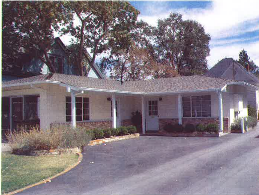
View of building looking west. Details of Ranch style include its horizontal layout, covered porch, and cross-buck door.
