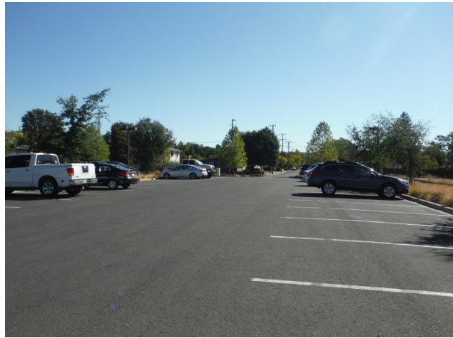
Photo 4: Typical view of the asphalt parking lot area, located on the north end of the subject parcel.
