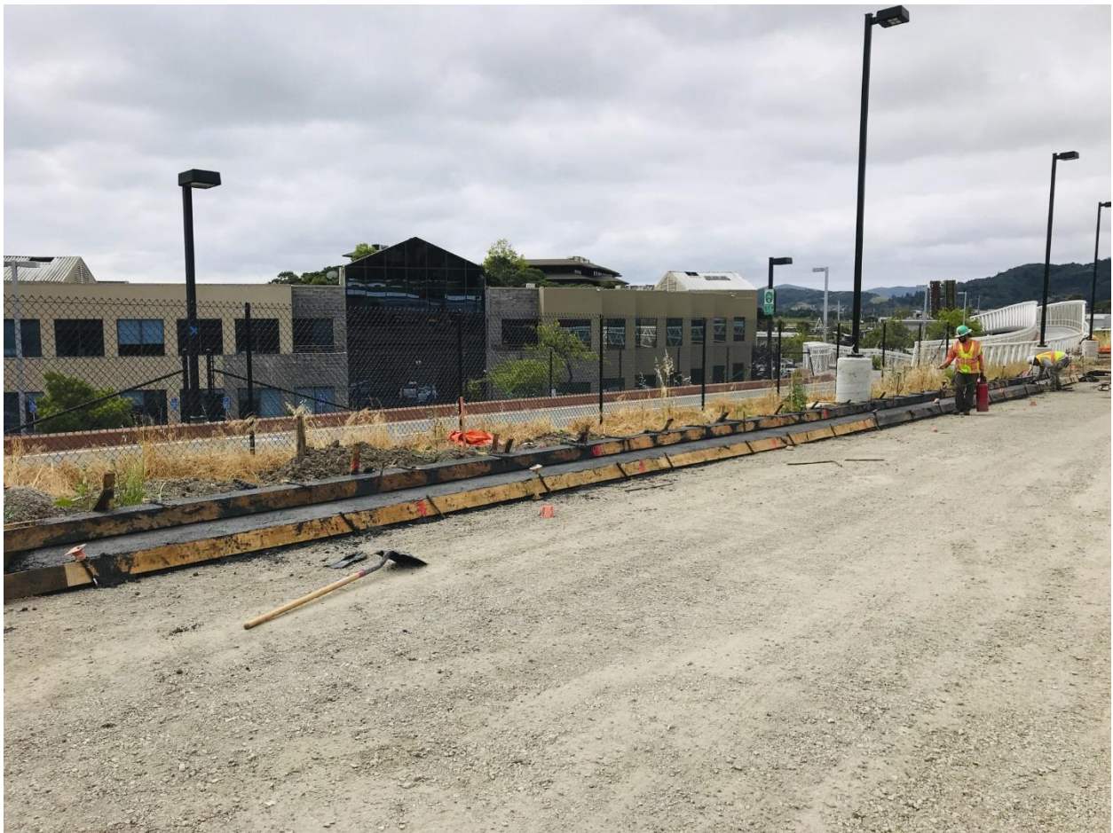
Larkspur Station- Curb and Gutter Construction at the Parking lot
