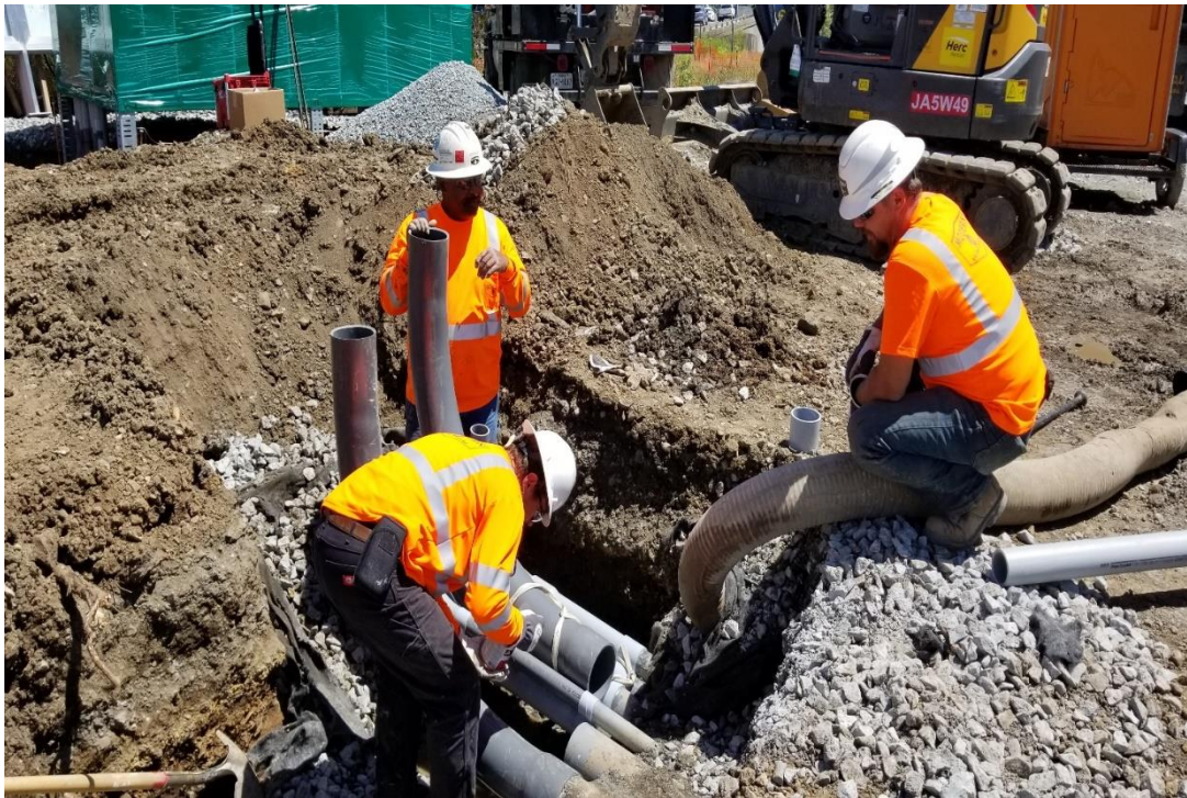
Conduit installation at the 2 nd Street
