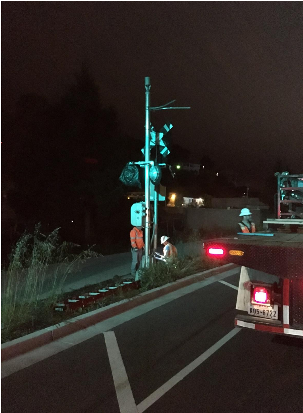
Installation of vehicle gate at Andersen Drive
