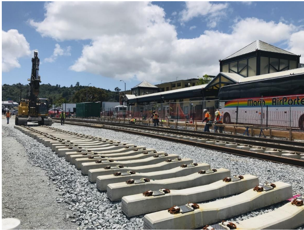
Track construction in the Bettini Transit Center
