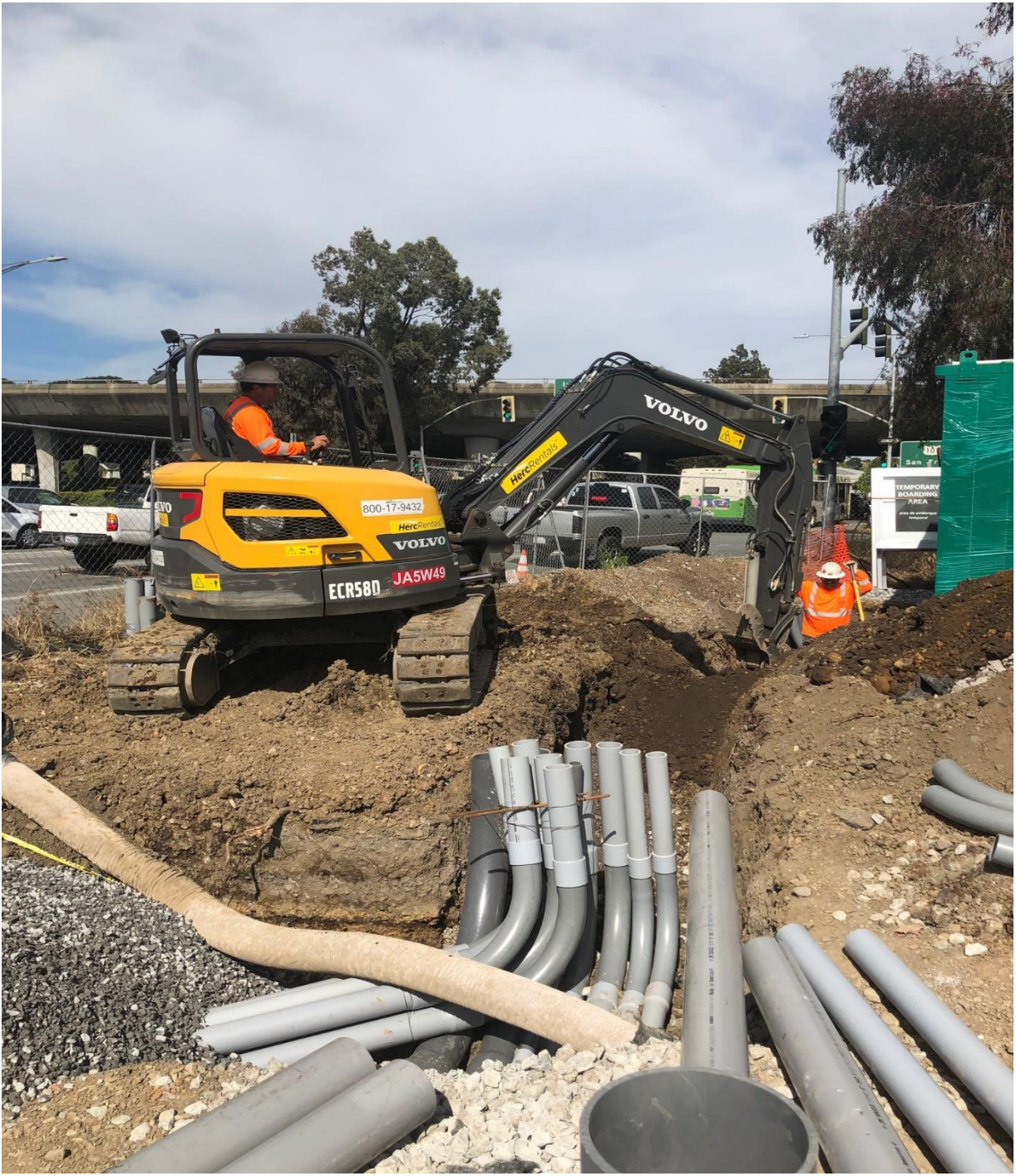
Signal conduit installation at 2 nd Street
