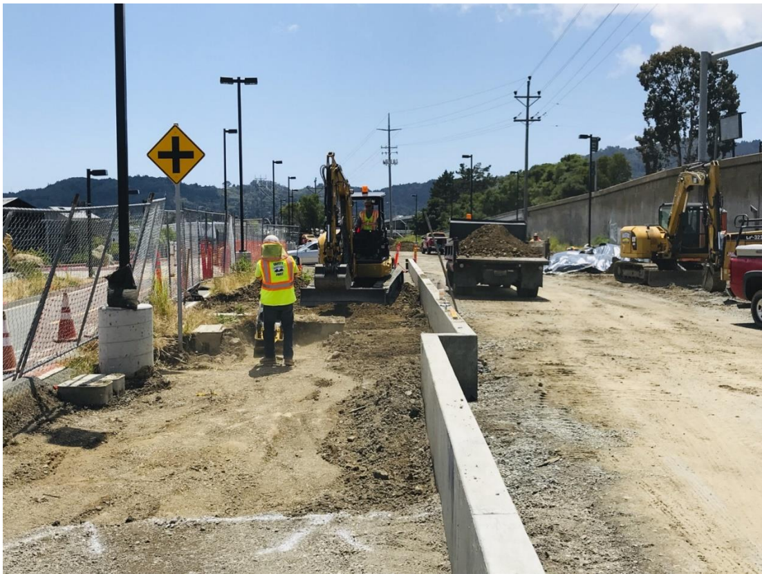
Larkspur Station- Ramp Construction
