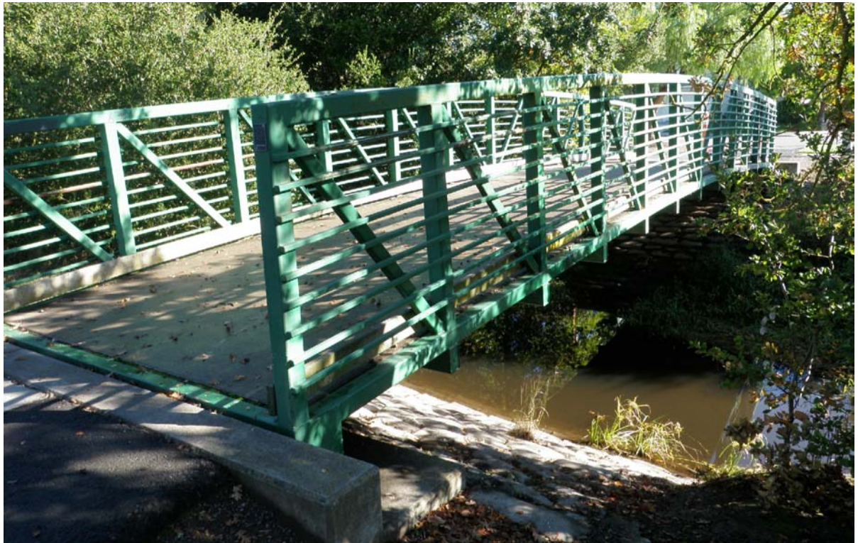
Existing Pedestrian & Bicycle Bridge at Todd Avenue
