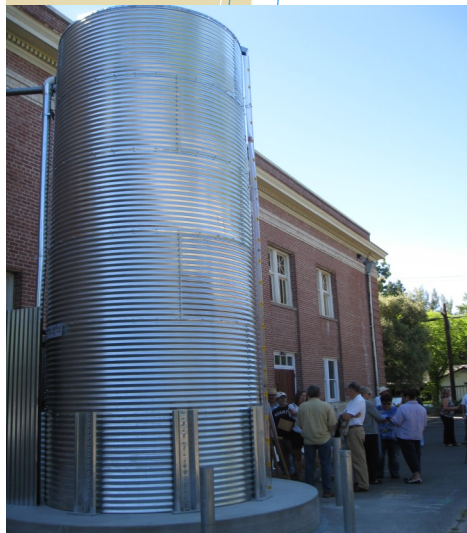
Water Tank at Sonoma Community Center
