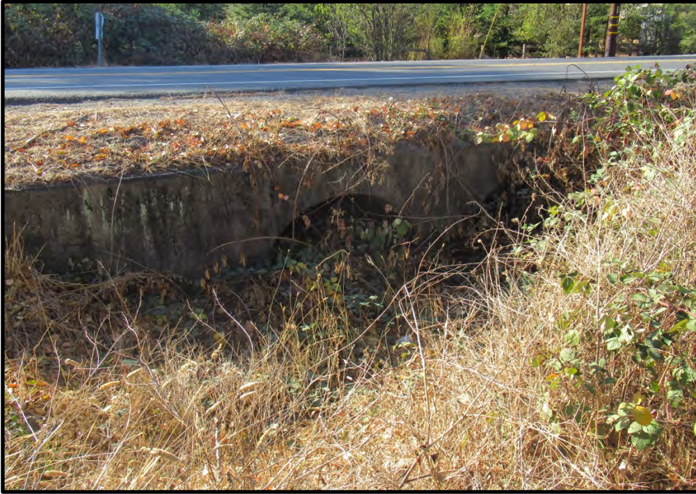
Dual culverts under Napa Road, just south of the south edge of the site, looking southwest; 11/22/19. Historically, a creek flowed through the site into this culvert. The creek has been relocated and the culverts no longer convey creek flows.
