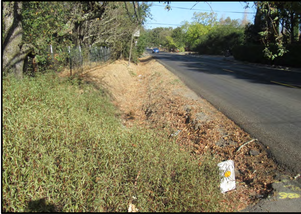
Roadside ditch just east of the east edge of the site, looking north along 5th Street from the entry of the site along the east edge; 11/22/19.
