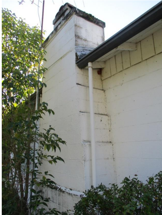
Photo showing the concrete block chimney along the east elevation.
