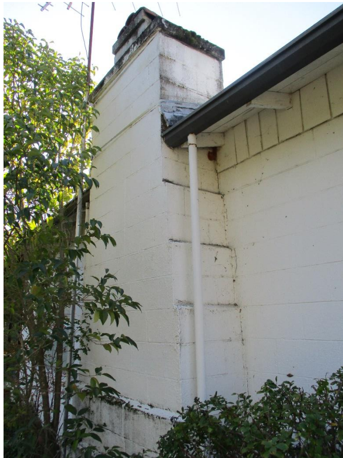
Figure 19. Photo showing the concrete block chimney along the east elevation.
