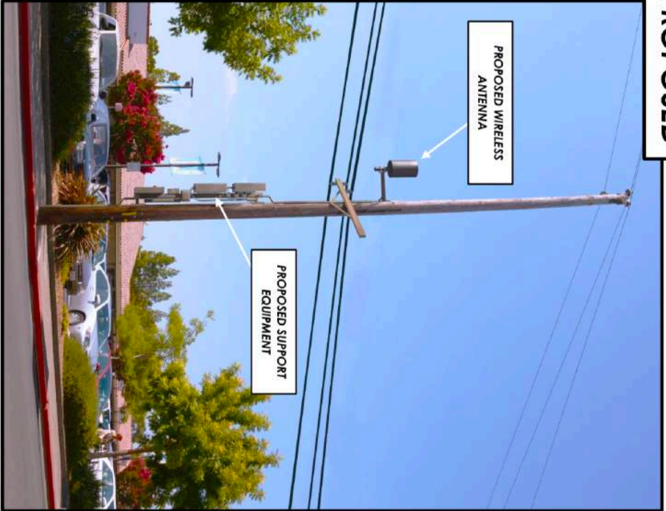
Comparison Photo of Proposed Equipment Planned Placement on Pole as compared to Removal of the RRU's and placed underground utility vault below the sidewalk.
