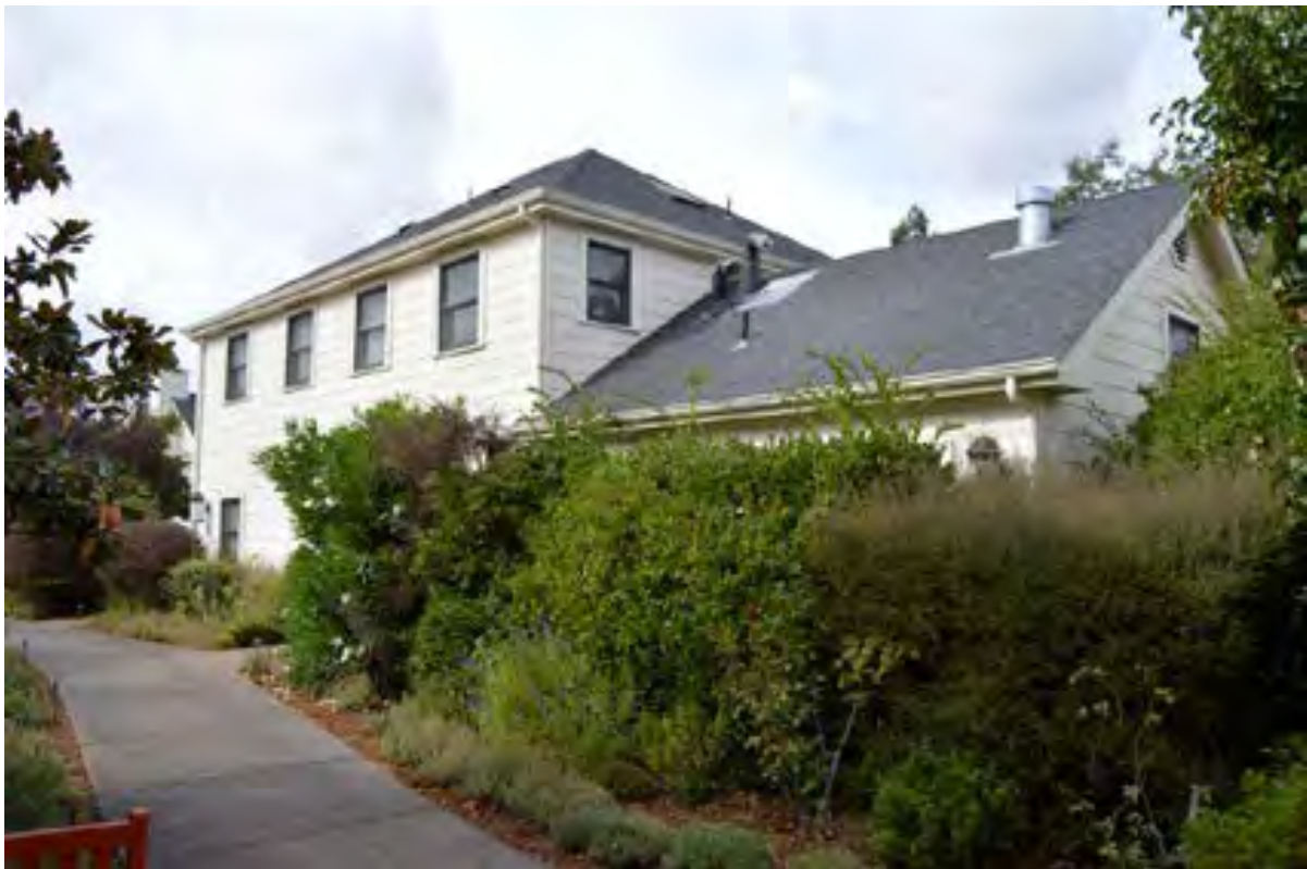
Photograph 1. View of spa and fitness building (identified as Building L in Figure 3), looking west
