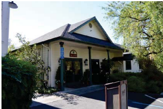
Figure 2: North facade of former garage. Looking southwest.
