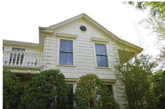
Figure 7: West gabled volume at primary (north) façade with stacked porch of west façade visible. Looking south.
