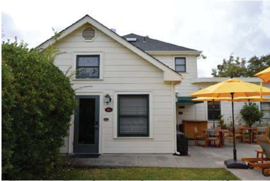
Figure 2: East facade of one-and-a-half story, gable-roofed volume. Looking west.
