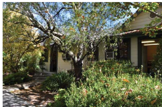
Figure 9: West facade of former garage building. Looking northeast.
