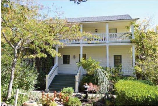
Figure 18: West façade with stacked porch. Wood balustrade at each story and wood stairs leading from ground level to first story. Looking east.
