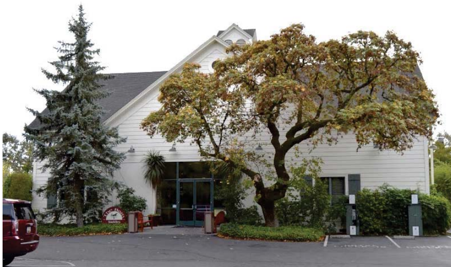
Figure 3: South gable end and south façade of converted barn. Looking south from west parking lot.
