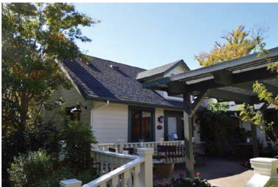
Figure 4: East facade of garage building with outdoor deck. Looking west.
