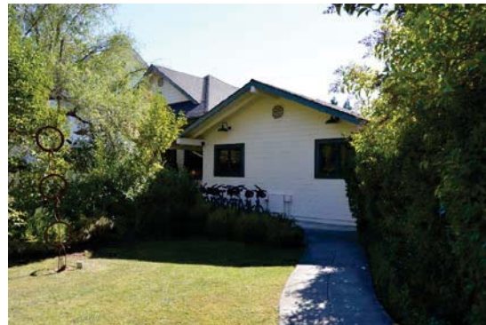
Figure 3: Gable-roofed volume original to former garage building. Looking south.
