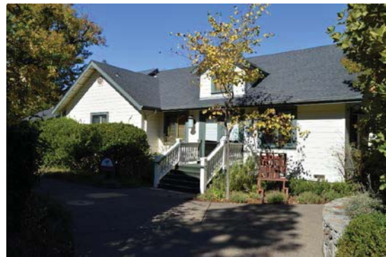
Figure 5: South facade of former garage building. Library addition added in 1999. Looking north.
