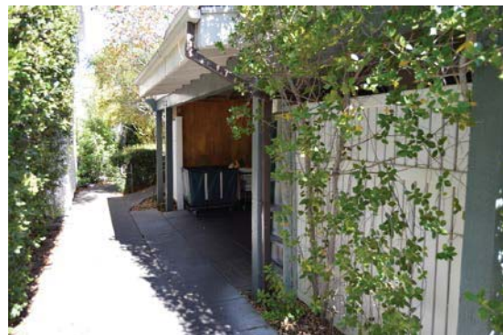
Figure 7: Original garage bay at southwest end of former garage building. Looking north.
