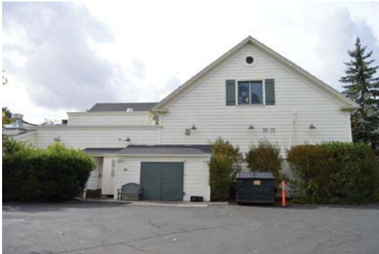
Figure 4: Northernmost portions of converted barn's east facade. Looking west from west parking lot.
