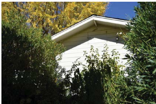
Figure 2: South gable-end with wood fascia and soffit. Looking north.
