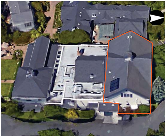
Figure 1: 3-D aerial imagery of former barn building. Original massing of building indicated with orange line. Source: Google Earth Pro, 2016.
