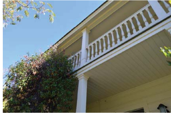
Figure 19: Balustrade at second story of porch. Looking north.
