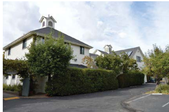
Figure 7: View from south end of west parking lot of barn (far-right) and additions added in 1998 and 2003. Looking northwest.
