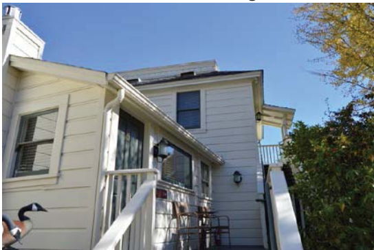
Figure 12: Rear (south) facade of hyphen connecting main residential volume and converted larder building.
