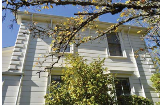
Figure 9: West façade at main residential volume. Rusticated quoins pictured at north and south end of façade. Looking west.
