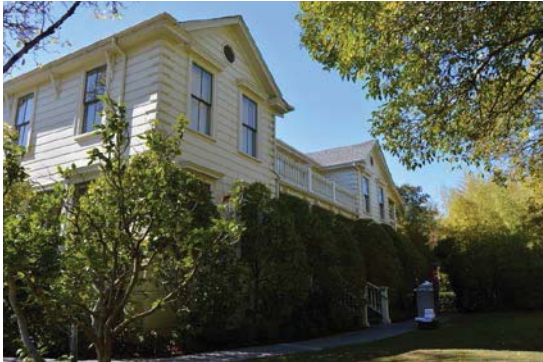
Figure 2: Primary (north) façade viewed from lawn to north of Burris House. Looking west.
