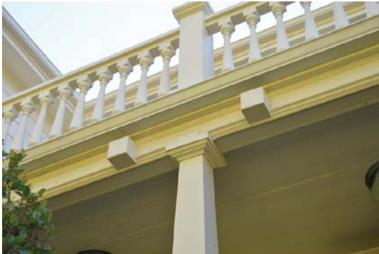
Figure 4: Tapered, square columns and wood balustrade at primary façade. Looking south.
