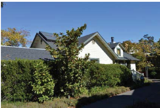
Figure 6: Library addition viewed from adjacent path. Looking northwest.
