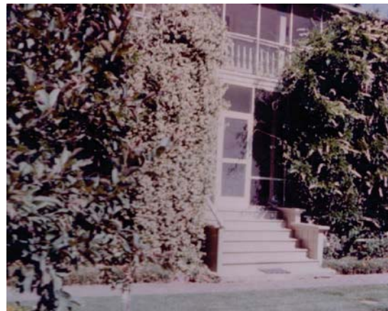
Figure 29: Wood steps leading to first story porch along west facade of Burris House, ca. 1950s. Courtesy MacArthur Place Hotel.
