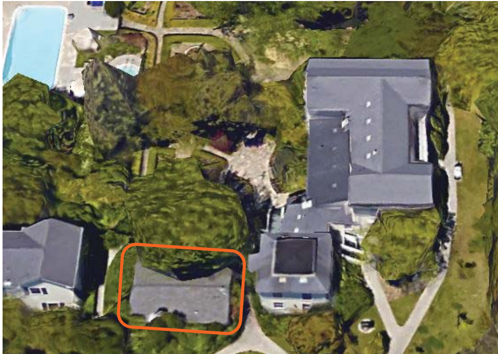
Figure 1: 3-D aerial imagery of caretaker's cottage and surrounding buildings. Dense tree coverage surrounds the cottage. Oriented to west. Source: Google Earth Pro, 2016.
