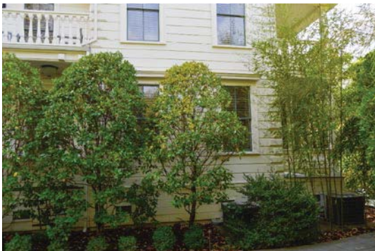
Figure 6: Fenestration at first story of outermost bays at primary (north) façade. Looking south.
