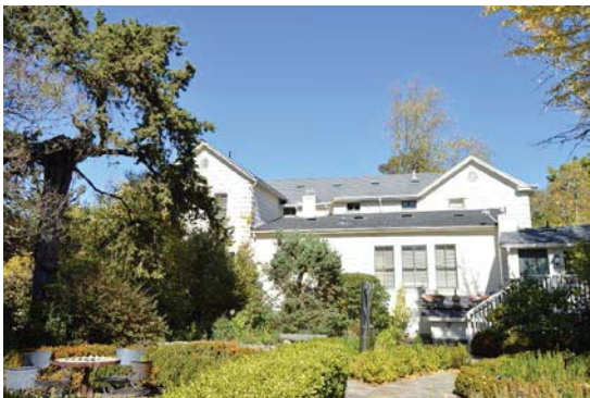
Figure 15: Rear (south) facade of Burris House viewed from central garden. Looking north.
