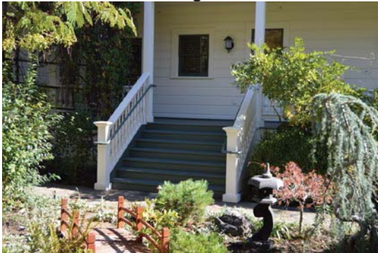
Figure 20: Wood stairs and molded wood hand rails with turned balusters. Looking east.
