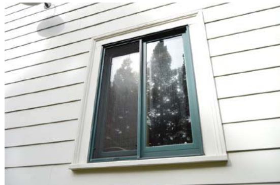
Figure 9: Typical sliding, aluminum casement window located at several locations around barn.
