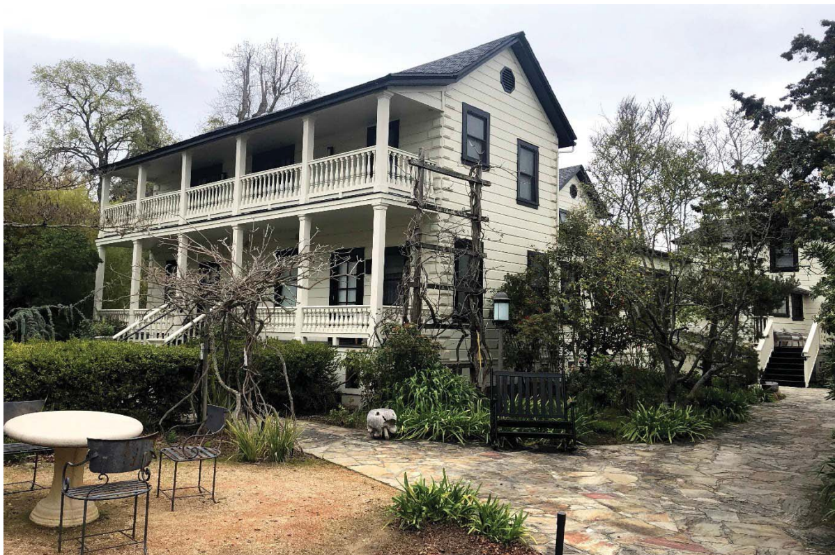
Photograph 2. View of the existing Burris House (Building T), looking southeast
