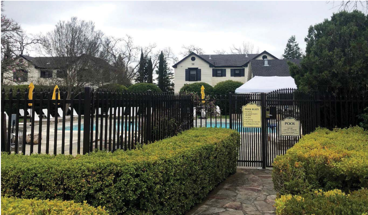
Photograph 3. View of the existing pool, looking south
