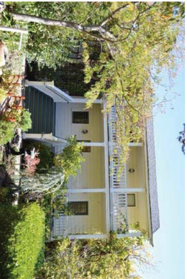
Figure 20: West façade with stacked porch. Wood balustrade at each story and wood stairs leading from ground level to first story. Looking east.
