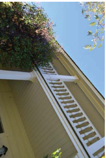
Figure 21: Balustrade at second story of porch. Looking north.
