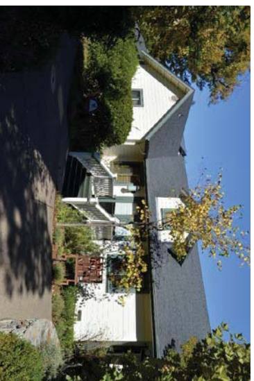
Figure 46: South facade of former garage building. Library addition added in 1999. Looking north.
