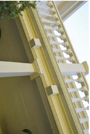
Figure 6: Tapered, square columns and wood balustrade at primary facade. Looking south.
