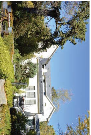
Figure 17: Rear (south) facade of Burris House viewed from central garden. Looking north.
