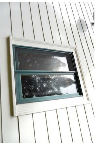
Figure 32: Typical siding, aluminum casement window located at several locations around barn.
