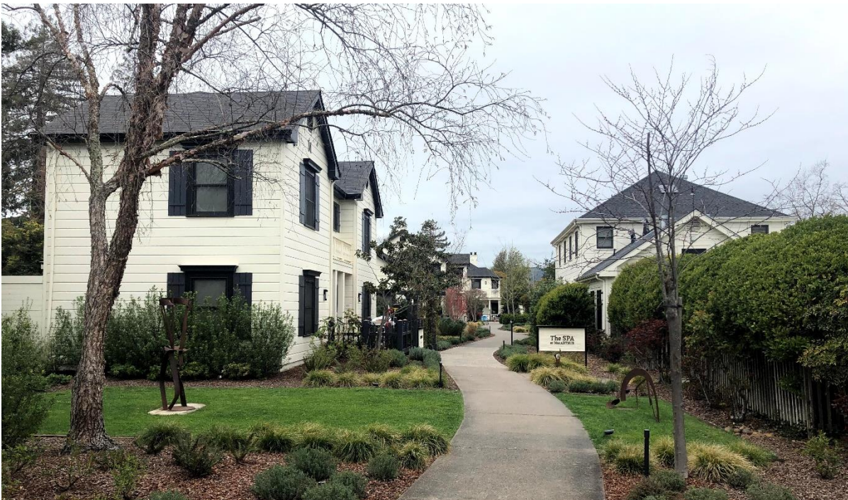
Photograph 4. View of existing Buildings N, M, L, and K, looking west
