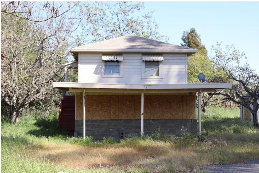
Figure 18. West elevation, facing east.
