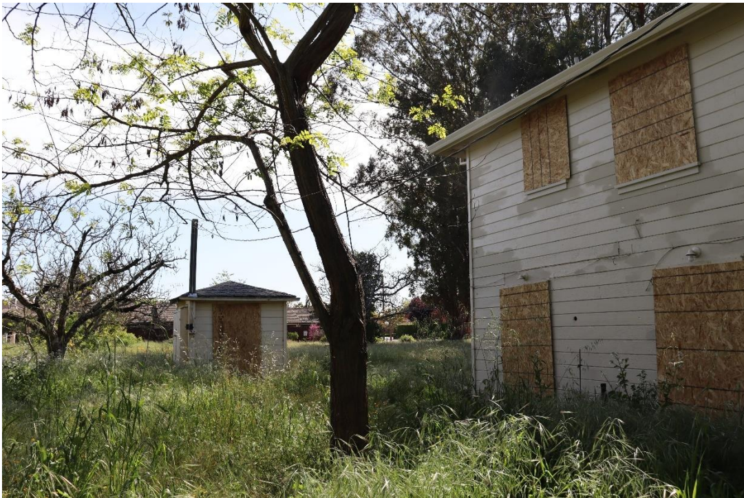
Figure 26. Photo showing the ca. 1940 auxiliary building, adjacent and south of the ca. 1940 house.
