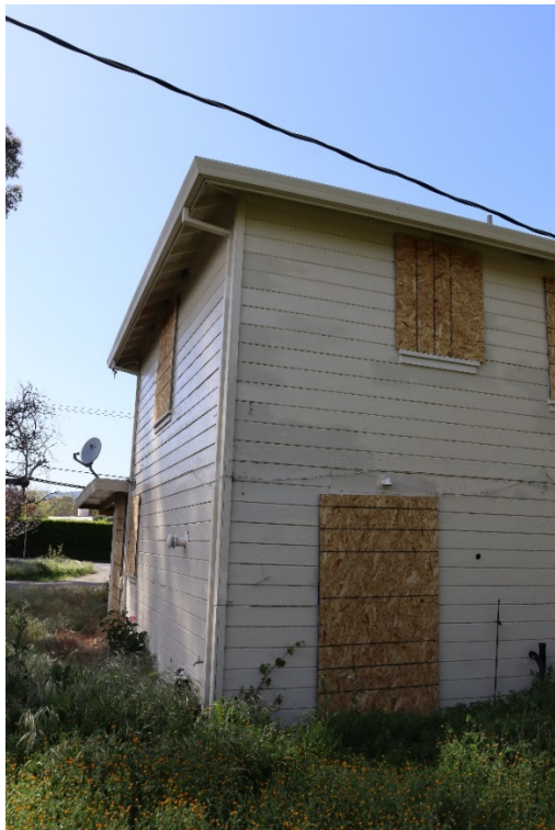
Figure 7. Photo showing the southeast corner of the east elevation, facing west.
