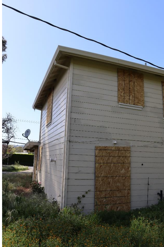
Figure 23. Photo showing the southeast corner of the east elevation, facing west.
