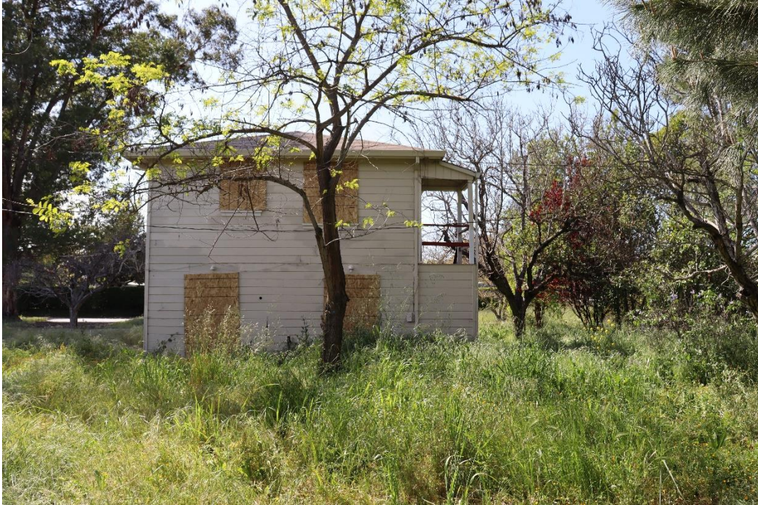
Figure 22. East elevation, facing west.
