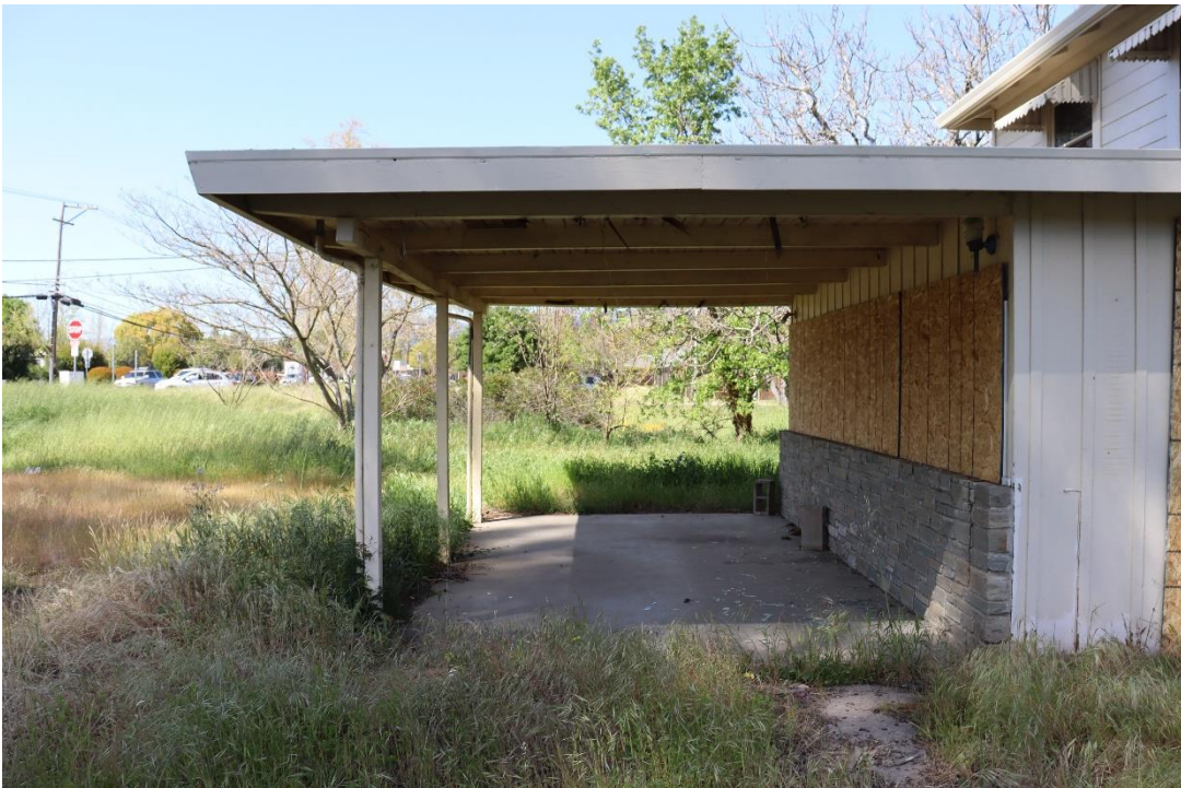
Figure 21. Photo showing the south elevation of the 1956 addition, facing north.
