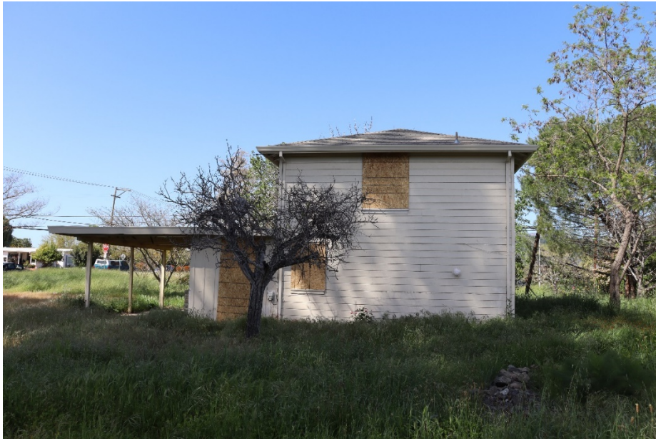
Figure 4. South elevation, facing north.
