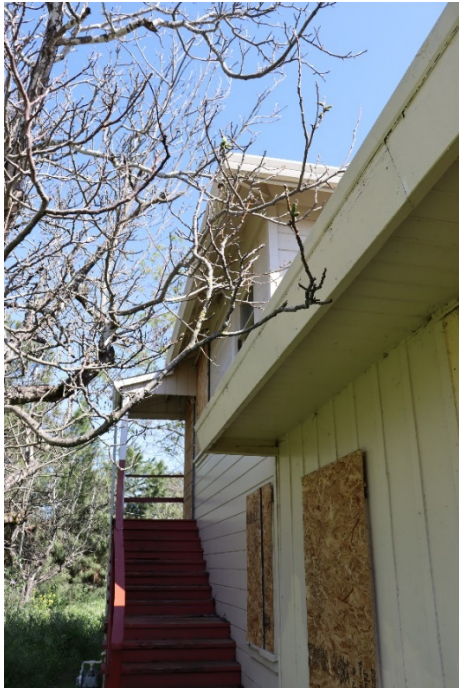
Figure 8. North elevation showing the exterior second story stairs, facing west.
