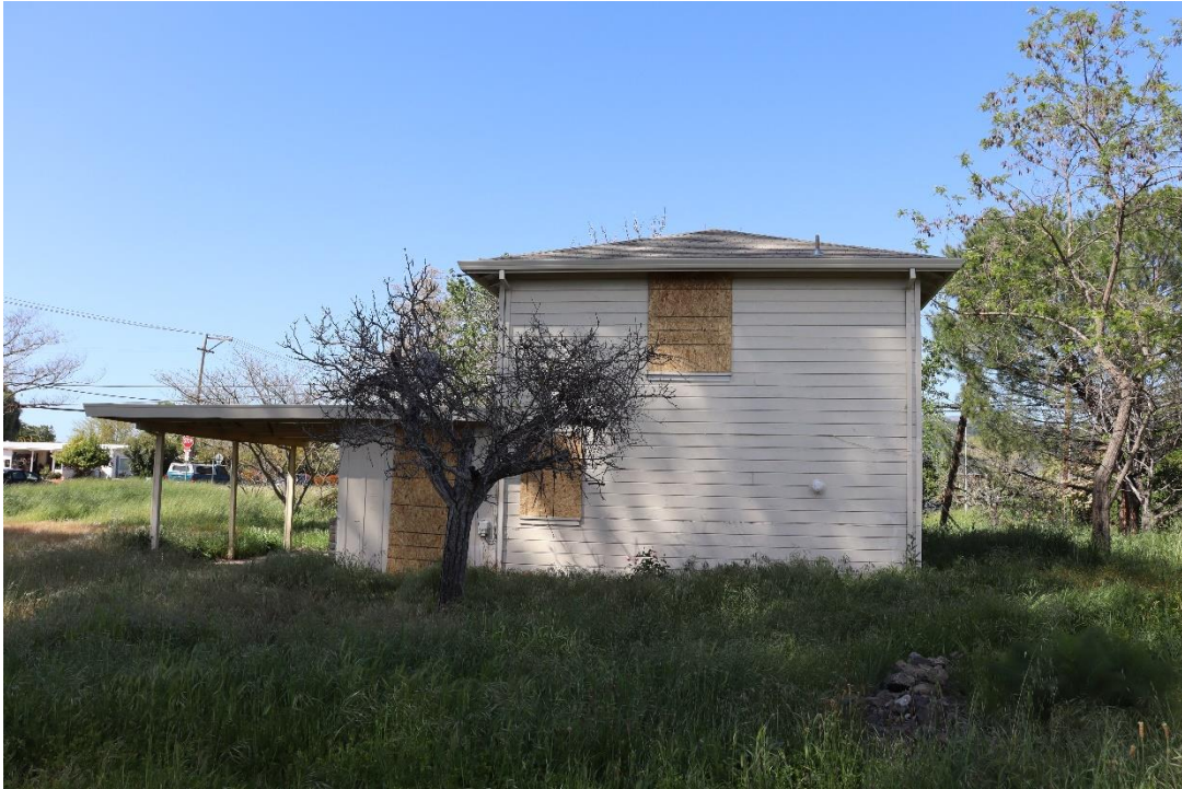
Figure 20. South elevation, facing north.
