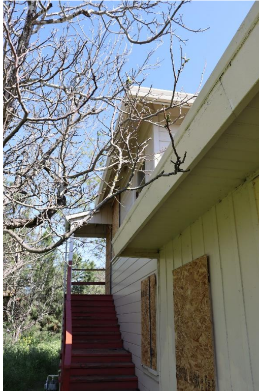
Figure 24. North elevation showing the exterior second story stairs, facing west.
