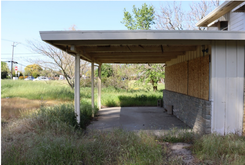
Figure 5. Photo showing the south elevation of the 1956 addition, facing north.
