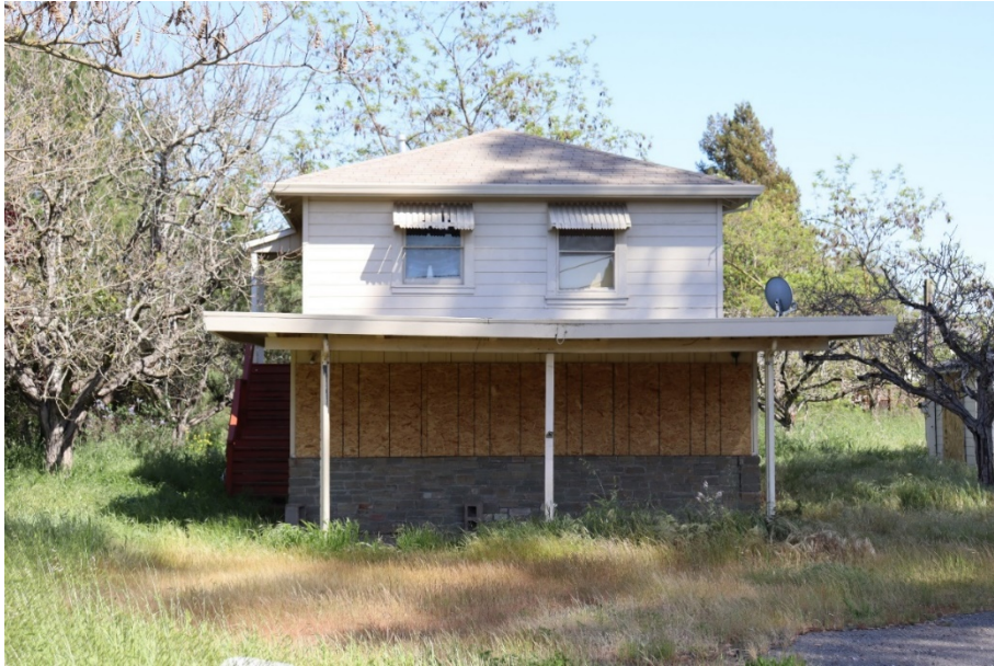
Figure 2. West elevation, facing east.
