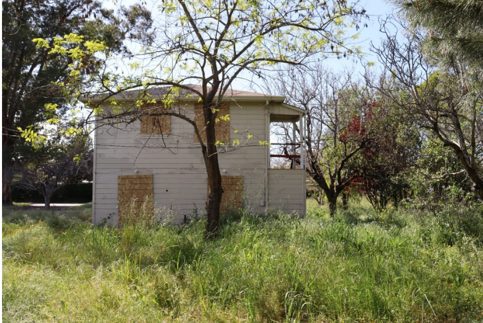
Figure 6. East elevation, facing west.
