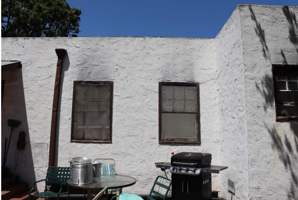
Figure 10. East elevation, facing north.
