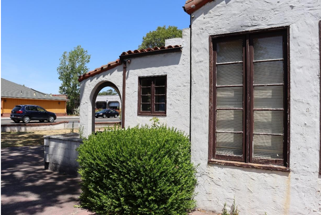
Figure 27. South elevation, facing northwest.
