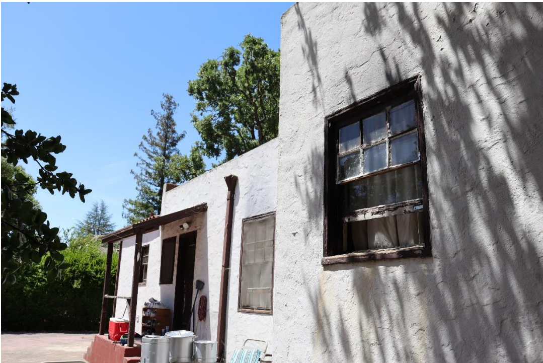
Figure 31. East elevation, facing south.
