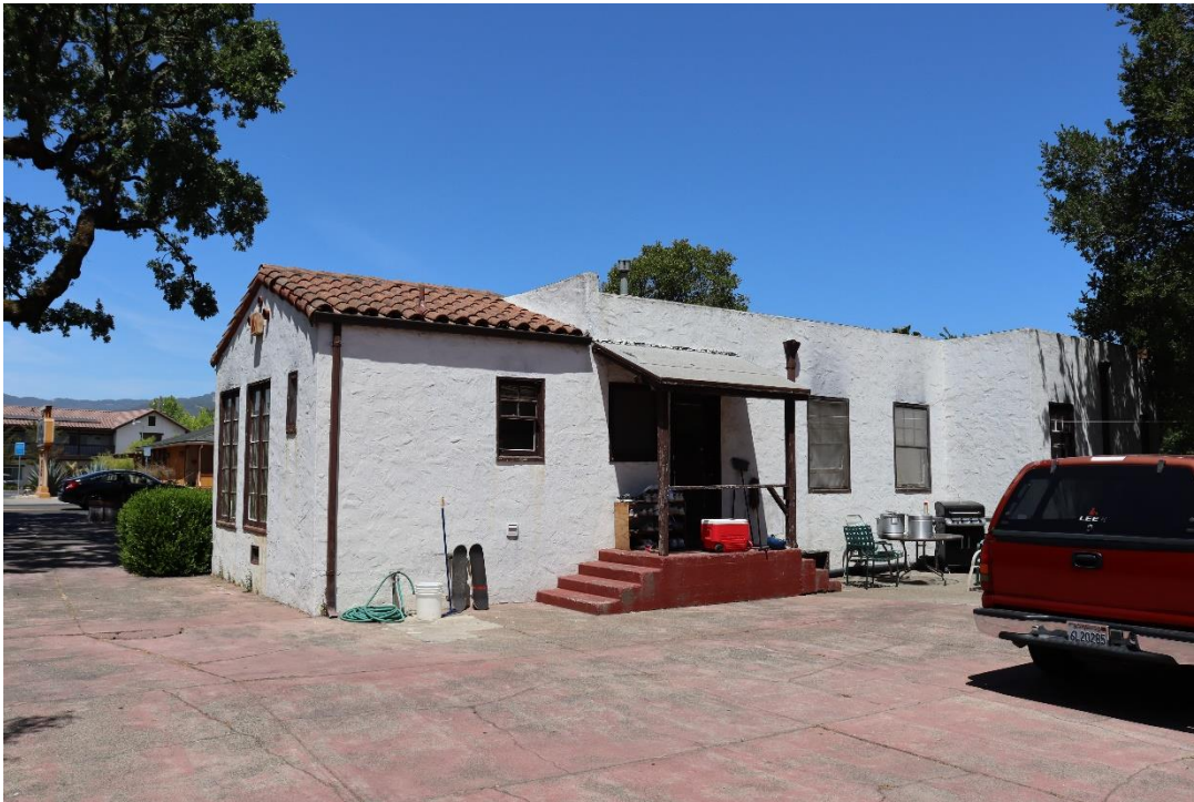
Figure 29. East elevation, facing north.
