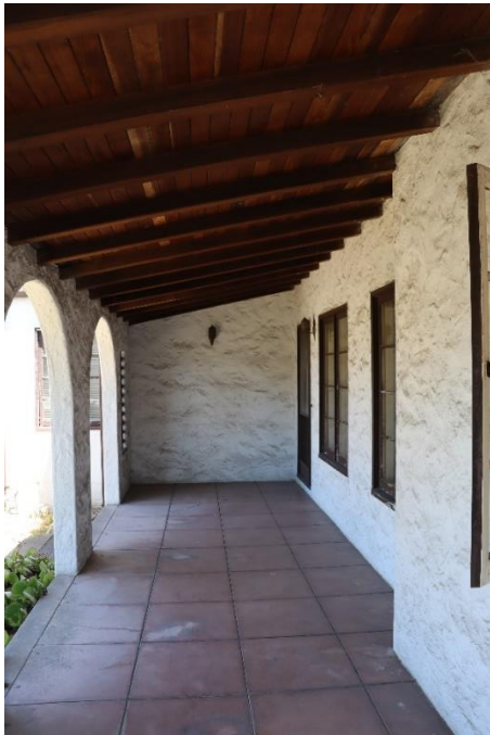
Figure 3. Photo showing the wooden beams and wood ceiling.
