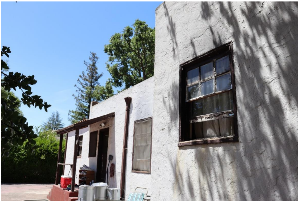
Figure 11. East elevation, facing south.
