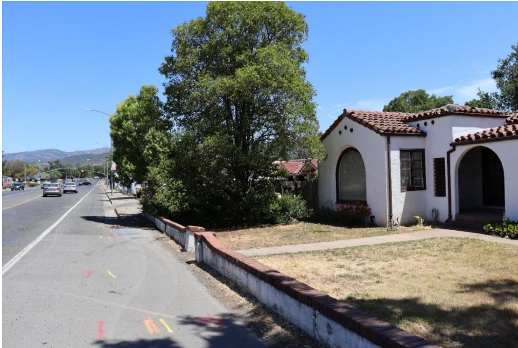
Figure 13. Photo showing the low garden wall along the western boundary of the property, facing north.
