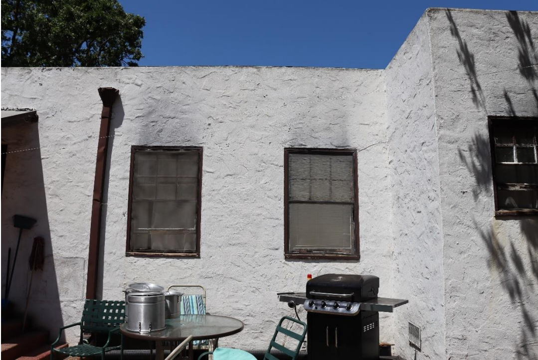
Figure 30. East elevation, facing north.
