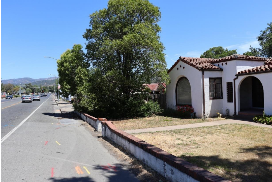
Figure 33. Photo showing the low garden wall along the western boundary of the Property, facing north.
