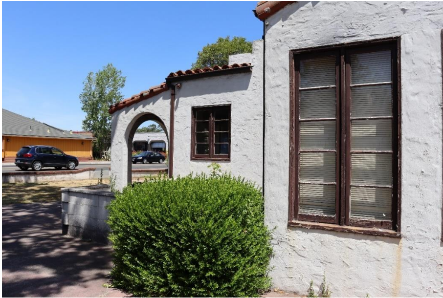
Figure 7. South elevation, facing northwest.
