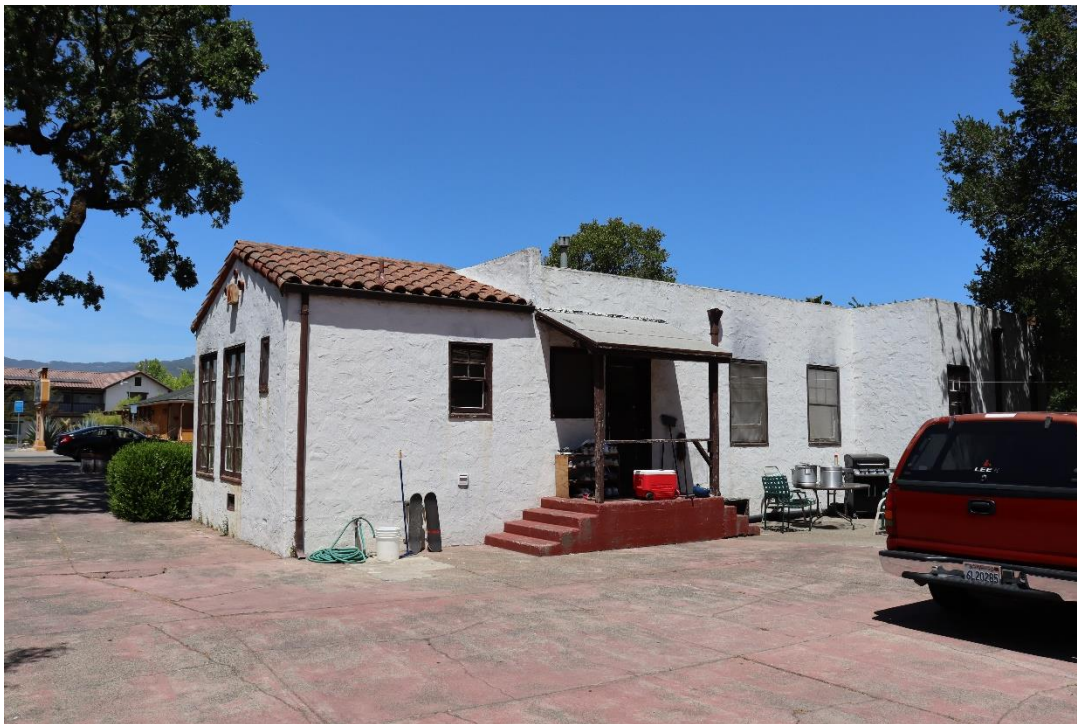
Figure 9. East elevation, facing north.
