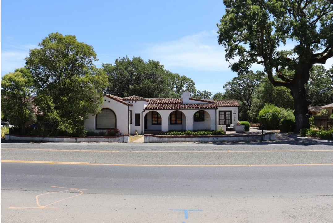
Figure 20. West elevation, facing east.
