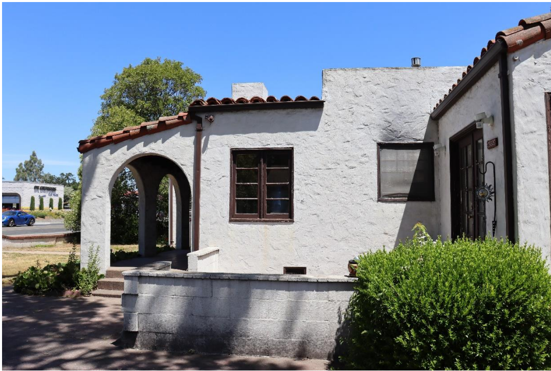
Figure 6. Photo showing a portion of the south elevation, facing north.
