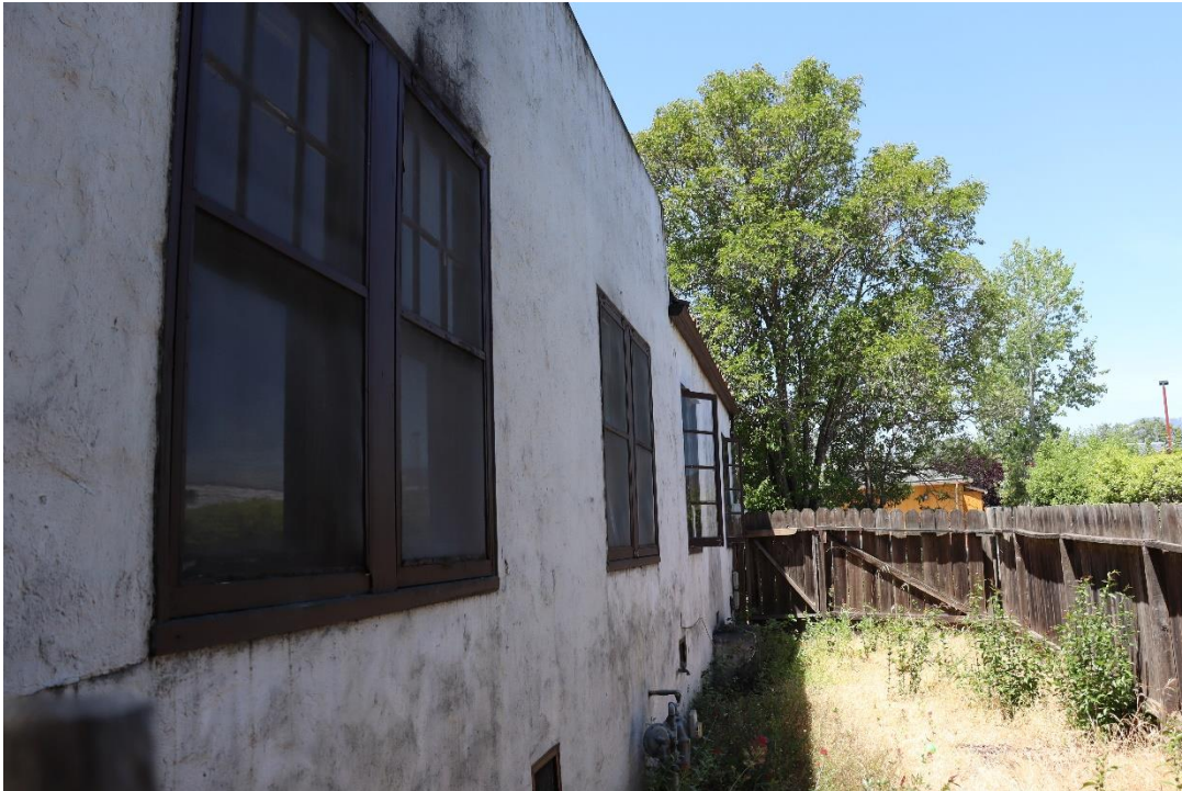
Figure 32. North elevation, facing west.
