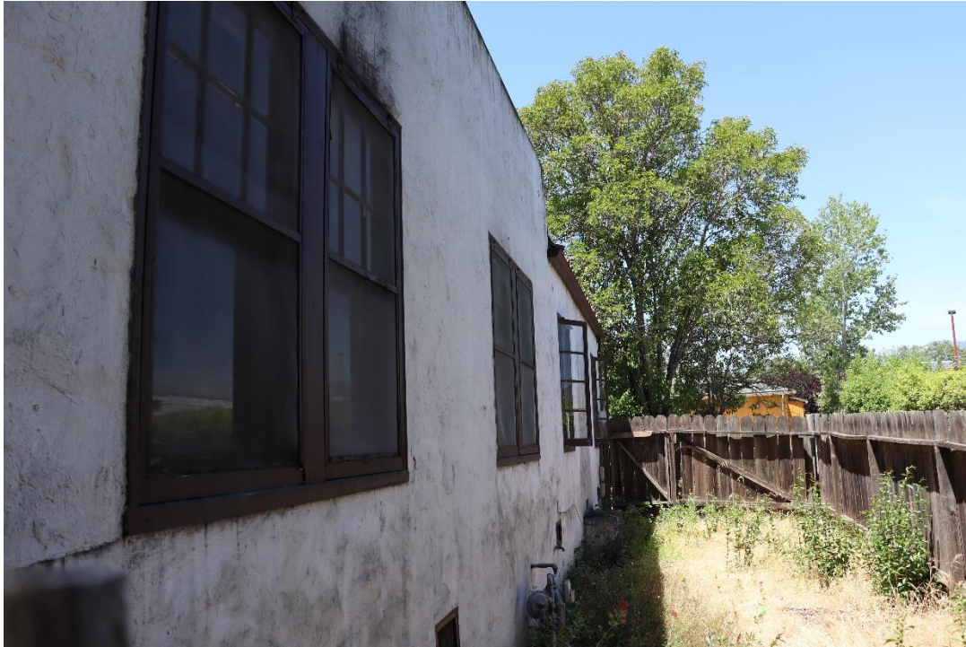
Figure 12. North elevation, facing west.
