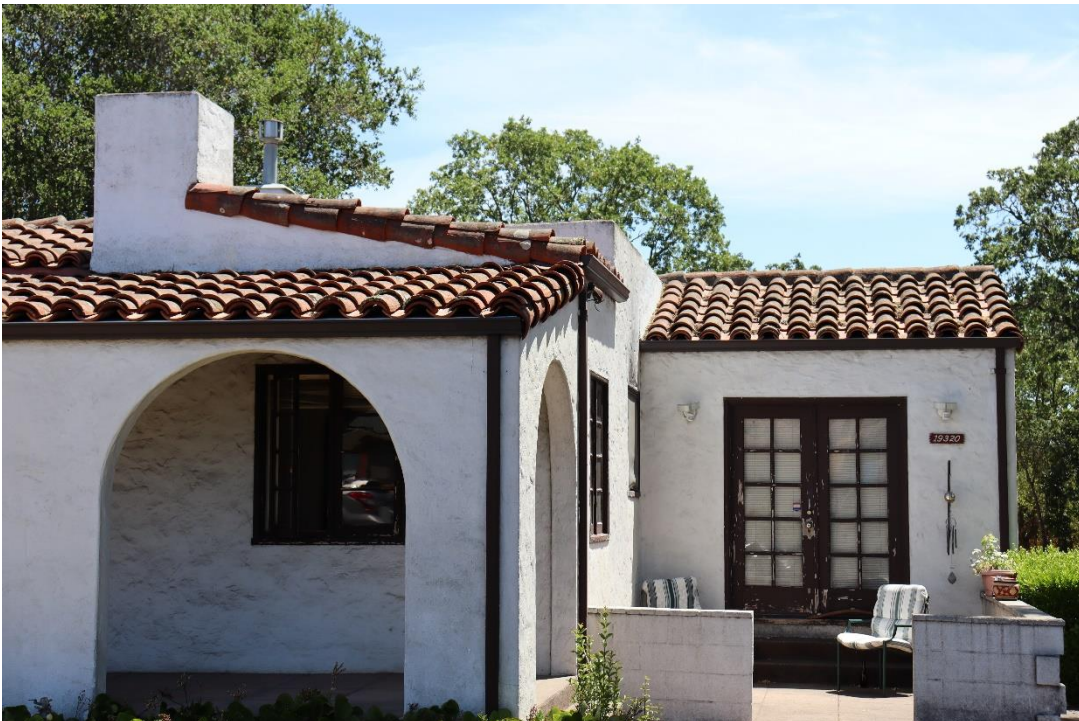
Figure 25. Photo showing the open courtyard along the primary façade.
