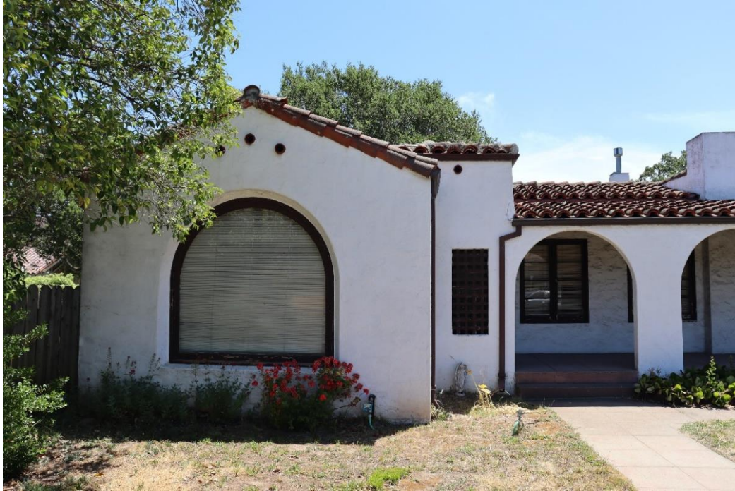
Figure 4. Photo showing the fixed arched picture window along the projecting gable wing, facing east.
