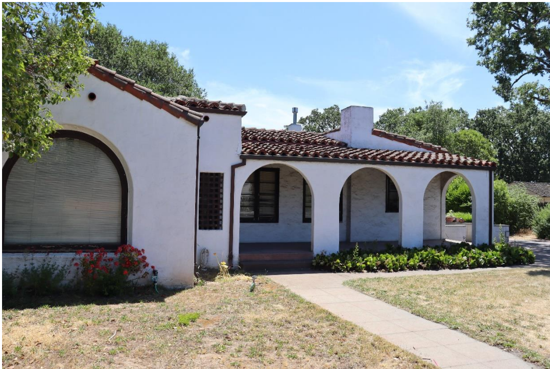
Figure 1. West elevation, facing east.
