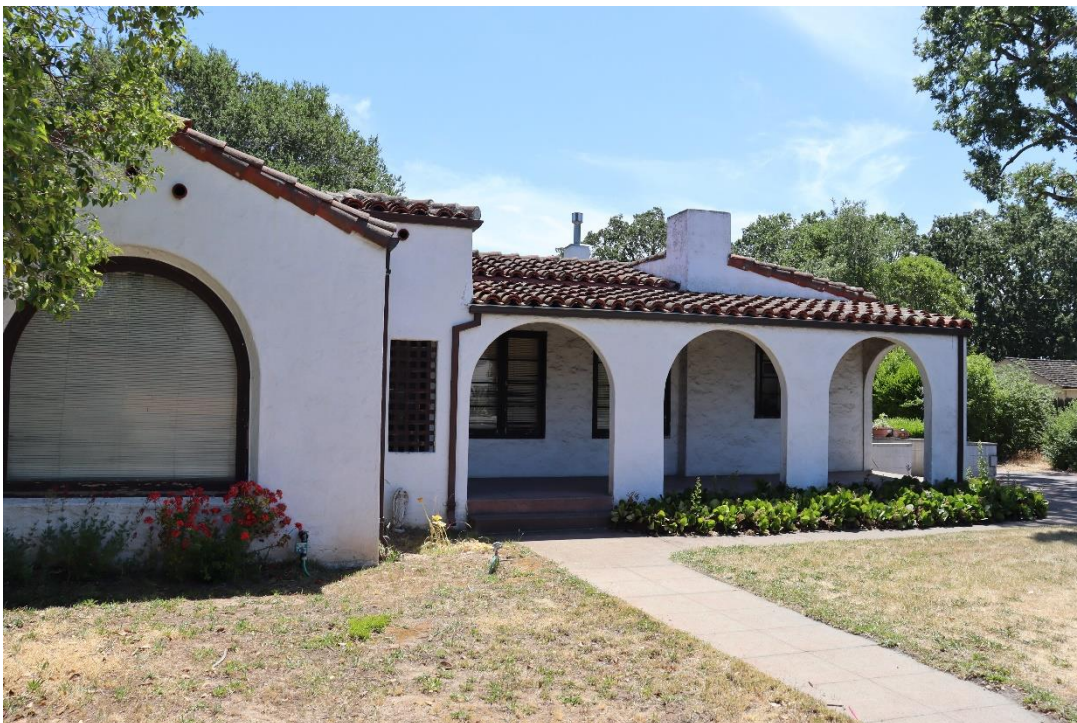
Figure 21. West elevation, facing east.
