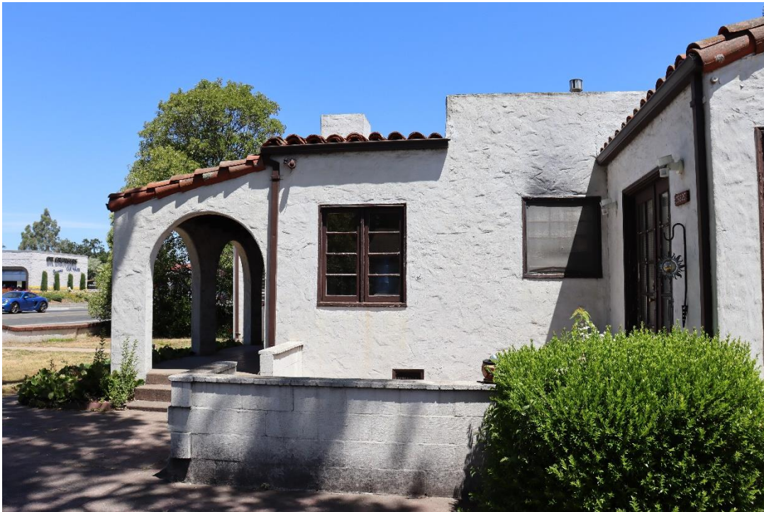
Figure 26. Photo showing a portion of the south elevation, facing north.
