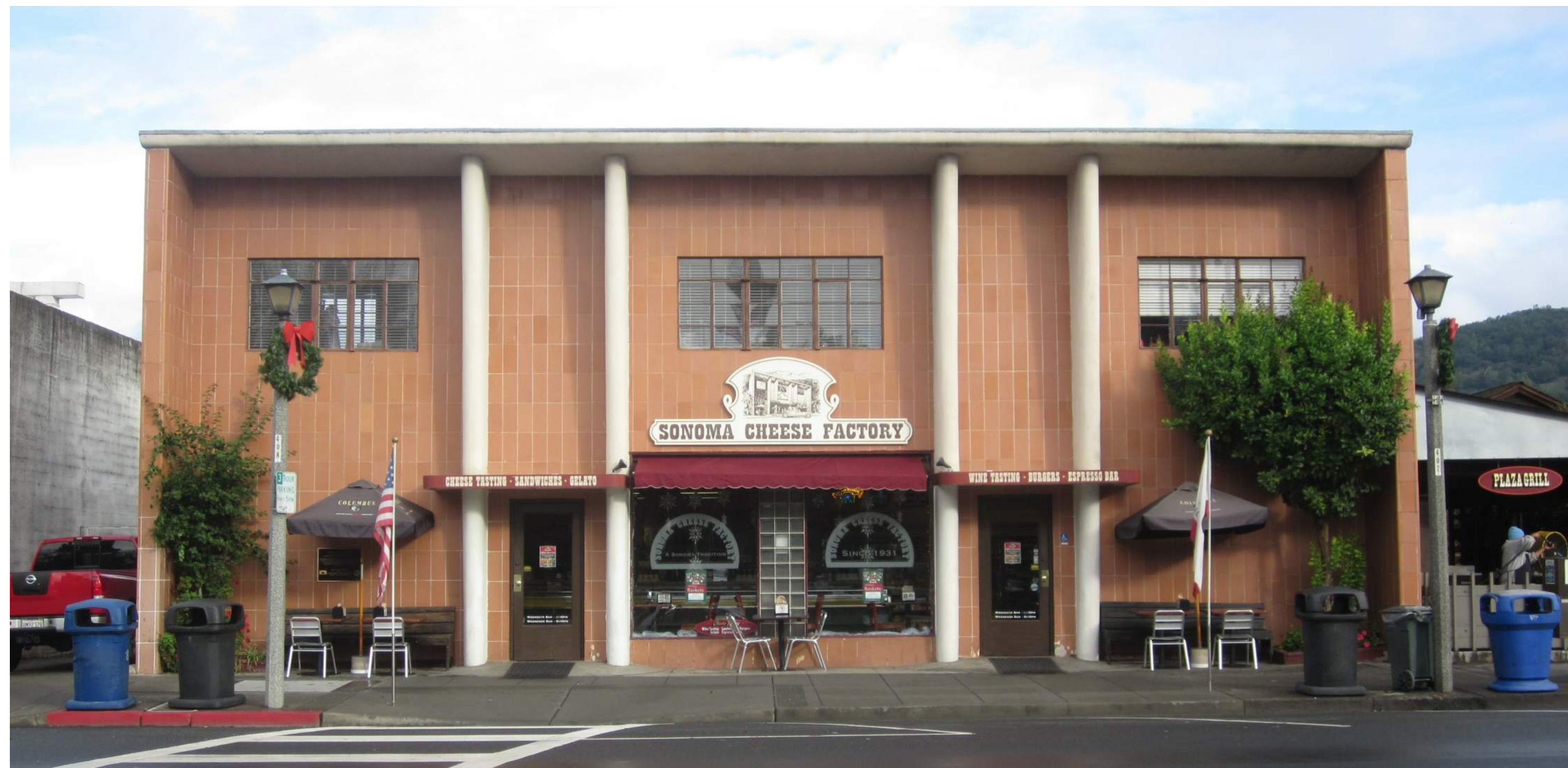
SOUTH ELEVATION - FROM HISTORIC SONOMA PLAZA
