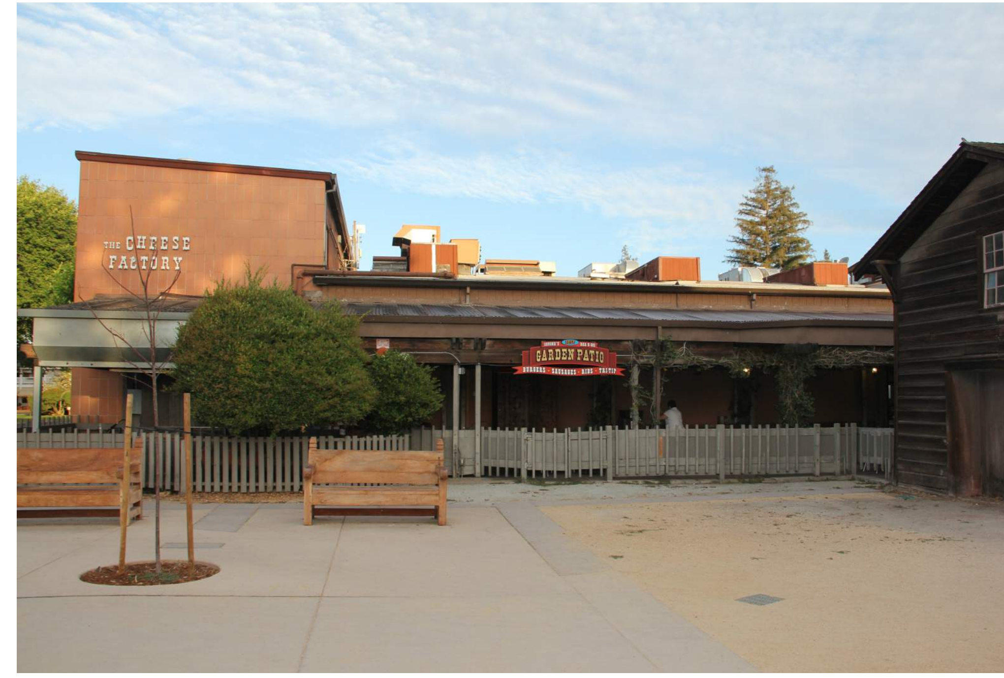
EAST ELEVATION (PARTIAL) - FROM STATE HISTORIC PARK
