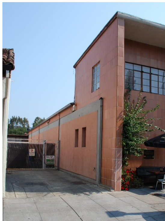
Figure 4. West façade of the Sonoma Cheese Factory building, view northeast. Photo by Page & Turnbull, 2014.
