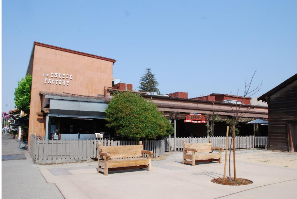
Figure 5. East façade of the Sonoma Cheese Factory building, view northwest. Photo by Page & Turnbull, 2014.
