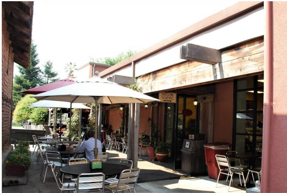
Figure 8. Relationship of adjacent buildings, Casa Grande Servants' Quarters building at left, non-original patio of the Sonoma Cheese Factory building at right. View southwest. Photo by Page & Turnbull, 2014.
