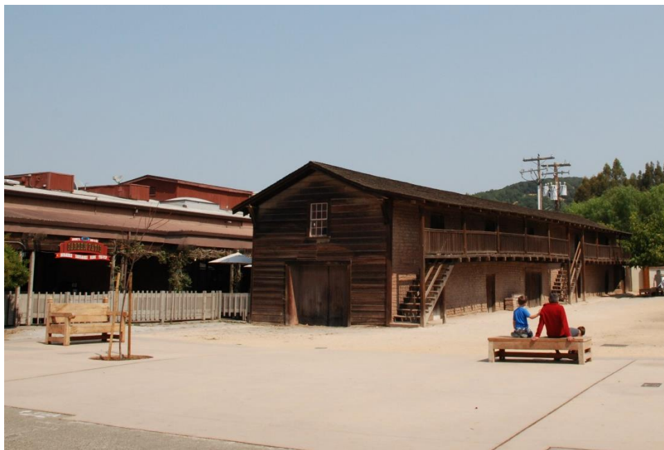
Figure 7. Casa Grande Servants' Quarters building, view northwest from W Spain Street. Photo by Page & Turnbull, 2014.
