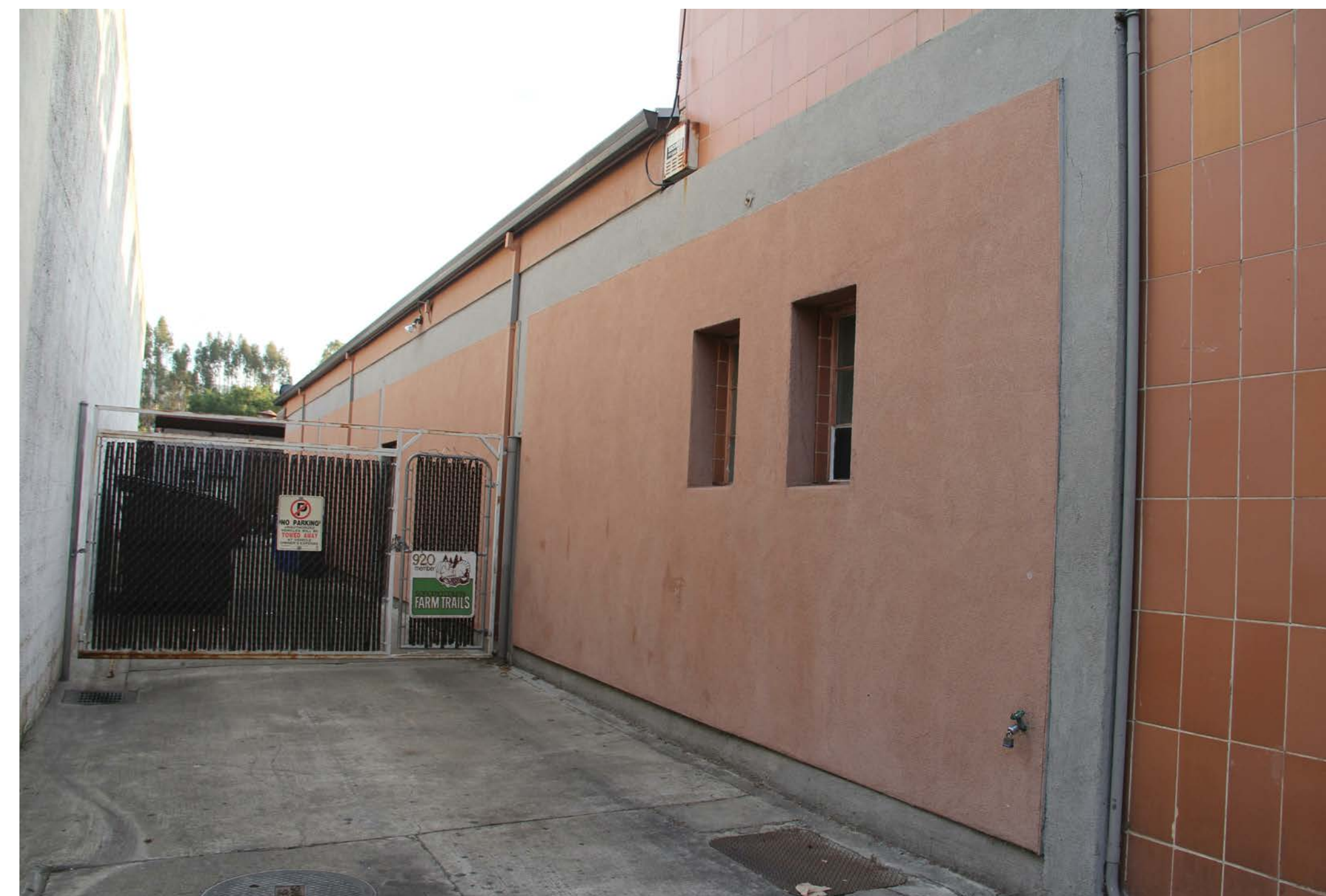
WEST ELEVATION (PARTIAL) - FROM ALLEY
