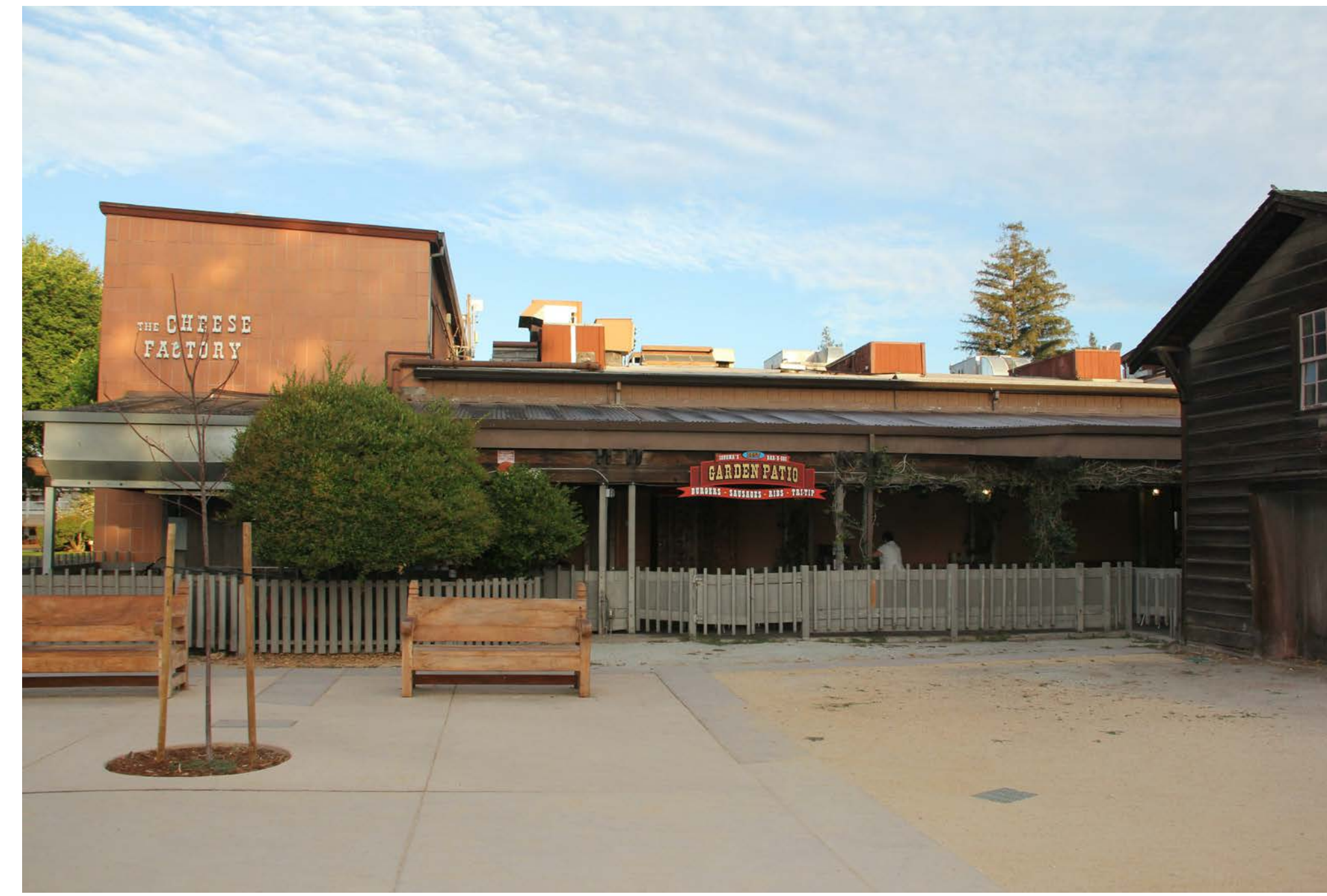
EAST ELEVATION (PARTIAL) - FROM STATE HISTORIC PARK
