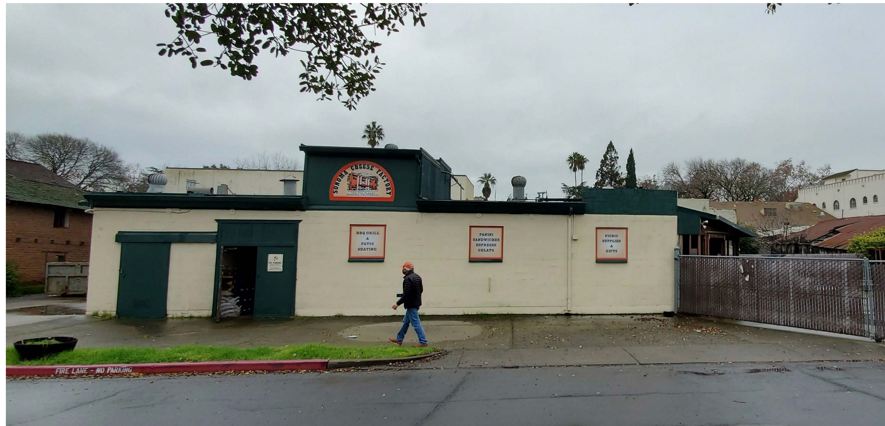
NORTH ELEVATION - FROM CASA GRANDE PARKING LOT
