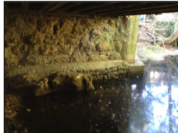
Existing Retaining Wall
