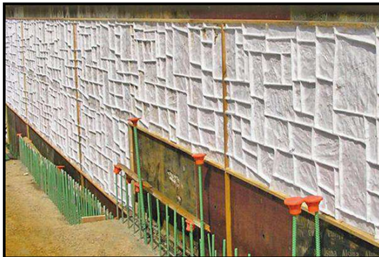
Architectural Treatment - concrete form liners
