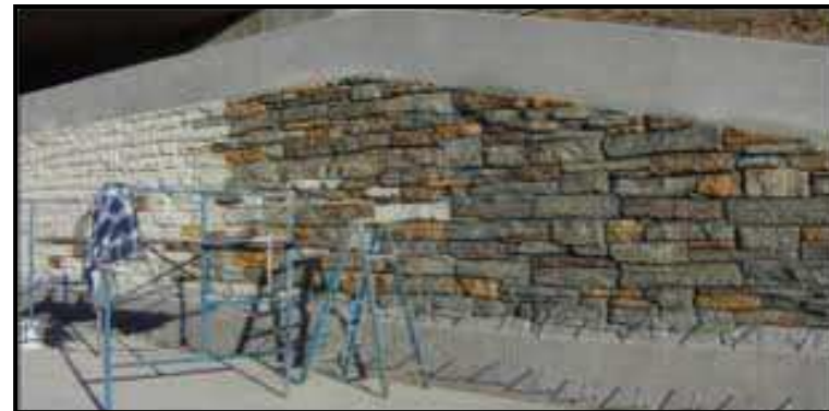
Architectural Treatment – staining concrete
