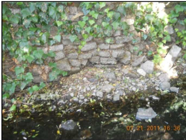
Existing Retaining Wall
