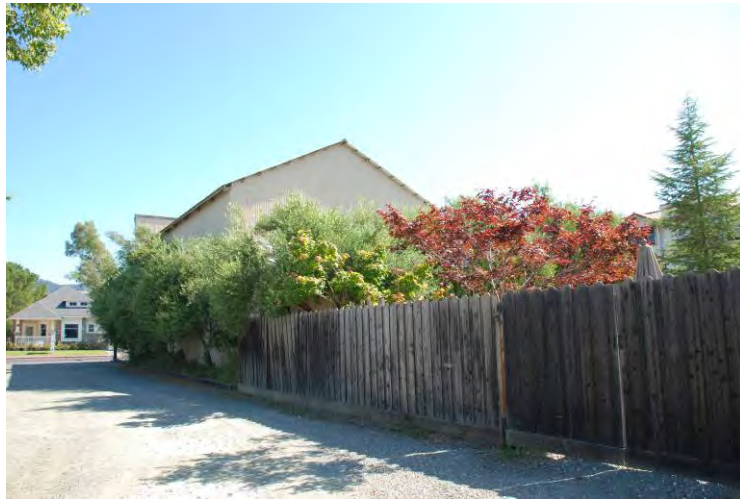
Figure 5. Looking northeast from adjacent western lot. Note the length of the subject property's rear yard. Source: Page & Turnbull.
