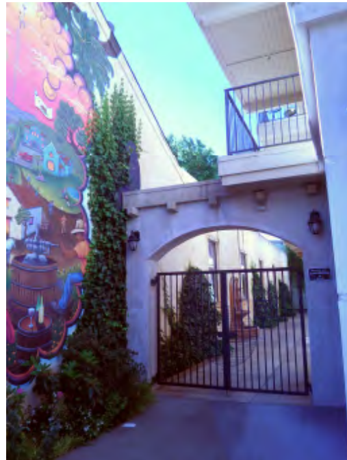
Figure 9. West façade, looking south. Source: Page & Turnbull, 2012.
