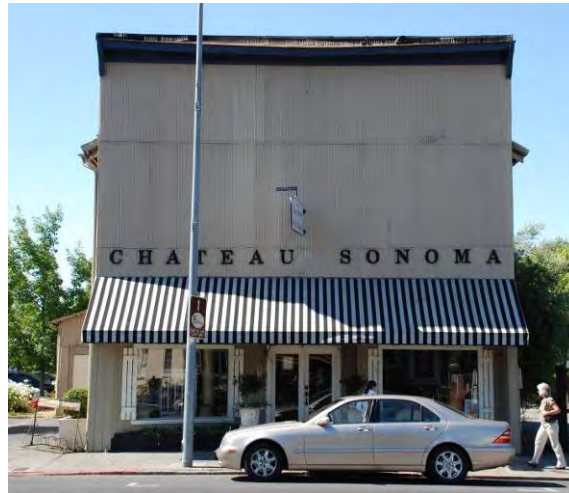
Figure 6. Primary (north) façade. Source: Page & Turnbull, 2011.
