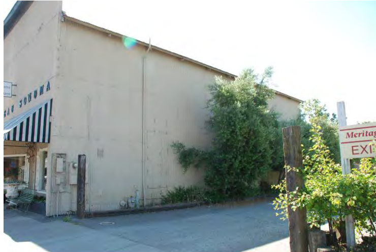
Figure 11. West façade looking southeast. Source: Page & Turnbull, 2011.
