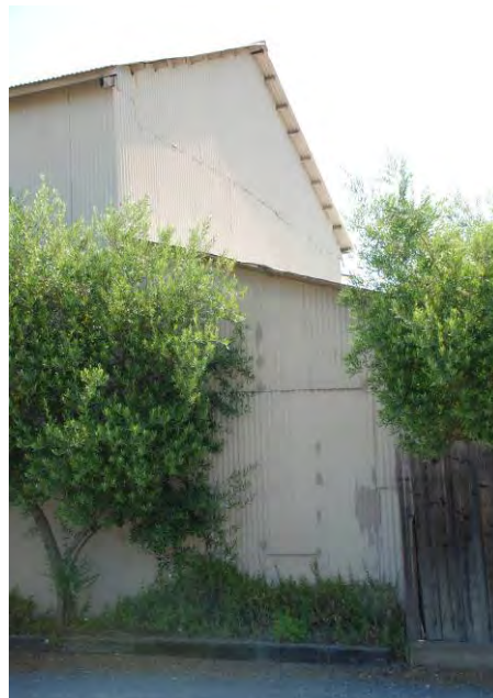
Figure 12. South façade looking northeast. Source: Page & Turnbull, 2011.
