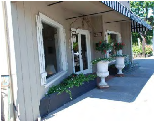
Figure 7. Recessed storefront. Source: Page & Turnbull, 2011.
