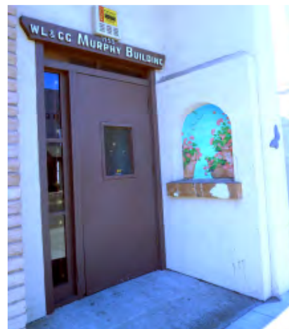
Figure 7. Doorway in west portion of primary façade. Source: Page & Turnbull, June 2012.
