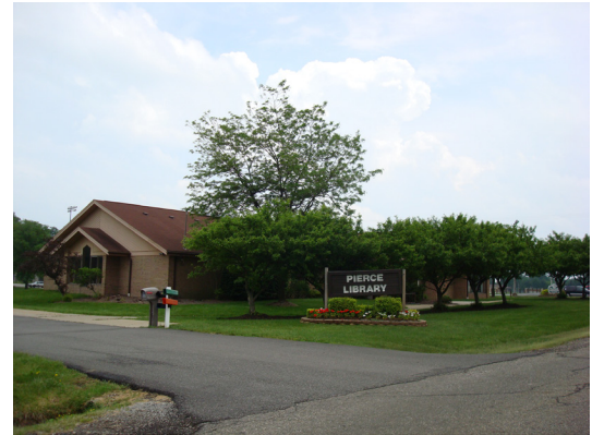
Above: Pierce Streetsboro Library on Kirby Lane.
