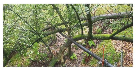
elevated pipe there is approximately 60 feet in length with two existing concrete supports for a clear span of 30'. The pipe needs to be repaired and bolstered-up with additional support like an I-beam and/or a steel casing pipe with sealed HDPE pipe.
