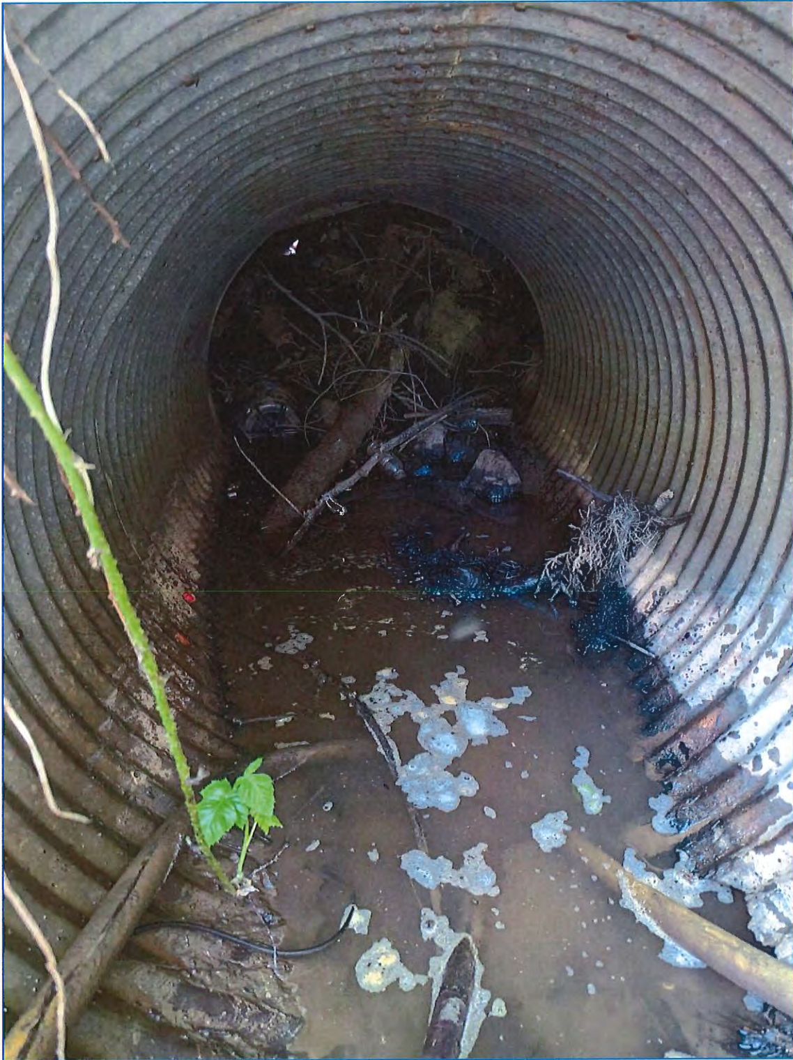
Figure 13: View looking inside the culvert under Palma Way, blocked by debris and rocks. Also the water supply hose was leaking and sitting in septic water which could pose a health risk to residents.
