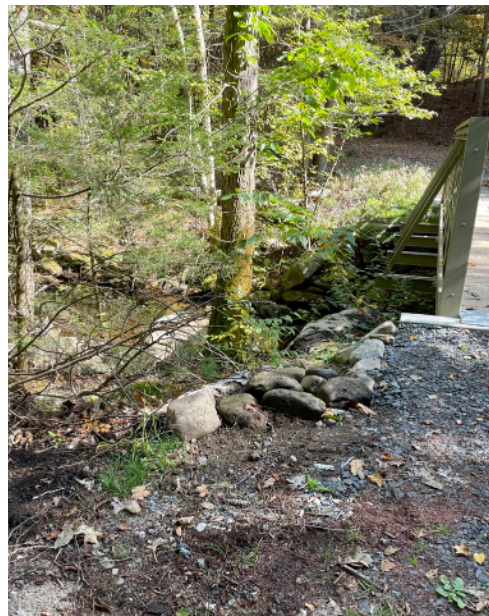
Rock reinforcement to prevent erosion. Left: larger context. Right: detail. (9.2025)
