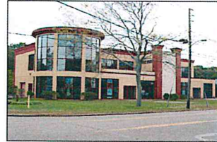
1. New building that could provide diverse business.
