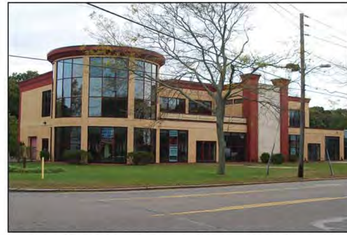
1. New building that could provide diverse business.
