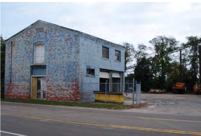
Location 5: View looking east towards Town DPW yard south of LIRR and east side of CR 31 in B-3 District
