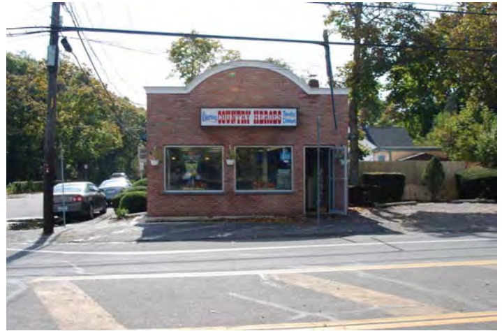
Location 34: View looking south towards restaurant on south side of CR 80 and west of CR 31 in B-2 District
