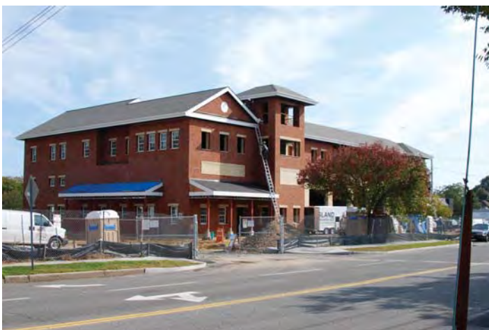
Location 42: View looking southeast toward new institutional fire station along Sunset Ave. in B-1 District
