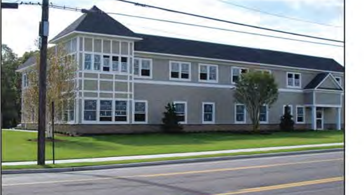
1. New building that could provide diverse business.
