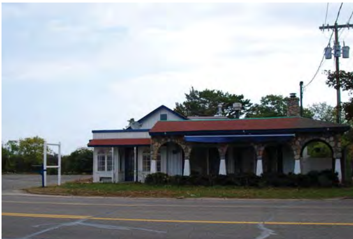
Location 3: View looking east towards abandoned commercial building north of LIRR and east side of CR 31 in B-3 District
