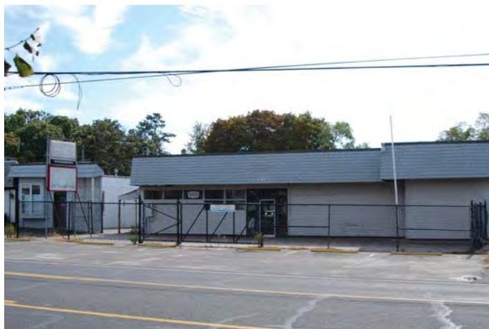
Location 31: View looking south towards vacant building along south side of CR 80 and east of CR 31 in B-2 District
