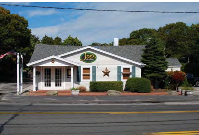
Location 36: View looking north towards restaurant north side of CR 80 and west of Beach Road in B-2 District
