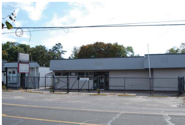
Location 31: View looking south towards vacant building along south side of CR 80 and east of CR 31 in B-2 District
