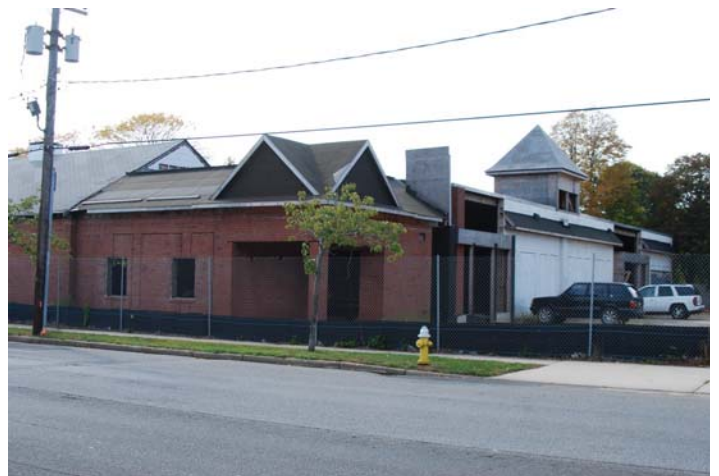
Location 43: View looking west toward vacant building along Sunset Ave. in B-1 District
