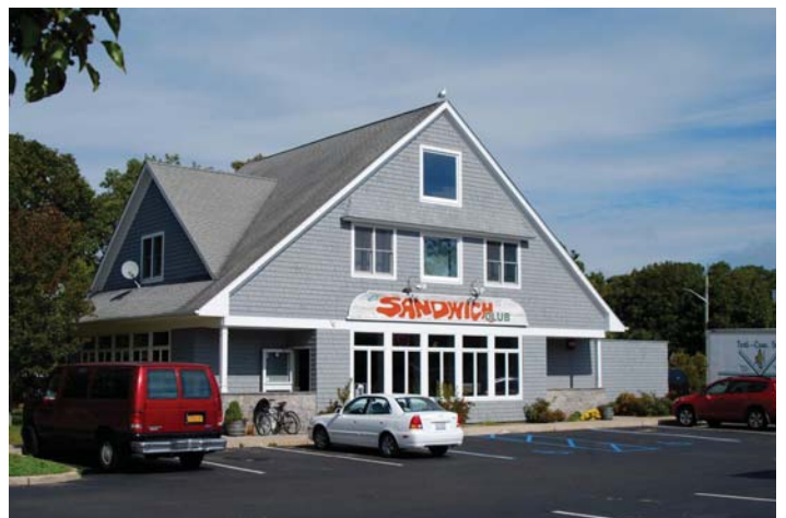
Location 29: View looking north toward a restaurant north of CR 80 along west side of Pine St. in B-2 District
