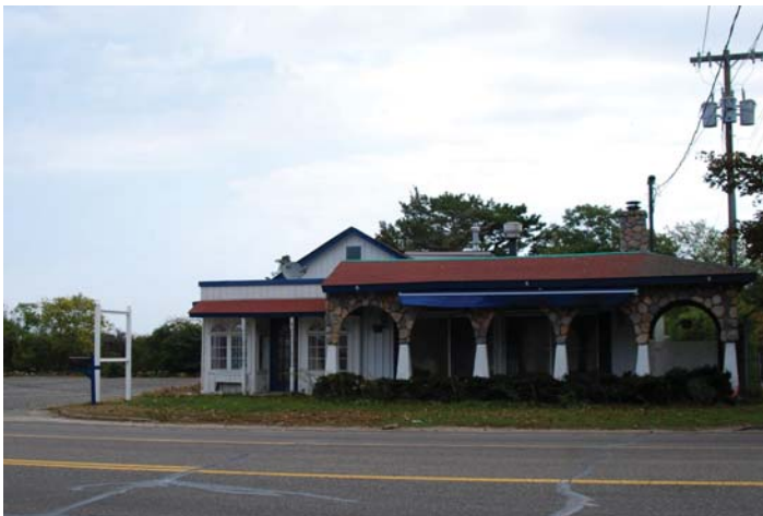
Location 3: View looking east towards abandoned commercial building north of LIRR and east side of CR 31 in B-3 District
