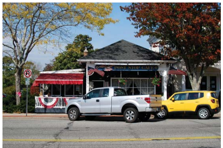
Location 24: View looking north toward mixed use retail and restaurant along Main St. in B-1 District
