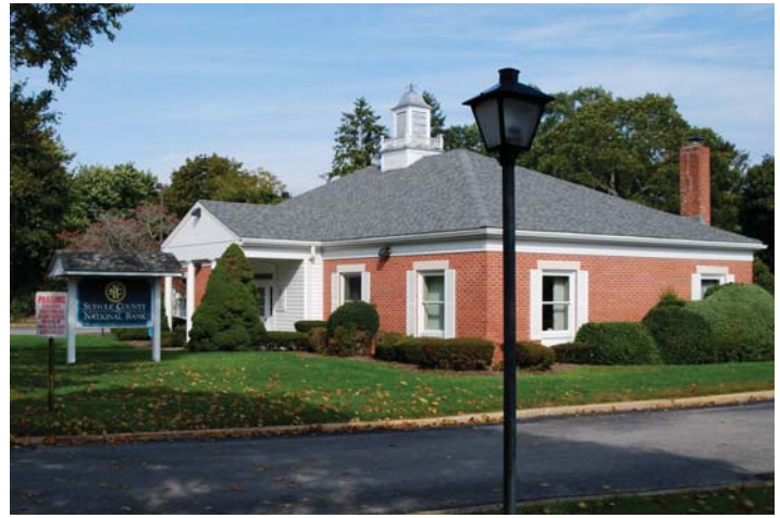
Location 45: View looking north toward a bank along Mill Rd. in B-1 District
