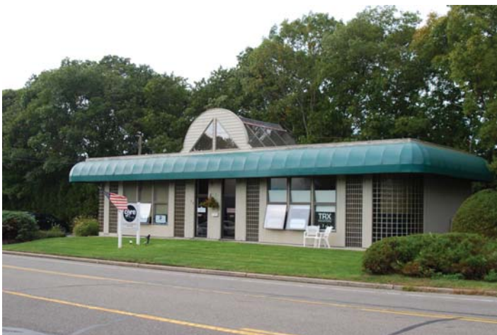
Location 11: View looking west towards medical office building on west side of CR 31 in B-2 District
