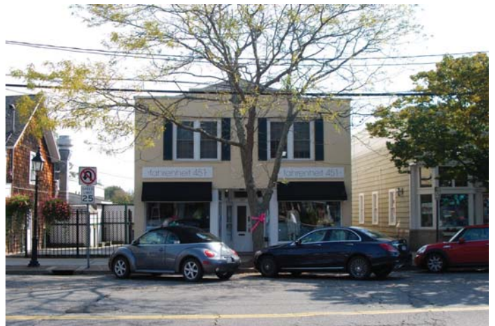
Location 18: View looking south towards retail business along Main St. in B-1 District
