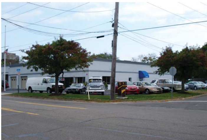
Location 7: View looking northeast towards motor vehicle services property south of LIRR, north of Rogers Ave. and east side of CR 31 in B-3 District
