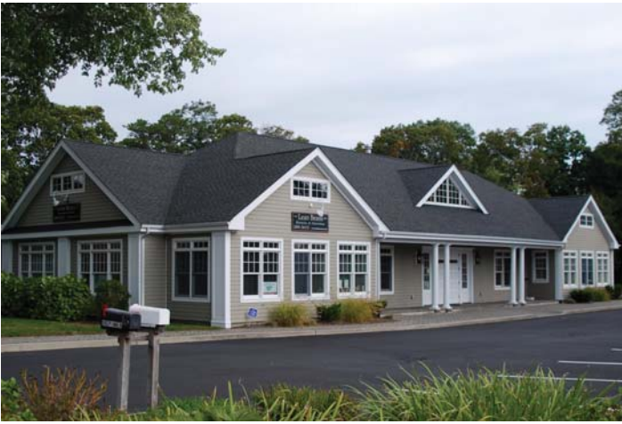
Location 13: View looking east towards office and medical office on east side of CR 31 in B-2 District
